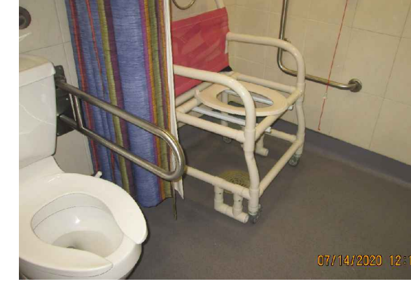
PIC. 4 EX. SHOWER AREA
