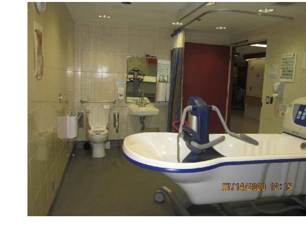
PIC. 1 EX. TUB & TOILET
