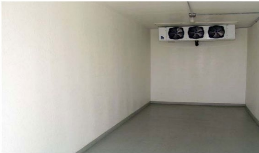
20x8 Cooler Electrical Requirements: 30 amps, 208-230 Volt, single phase
