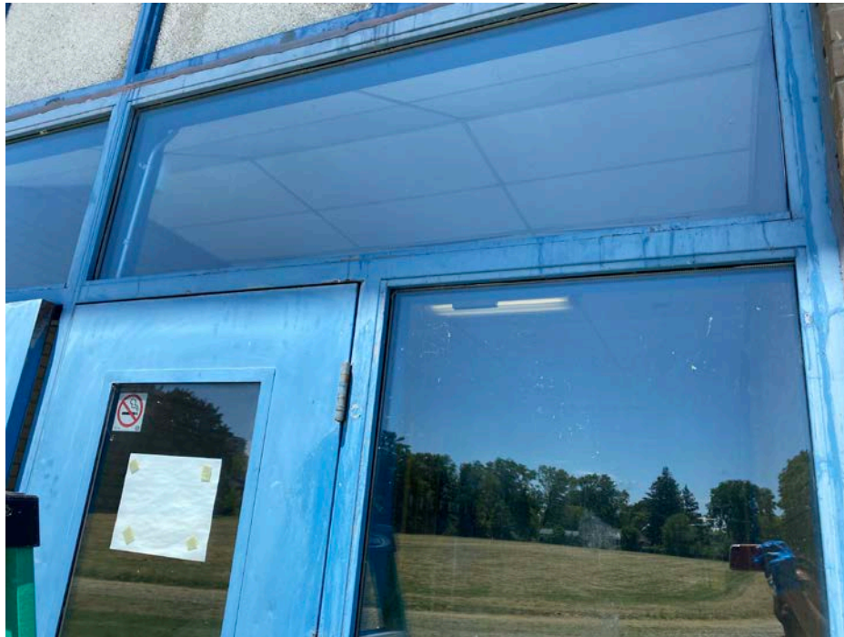
Photograph 3: View of the lead-containing blue paint on the door of Entrance 11 at the Subject Location.
