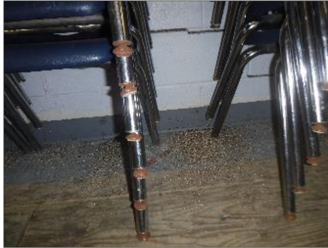
Photo 3 - . Non-asbestos vermiculite in the Hallway around the Ice Rink (Location 1-25).
