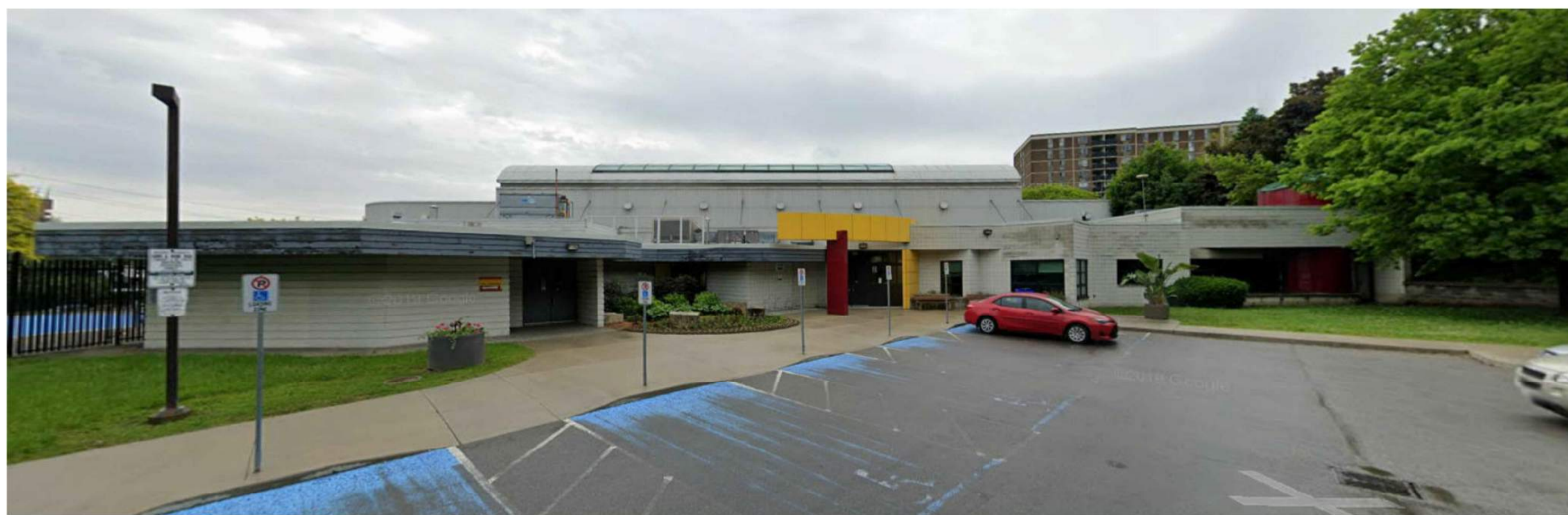
EAST ELEVATION - FRONT OF BUILDING EXTERIOR REPAIRS
