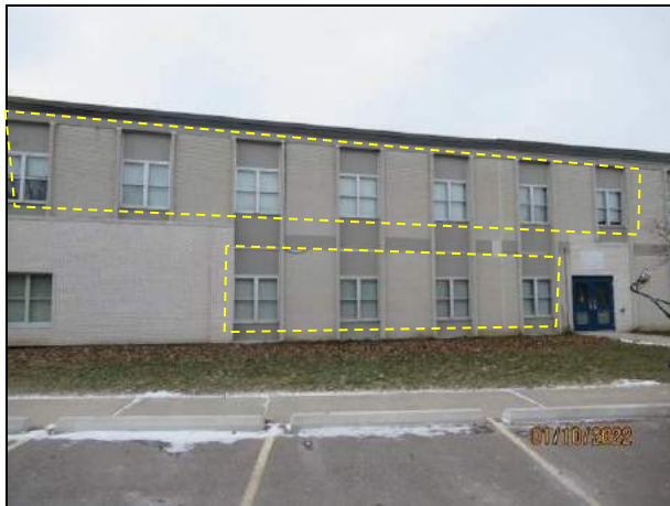
Photograph 5: Typical W5 windows (50 total) to be replaced.
