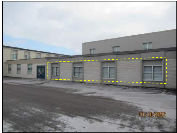
Photograph 6: Typical W6 windows (10 total) to be replaced.
