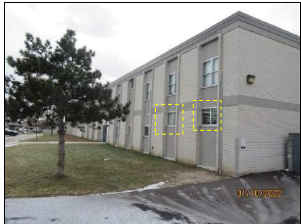
Photograph 8: Typical W8 windows (4 total) to be replaced.
