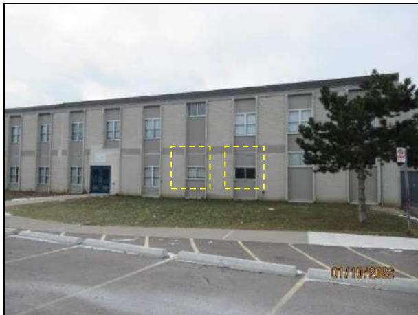
Photograph 7: Typical W7 windows (3 total) to be replaced.
