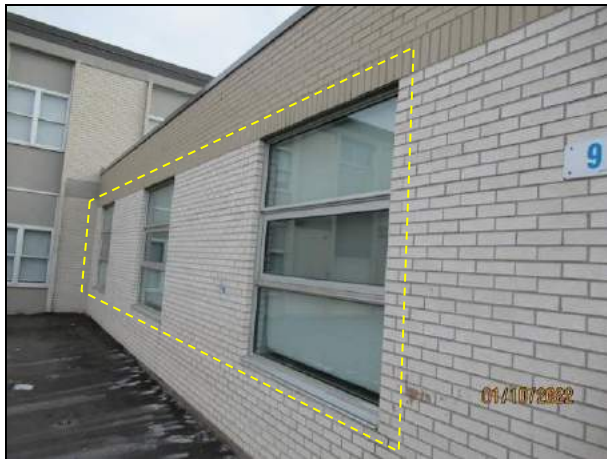
Photograph 3: Typical W3 windows (3 total) to be replaced.
