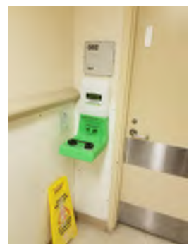
EXISTING CONDITION PHOTO - ECP16
