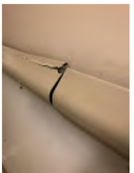
EXISTING CONDITION PHOTO - ECP17
