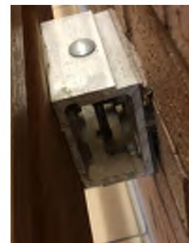
EXISTING CONDITION PHOTO - ECP09
