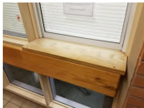
EXISTING CONDITION PHOTO - ECP06
