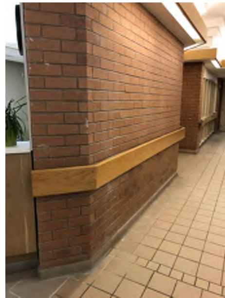
EXISTING CONDITION PHOTO - ECP01
