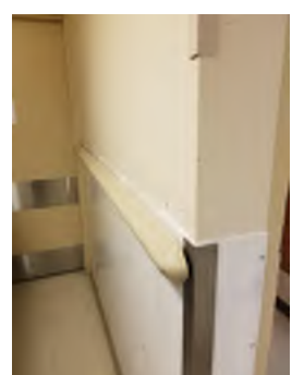
EXISTING CONDITION PHOTO - ECP19
