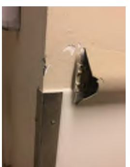
EXISTING CONDITION PHOTO - ECP20
