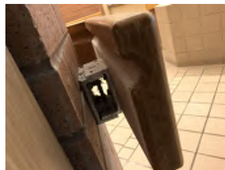
EXISTING CONDITION PHOTO - ECP07
