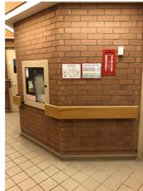
EXISTING CONDITION PHOTO - ECP04
