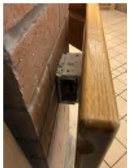
EXISTING CONDITION PHOTO - ECP11
