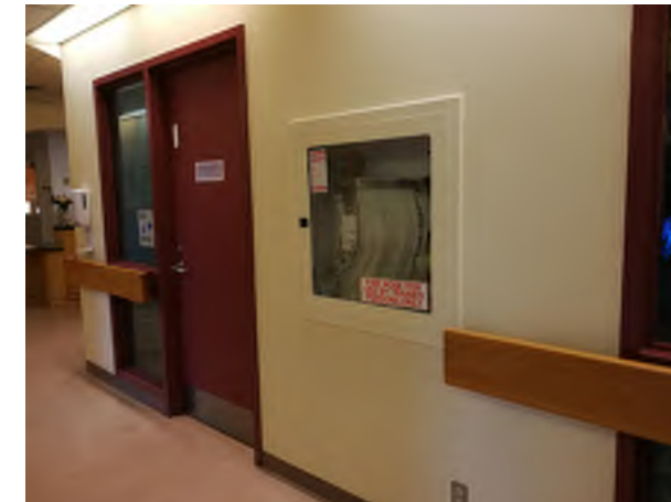
EXISTING CONDITION PHOTO - ECP13
