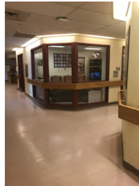
EXISTING CONDITION PHOTO - ECP03
