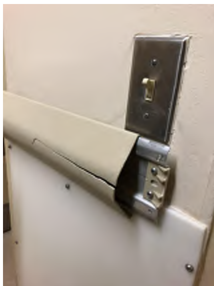
EXISTING CONDITION PHOTO - ECP15
