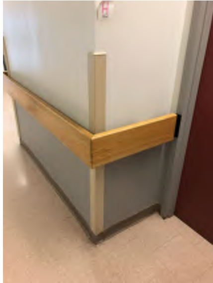
EXISTING CONDITION PHOTO - ECP05
