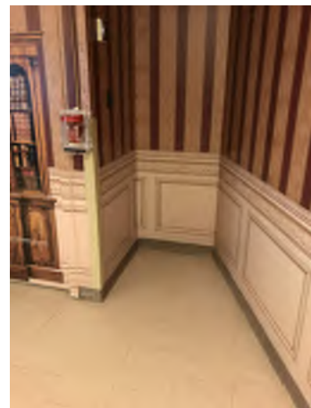
EXISTING CONDITION PHOTO - ECP04
