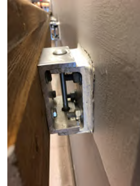
EXISTING CONDITION PHOTO - ECP09
