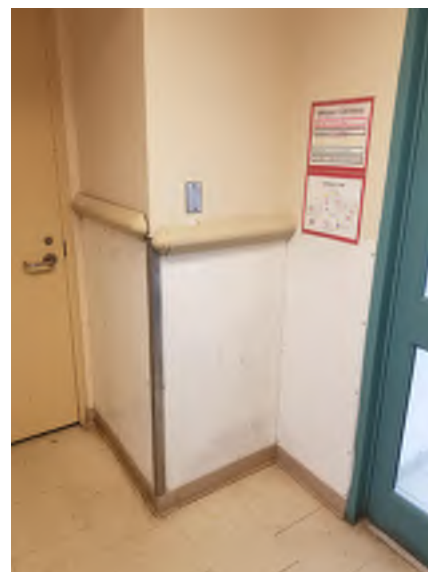
EXISTING CONDITION PHOTO - ECP14
