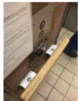
EXISTING CONDITION PHOTO - ECP10
