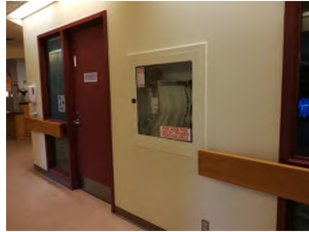
EXISTING CONDITION PHOTO - ECP03
