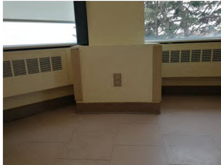
EXISTING CONDITION PHOTO - ECP01
