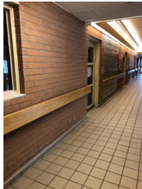
EXISTING CONDITION PHOTO - ECP03
