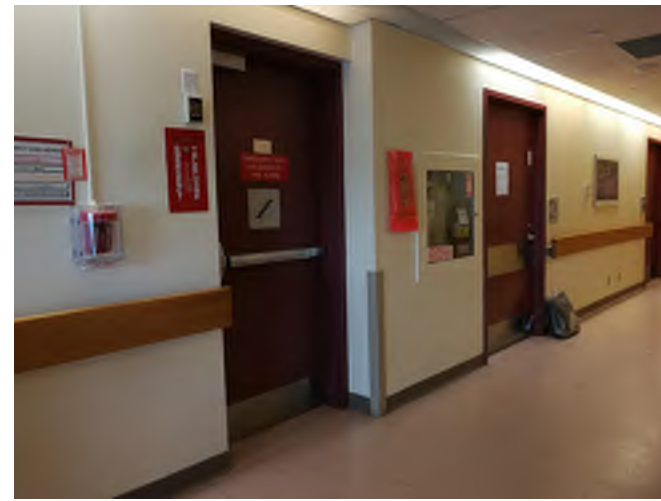
EXISTING CONDITION PHOTO - ECP02
