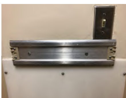
EXISTING CONDITION PHOTO - ECP21
