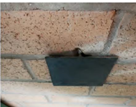
EXISTING CONDITION PHOTO - ECP12
