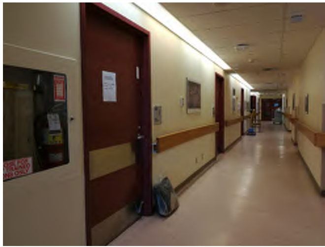
EXISTING CONDITION PHOTO - ECP01
