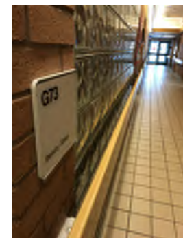
EXISTING CONDITION PHOTO - ECP08
