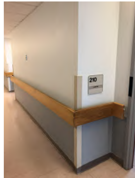
EXISTING CONDITION PHOTO - ECP 02
