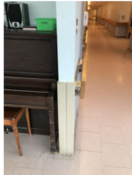
EXISTING CONDITION PHOTO - ECP11
