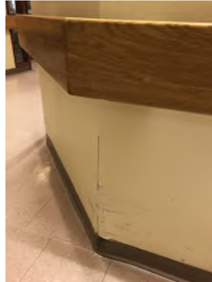
EXISTING CONDITION PHOTO - ECP07
