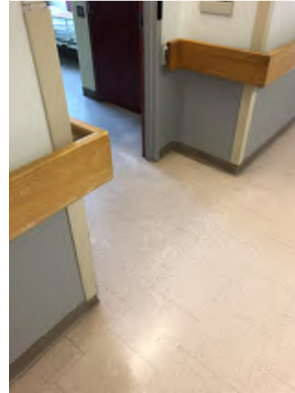
EXISTING CONDITION PHOTO - ECP06
