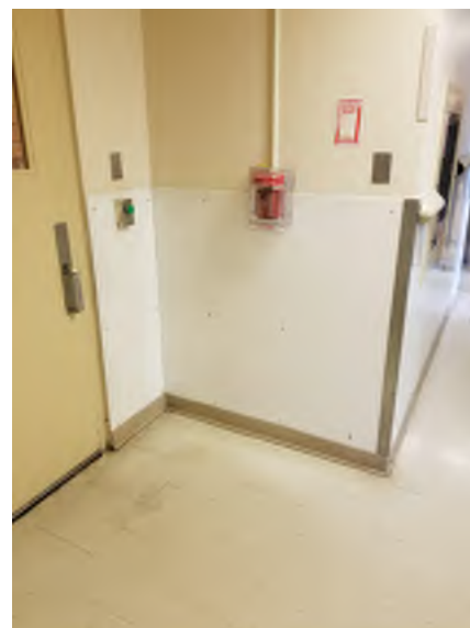
EXISTING CONDITION PHOTO - ECP13
