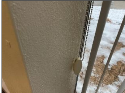
Non-asbestos plaster on columns throughout the assessed area
