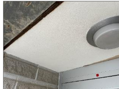
Non asbestos plaster on exterior soffits
