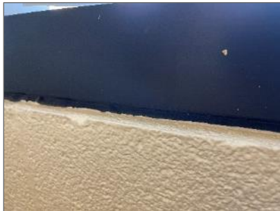
Non-asbestos window frame caulking
