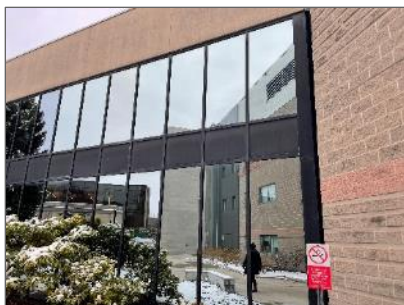
Non-asbestos butyl sealant on exterior window frames
