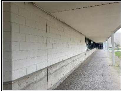
Non asbestos textured finish on exterior drywall soffits
