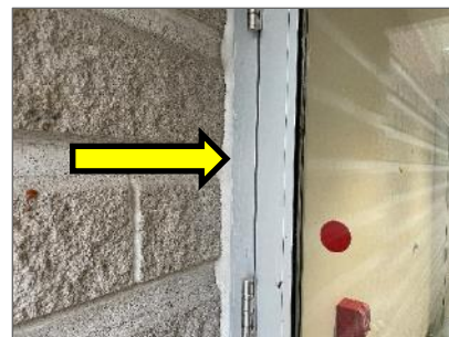
Non-asbestos grey caulking on exterior door frame
