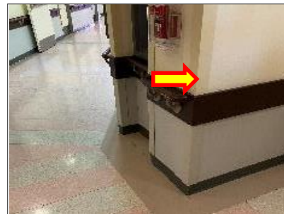
Insignificant level light yellow paint on drywall present throughout the floor.
