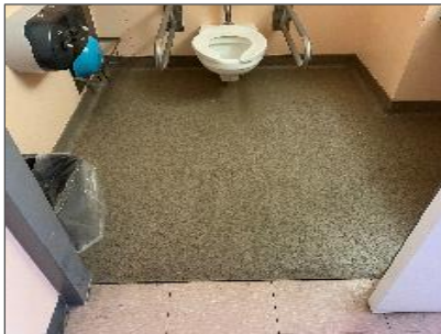
Non-asbestos, VSF2, beige with black flecks (Loc. 3-074).
