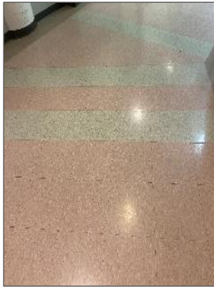
Non-asbestos VFT2 present throughout the corridors in northern portion of 3 rd floor.
