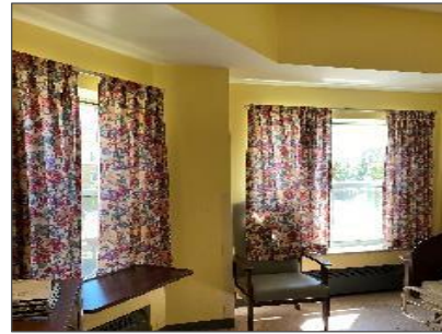
Insignificant level lead yellow paint on drywall wall, Loc. 3-019.
