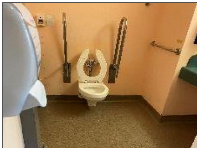
Insignificant level lead light pink paint on drywall present throughout the floor.
