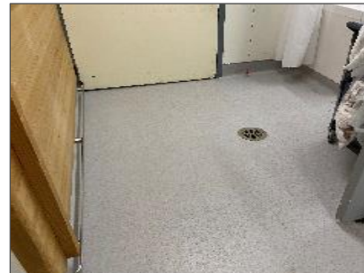
Non-asbestos, VSF11, light grey with black flecks (Loc. 3-081).
