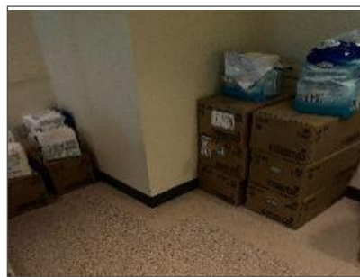
Insignificant level white paint on drywall present throughout the floor.
