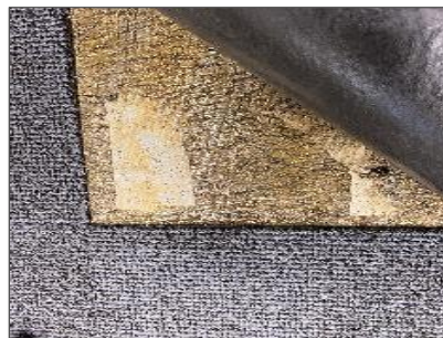
Non-asbestos yellow carpet mastic, office (Loc. 3-038).
