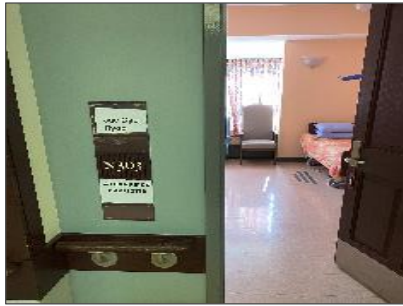
Insignificant level lead light blue paint on drywall wall, Loc.3-036.
