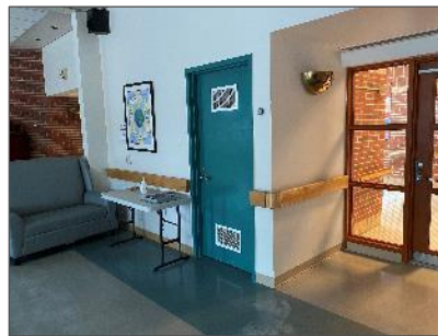
Non-asbestos joint compound on drywall walls, Auditorium (Loc. 1-089).
