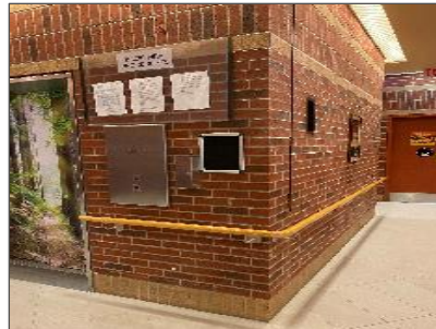
Non-asbestos mortar on brick walls, corridor (Loc. 1-097).
