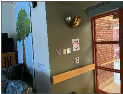
Insignificant level of lead in olive green paint on drywall, Auditorium (loc. 1-092).
