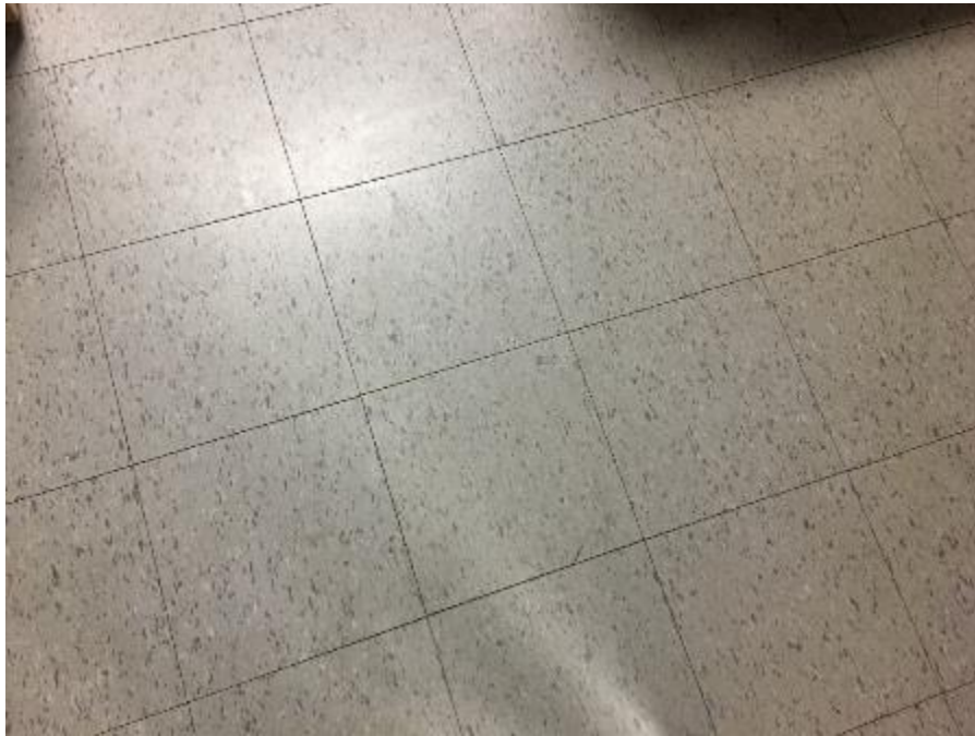
Photo 7: 12" x 12" Vinyl Floor Tile, grey with brown and white flecks confirmed to not contain asbestos, sampled in Room 126, 224 and 324 (Maple Sample ID 12233-S-02a-c).
