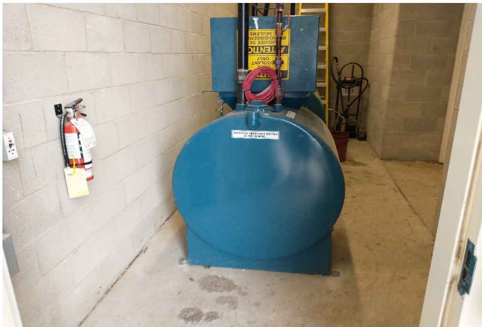
Photograph 2: View of an aboveground storage tank containing oil observed on the Waste Oil Room at the Subject Location.
