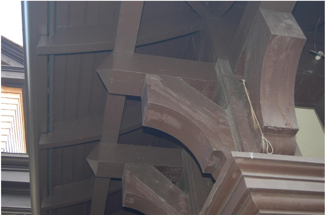
Photo 4: whitish areas may be lead sulphate as found on doors; needs to be analysed.
