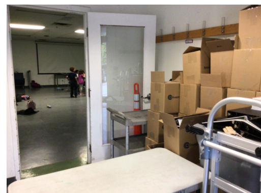
PHOTO 2: REMOVE EXISTING DOOR AND FRAME AND WIDEN OPENING.
