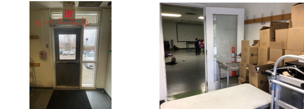
PHOTO 2: REMOVE EXISTING DOOR AND FRAME AND WIDEN OPENING.
