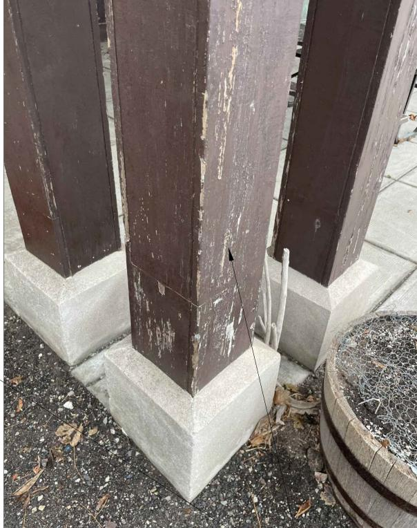
CONSOLIDATE/FILL AND REPAINT OUTER WOOD PANELS
