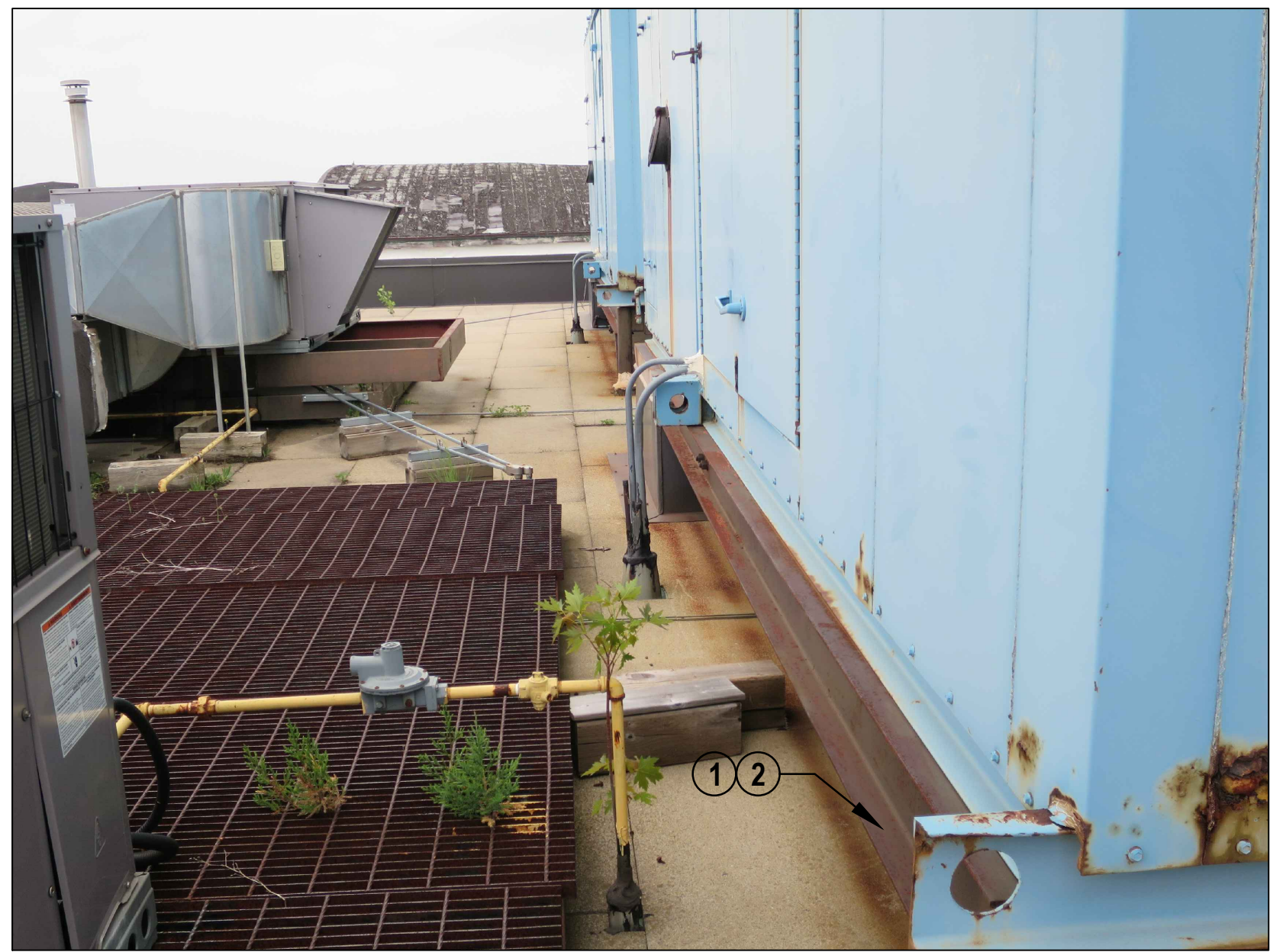
EXISTING ROOF CURB SUPPORT
