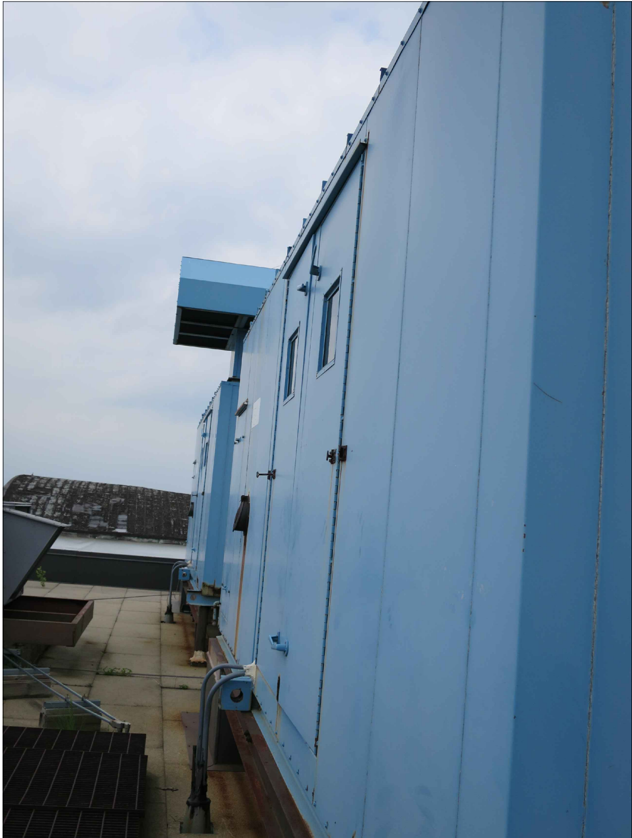
EXISTING ELECTRICAL ROOF PENETRATION
