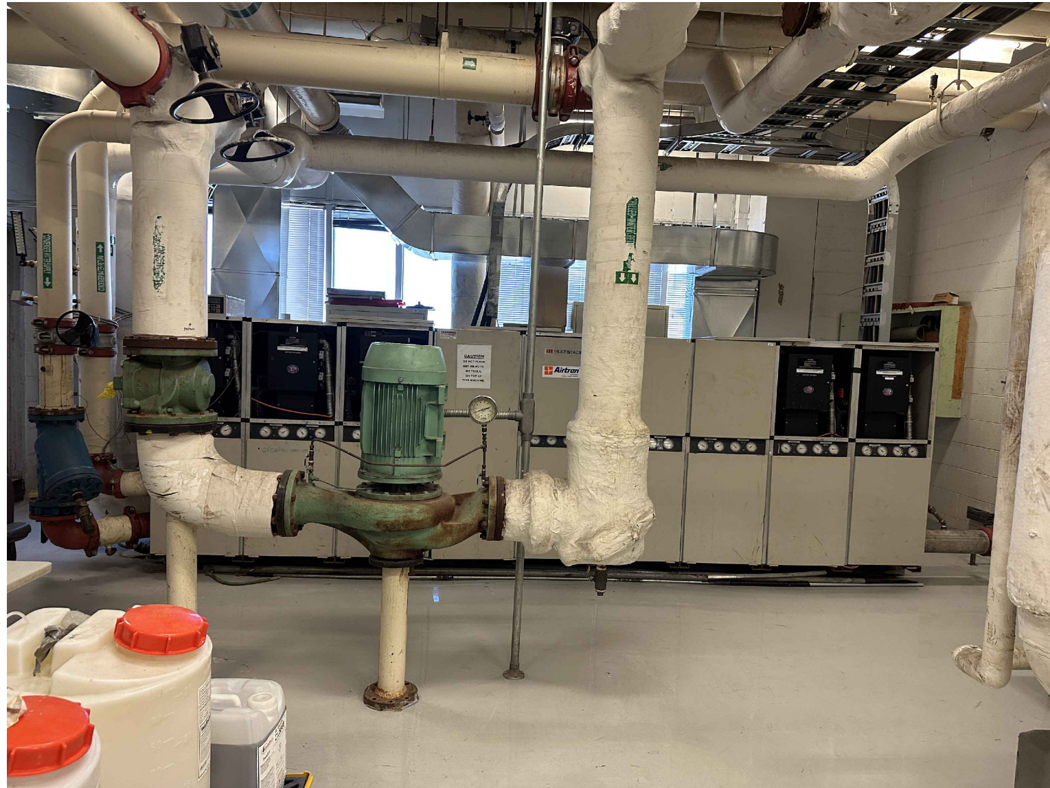
EXISTING MULTI-STACK CHILLER SETUP.
