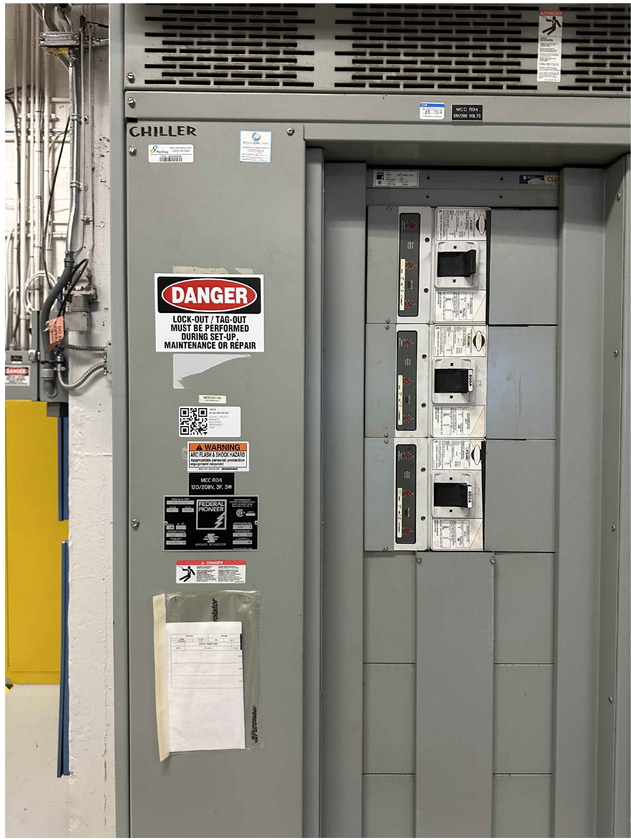
EXISTING ELECTRICAL MCC PANEL, MCC.
