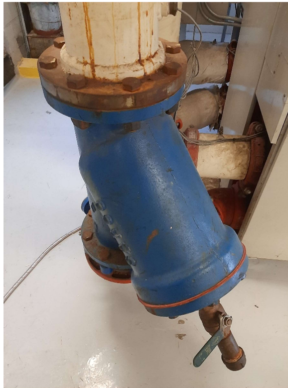
Photograph No. 4 – The blue paint on valves was observed in the penthouse mechanical room was sampled (LP02) and was reported as low level lead-containing.
