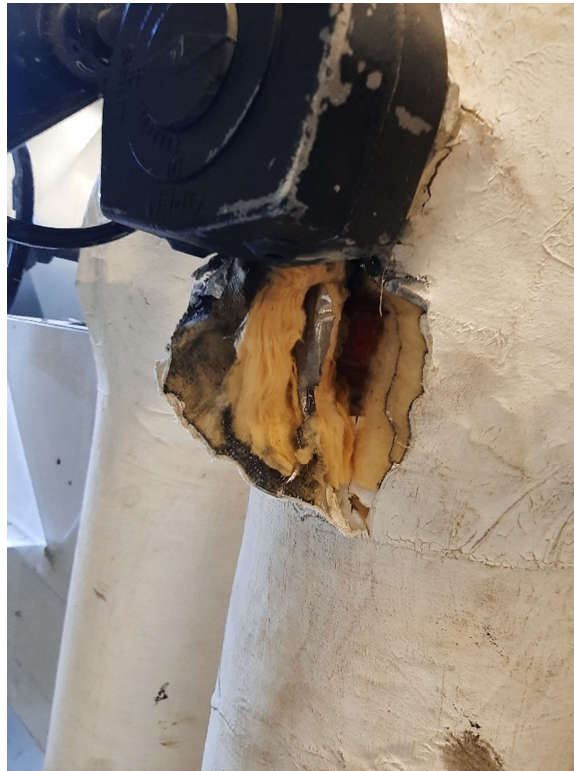
Photograph No. 1 – Fibreglass insulation was observed on pipe straights and elbows within the Penthouse Mechanical room.
