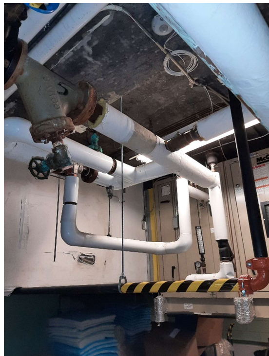
Photograph No. 8– The pipe network associated with the basement air handling unit in the basement mechanical room is a combination of fiberglass and PVC over fiberglass; therefore no suspect asbestos material is suspected present. The insulation on the ducts is also fiberglass.
