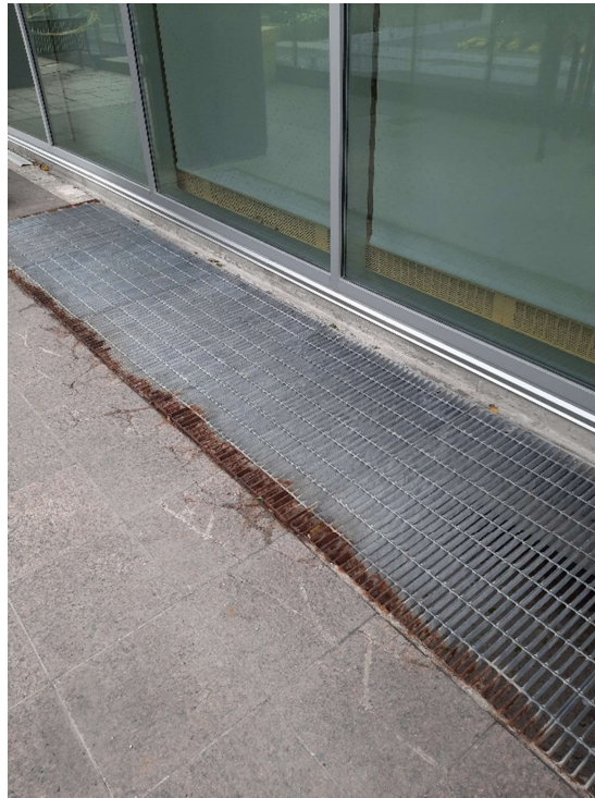
Photograph No. 10 – The exterior intake grating was inspected, and no suspect asbestos-containing material were observed; however, the masonry adjacent to the intake contains silica.
