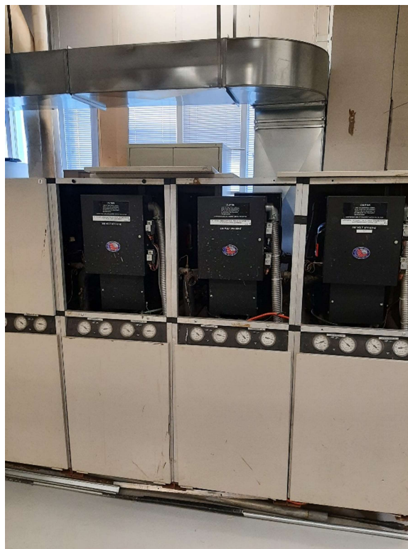
Photograph No. 2 – Ozone Depleting Substances are assumed within the chiller system.
