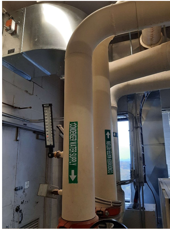
Photograph No. 3 – The white paint on pipe straights in the penthouse mechanical room was sampled (LP01) and was reported as low level lead-containing.
