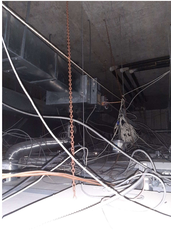
Photograph No. 5 – The variable air volume boxes were observed above ceiling spaces on the 15 th floor. No suspect asbestos material associated with the equipment was observed at the time of inspection.
