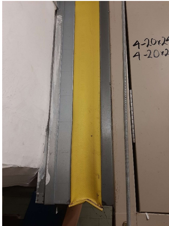
Photograph No. 9 – Rubber expansion joints were observed on the air handling unit which connects to the intake ducts. No asbestos is suspected present.
