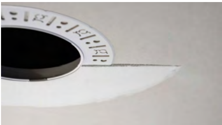
Partially finished mud ring, showing cross-section detail.
