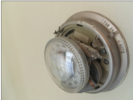
Liquid mercury in thermostats within the 2 nd Floor
