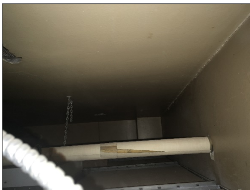
Non-asbestos plaster ceiling within the Men's Washroom, Location 8
