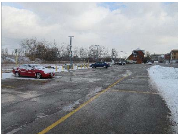
View of the asphalt paved parking areas on the west portion of the Site.
