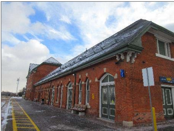
General view of the north elevation of the Site Building.
