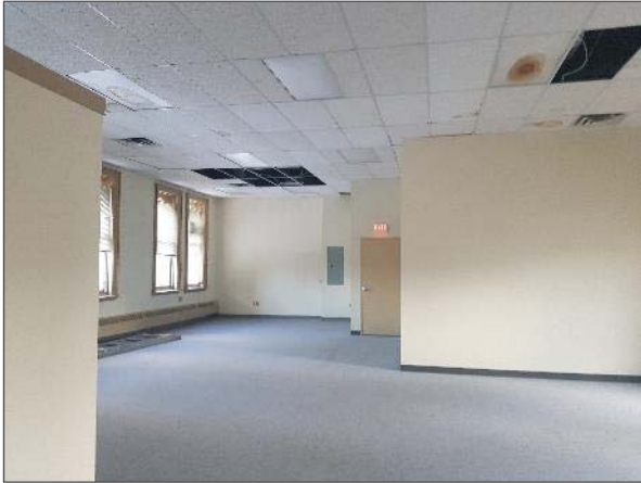
View of the finishes within the vacant second floor area.
