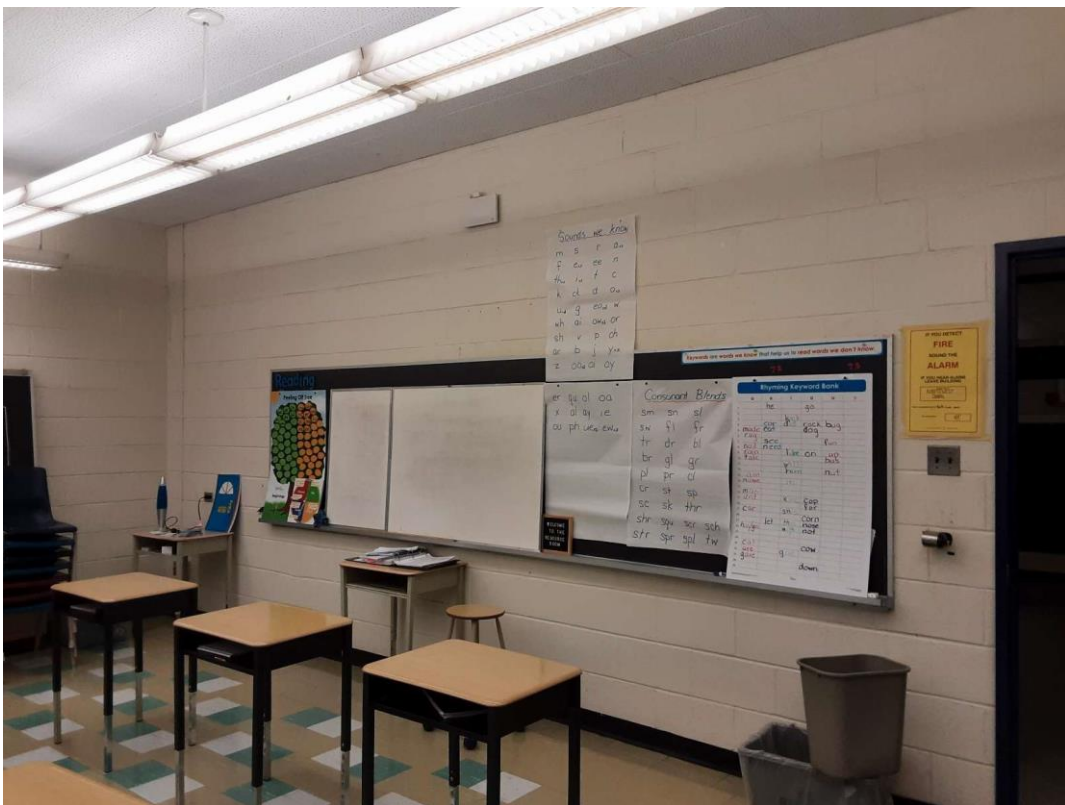
S0159C (Confirmed Asbestos), White paint on block wall in Location #: 262
