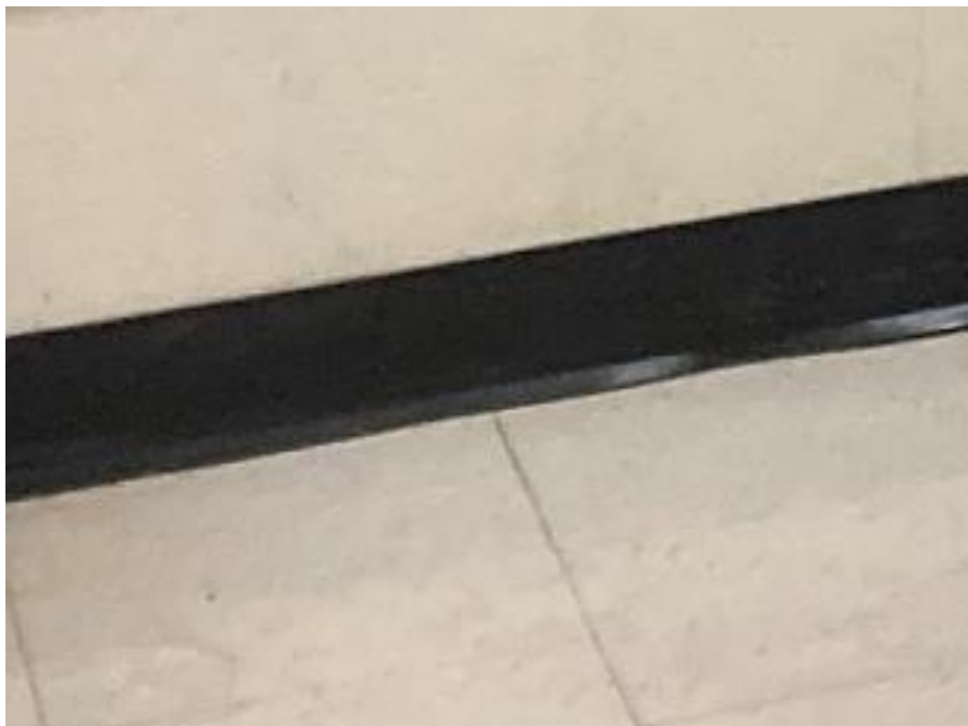
S0170 (Confirmed Asbestos), mastic behind the baseboard in Location #: 260
