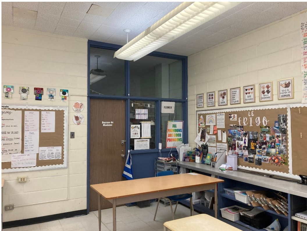
L0039 (Lead Containing), Blue paint on various metal pieces in Location #: 259
