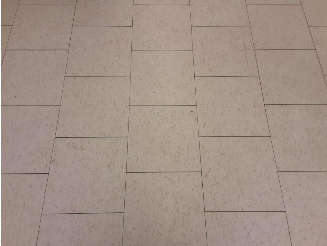
S0163C (None), 12in by 12in white mottled vinyl Floor Tile and Mastic in Location #: 259
