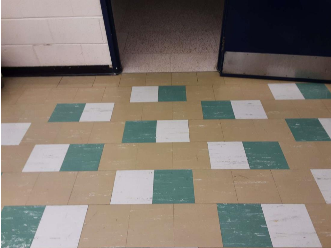
S0168C (Confirmed Asbestos), 9in by 9in light green Vinyl Floor Tile and Mastic in Location #: 262
