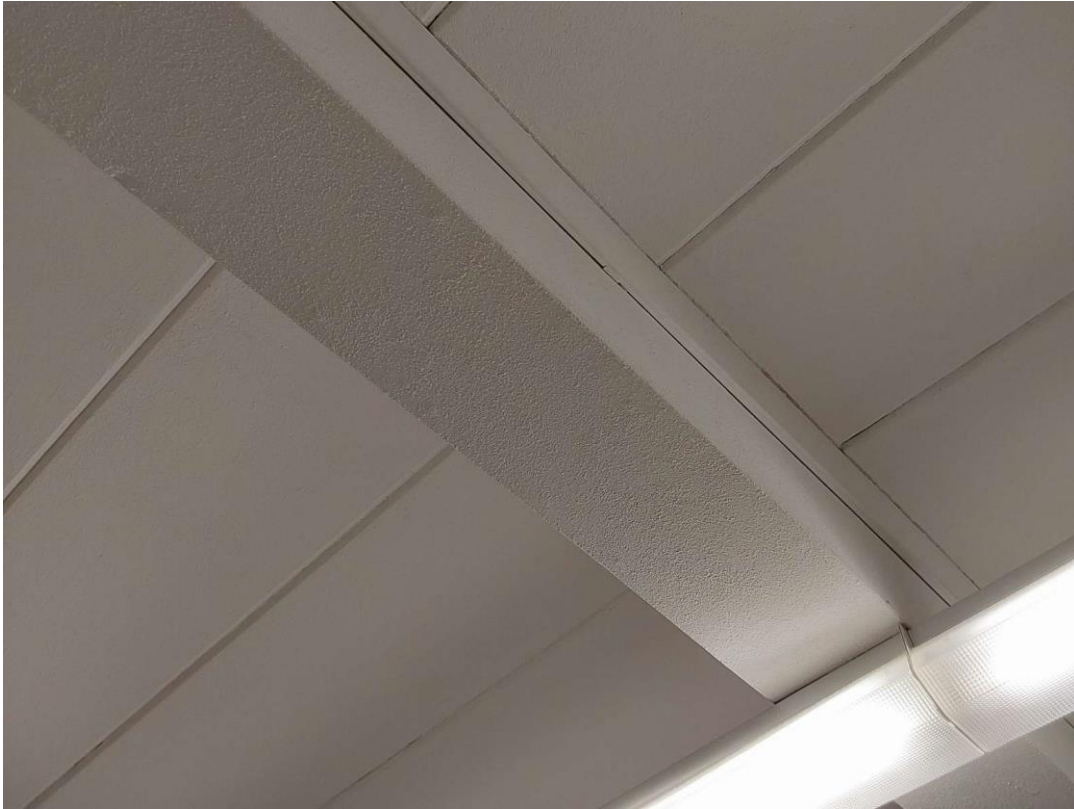
S0019A (Confirmed Asbestos), Structure, Texture Coat, CLASSROOM (Location #: 13)
