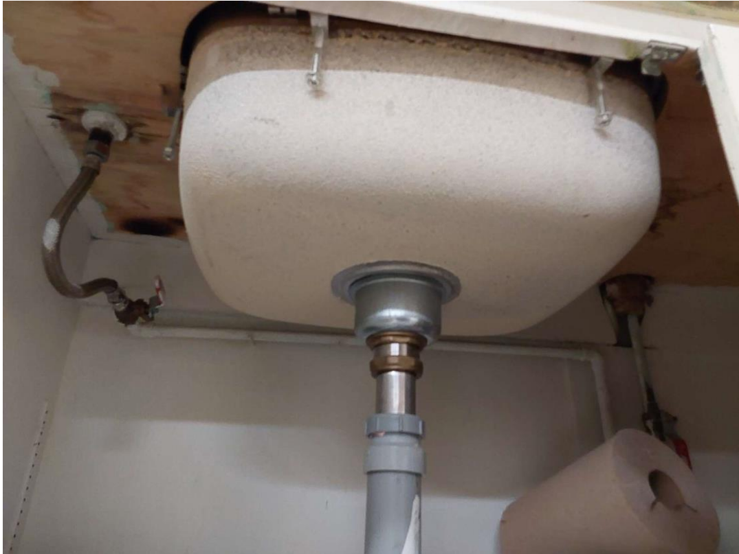
S0027C (None), Other, Adhesive/mastic, CLASSROOM (Location #: 26) Grey sink mastic
