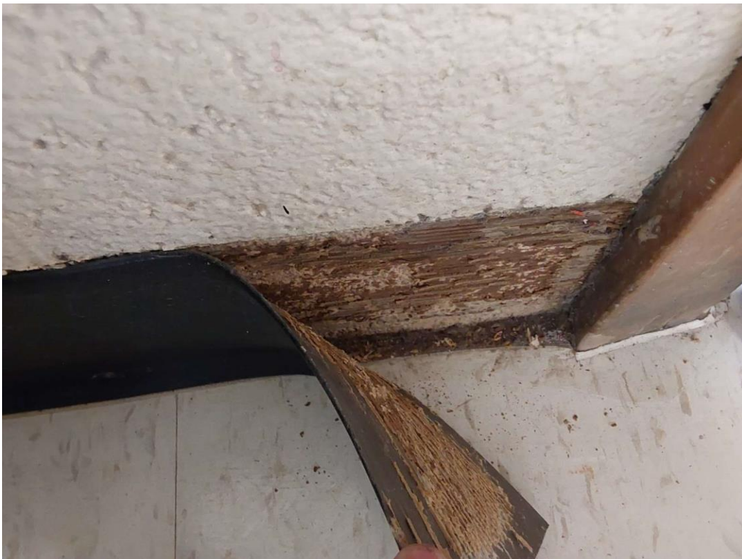
S0020A (None), Mastic behind vinyl baseboards, Wall, Adhesive/mastic, CLASSROOM (Location #: 13)
