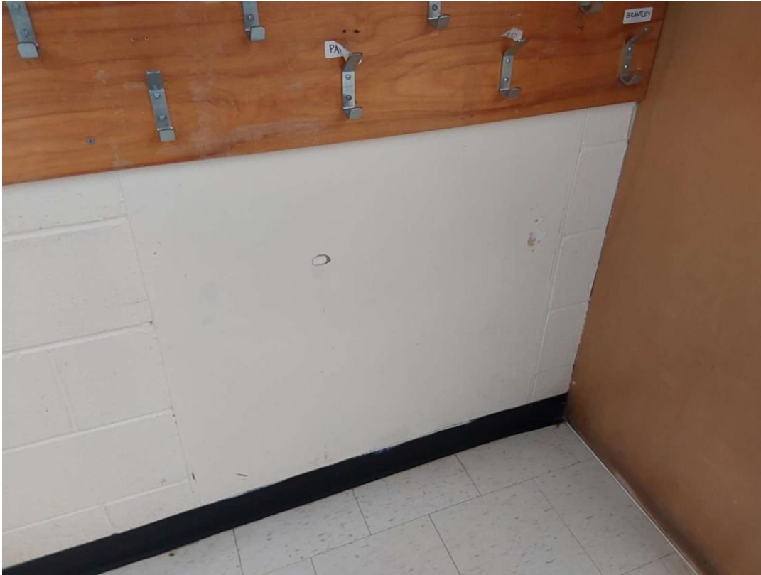
V0001 (None), Wall, Drywall and joint compound, CLASSROOM (Location #: 26)
