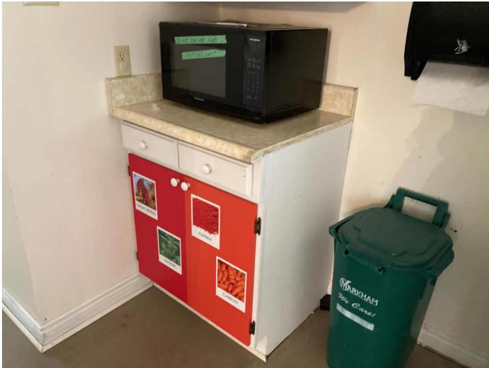
8. Existing kitchen countertop to be replaced
