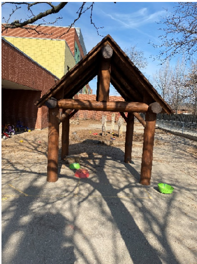
Existing Wooden Structure To be removed and disposed off-site
