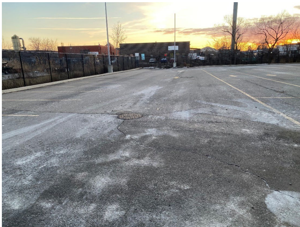
Photograph 3 Southern Area of the Site Looking West (cracks focused on sewers)
