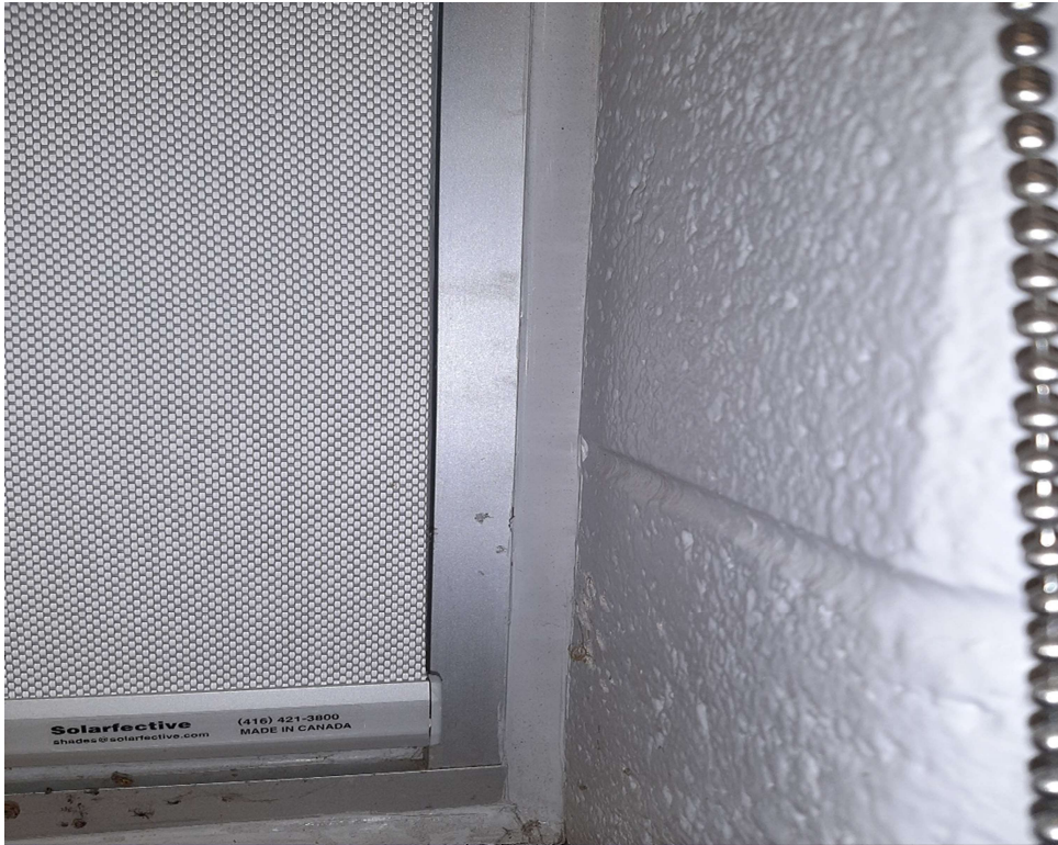
Photograph No. 3 – Gray interior window sealant in 2044 and 2041 is non-asbestos.
