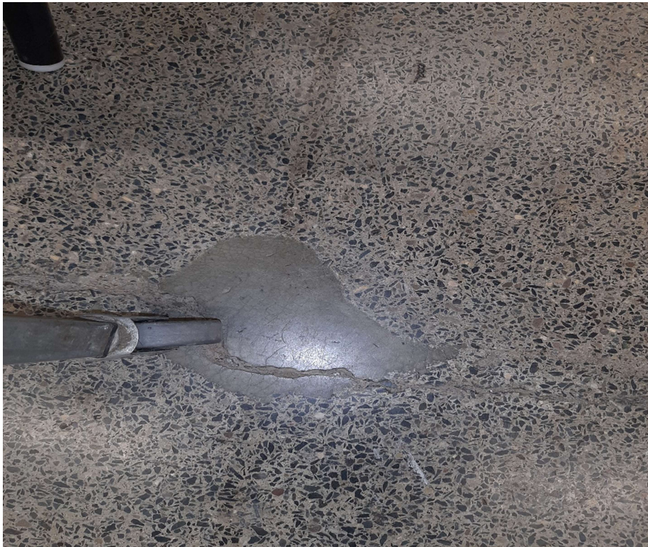
Photograph No. 4 – Floor levelling compound in 2044 is non-asbestos.
