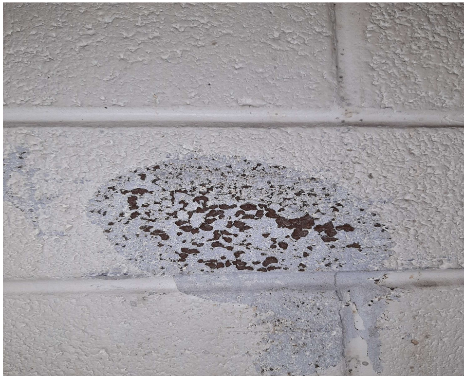
Photograph No. 6 – Brown wall mastic residue in 2041 was found to be non-asbestos.
