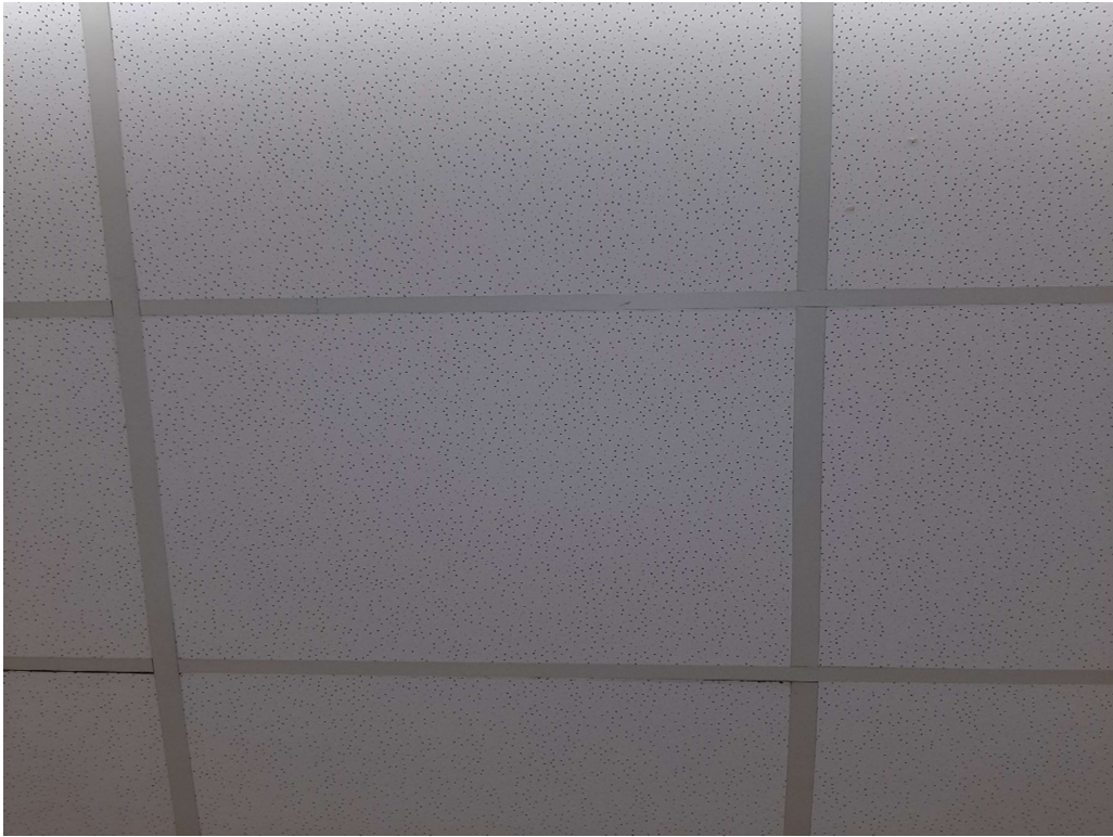
Photograph No. 1 – 2’x4’ pinhole pattern ceiling tiles are non-asbestos.
