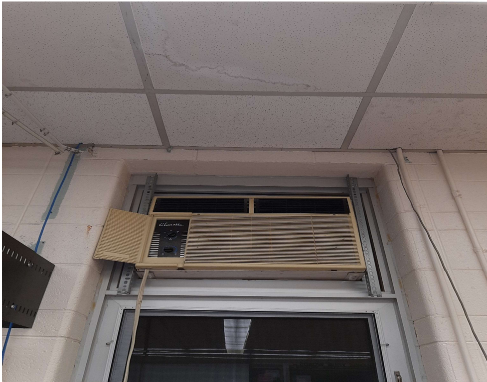
Photograph No. 8 – Window mounted air-conditioners may contain ODSs.
