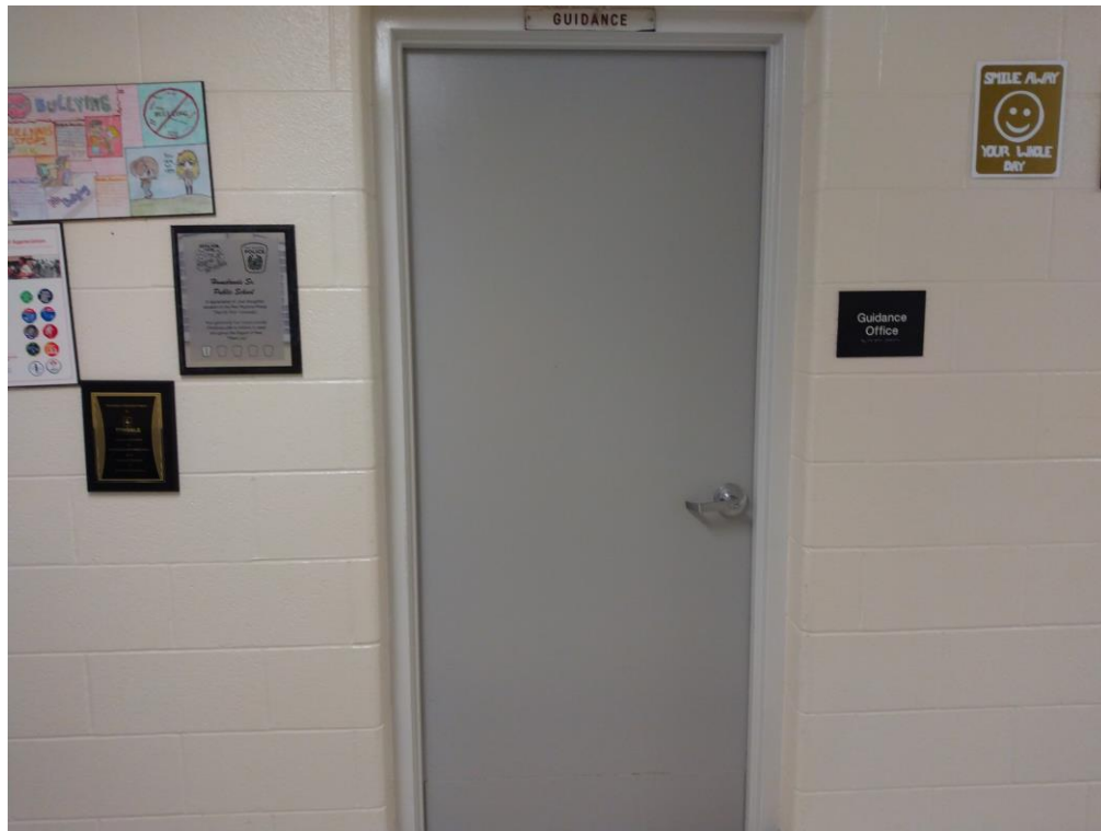
Photograph 1: Existing elevation for single door slab replacement for door No. 12.
