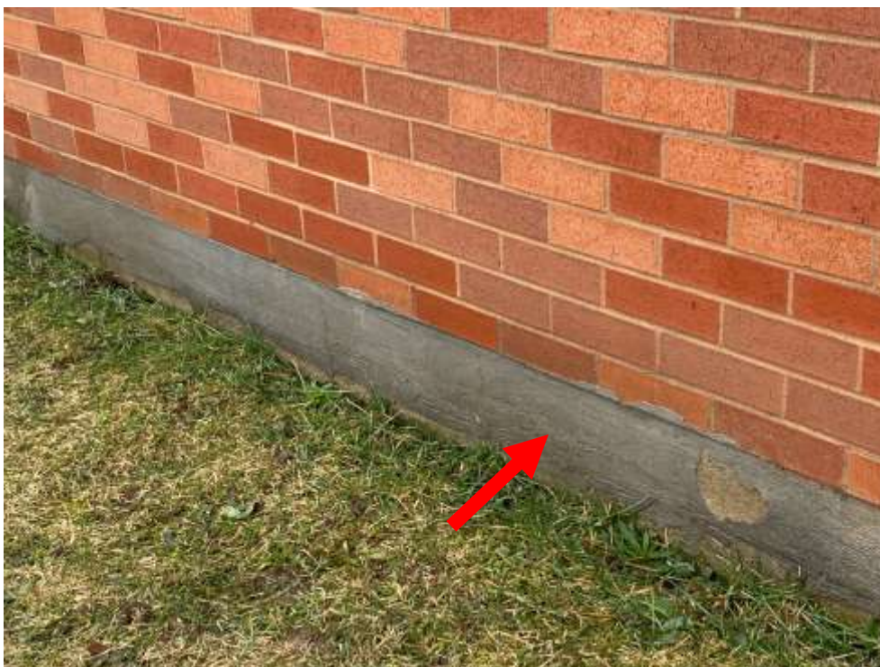
Photo 6 – View of non-asbestos-containing cement parging.
