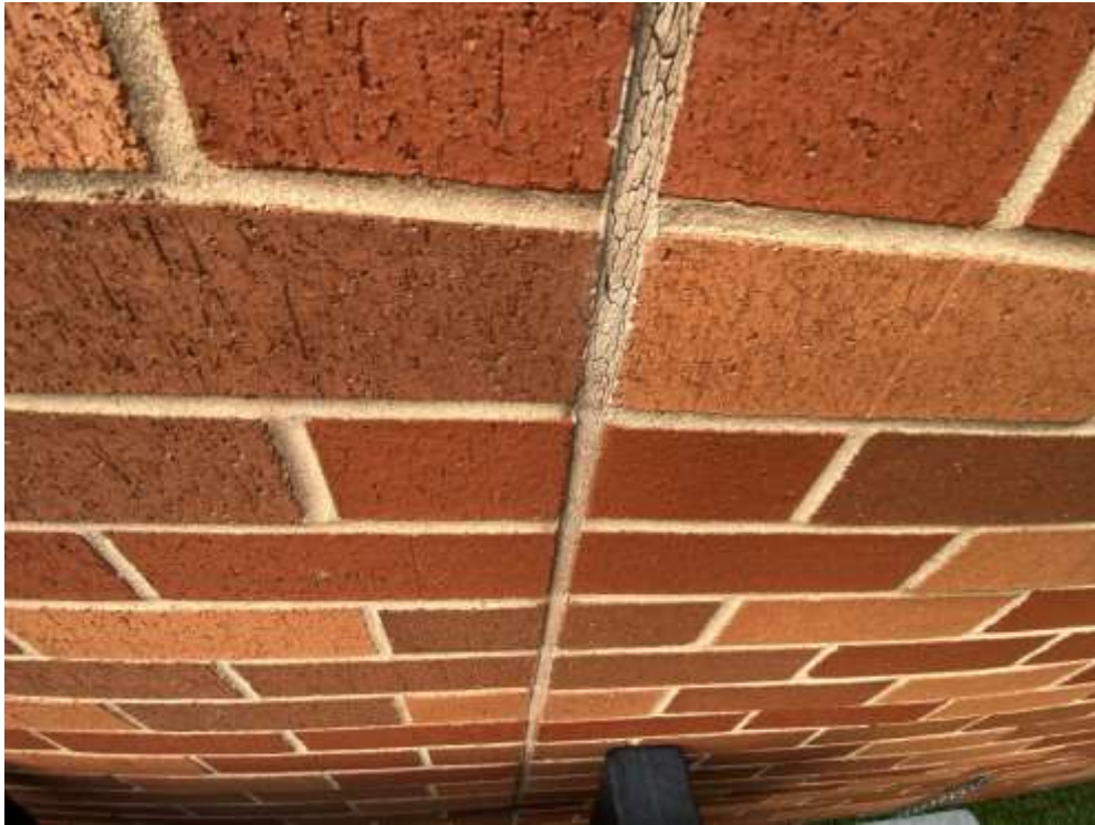
Photo 3 – View of non-asbestos and non-lead-containing mortar on the bricks.
