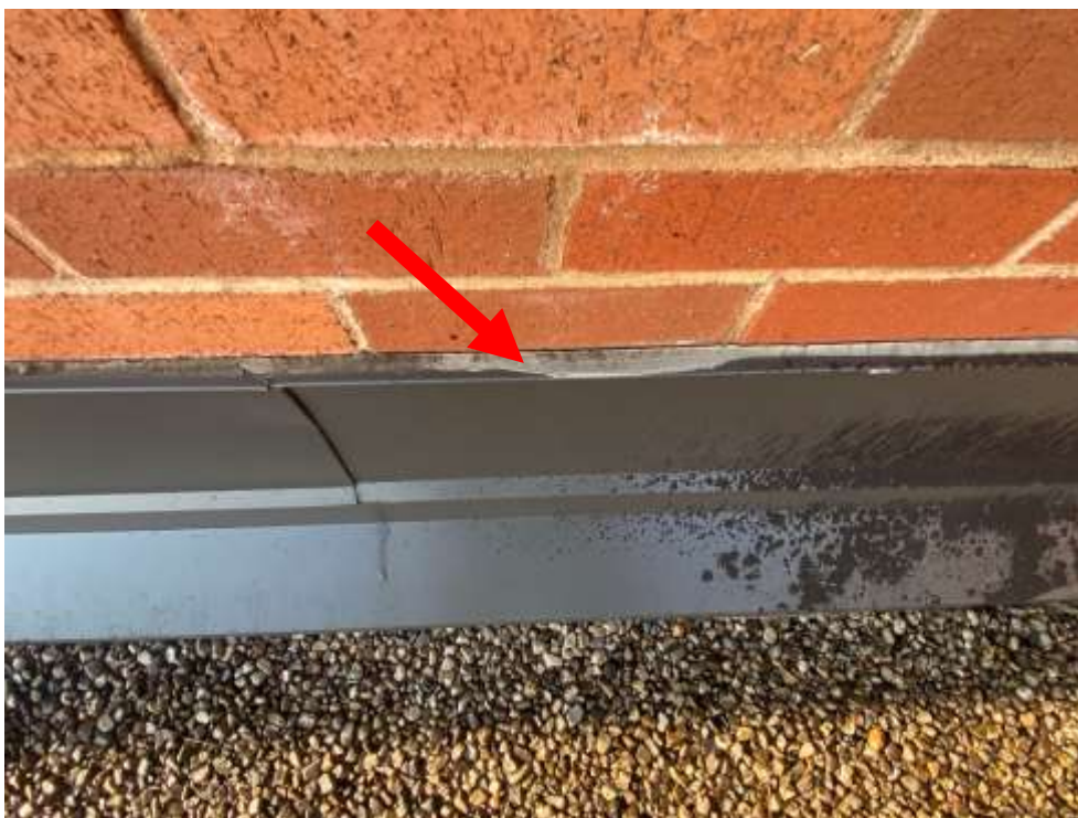
Photo 5 – View of non-asbestos-containing dark grey caulking.
