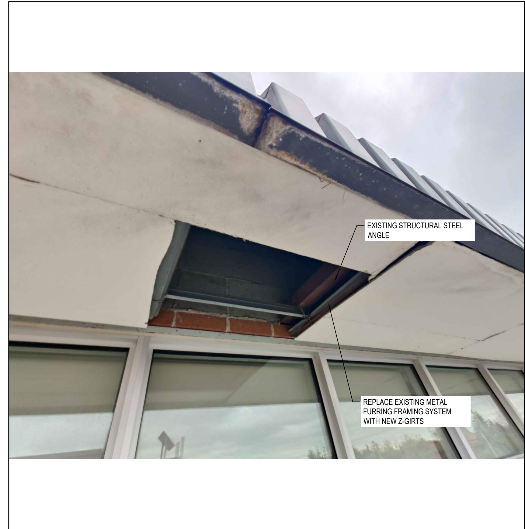
3 EXISTING SOFFIT OPENING R601
