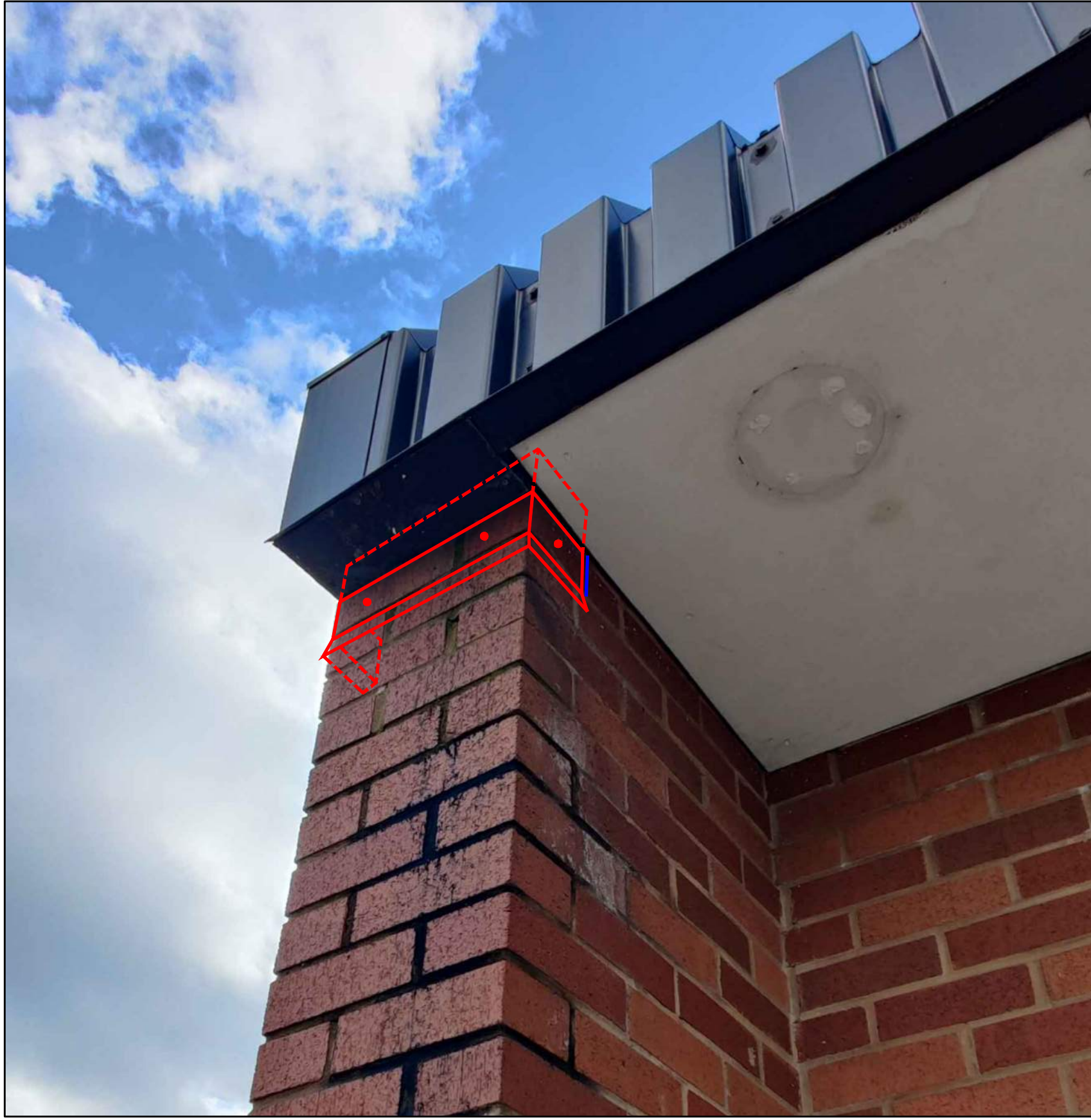
5 SOUTH-EAST CORNER FLASHING R501
