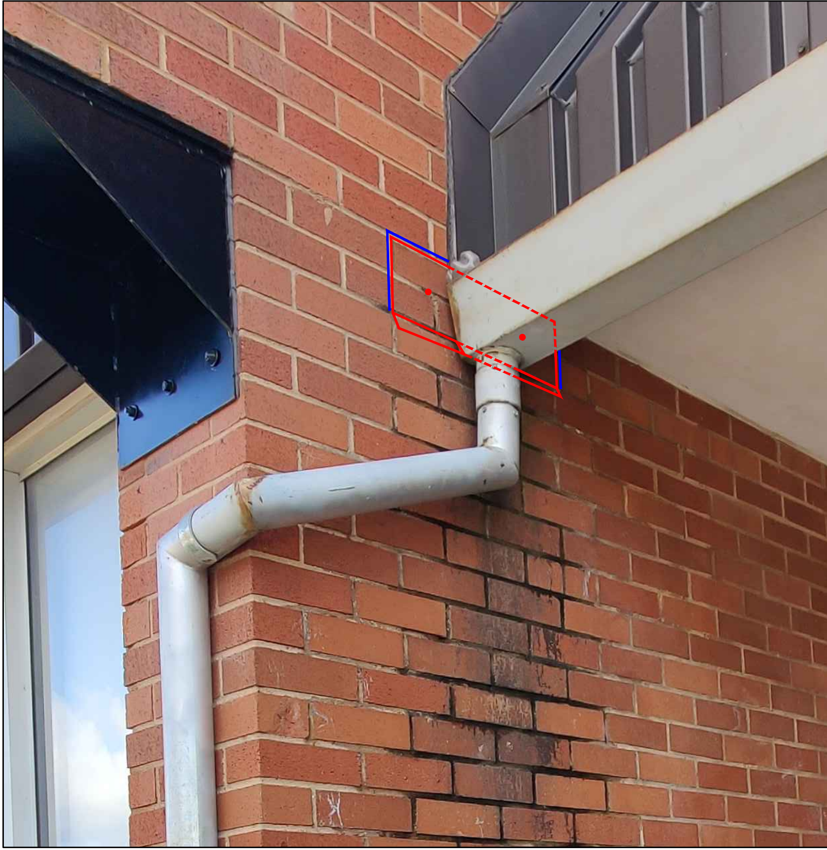
4 SOUTH ELEVATION ENTRANCE 16 - FLASHING R501
