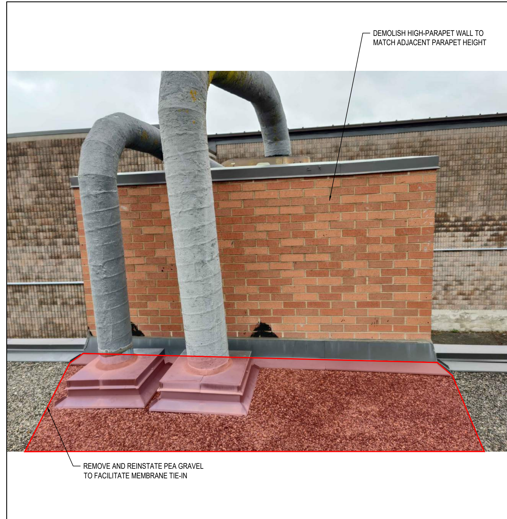
5 WEST ELEVATION - DUST COLLECTOR PARAPET FROM ROOF R601
