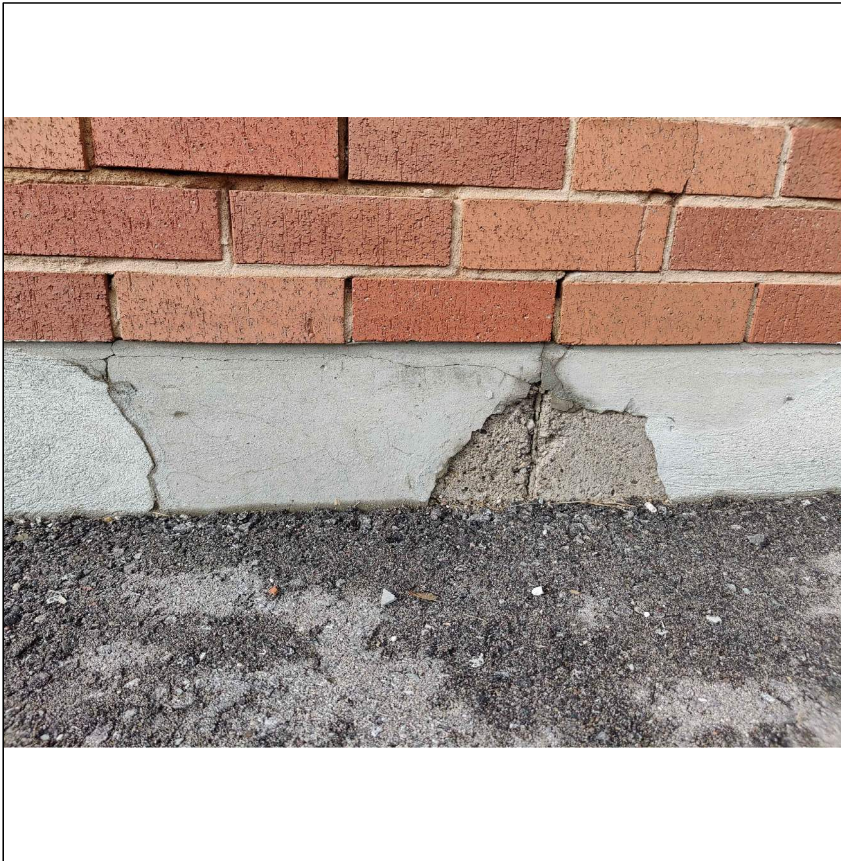
4 TYPICAL PARGING REPAIR R600
