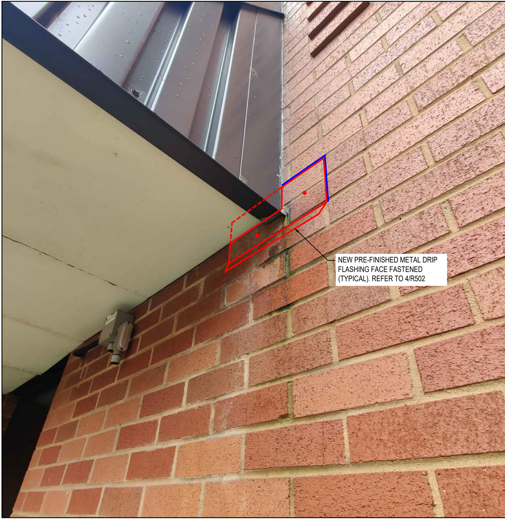
1 COURTYARD CORNER FLASHING R501
