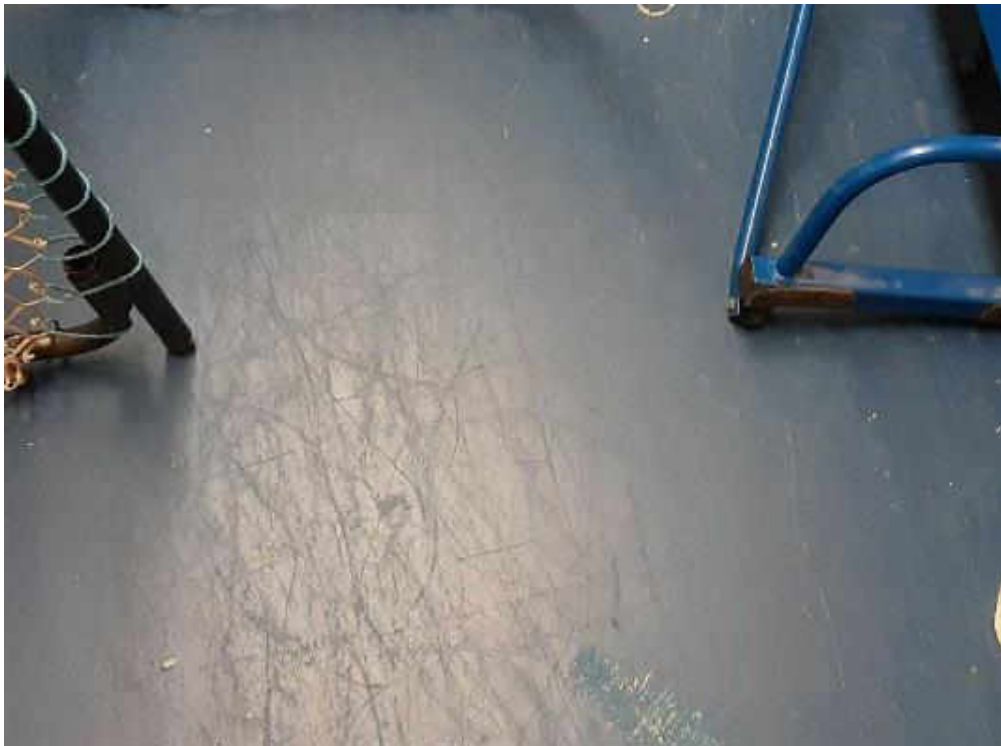
Concrete (poured), Blue, L0020, Gym Storage (Location #: 25)
