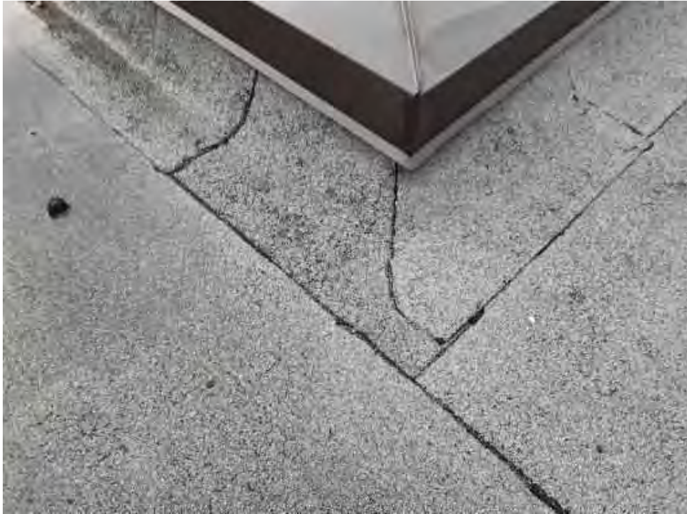
V0000 (None), Other, Roof, Lower Roof (Location #: 17) Built up,
