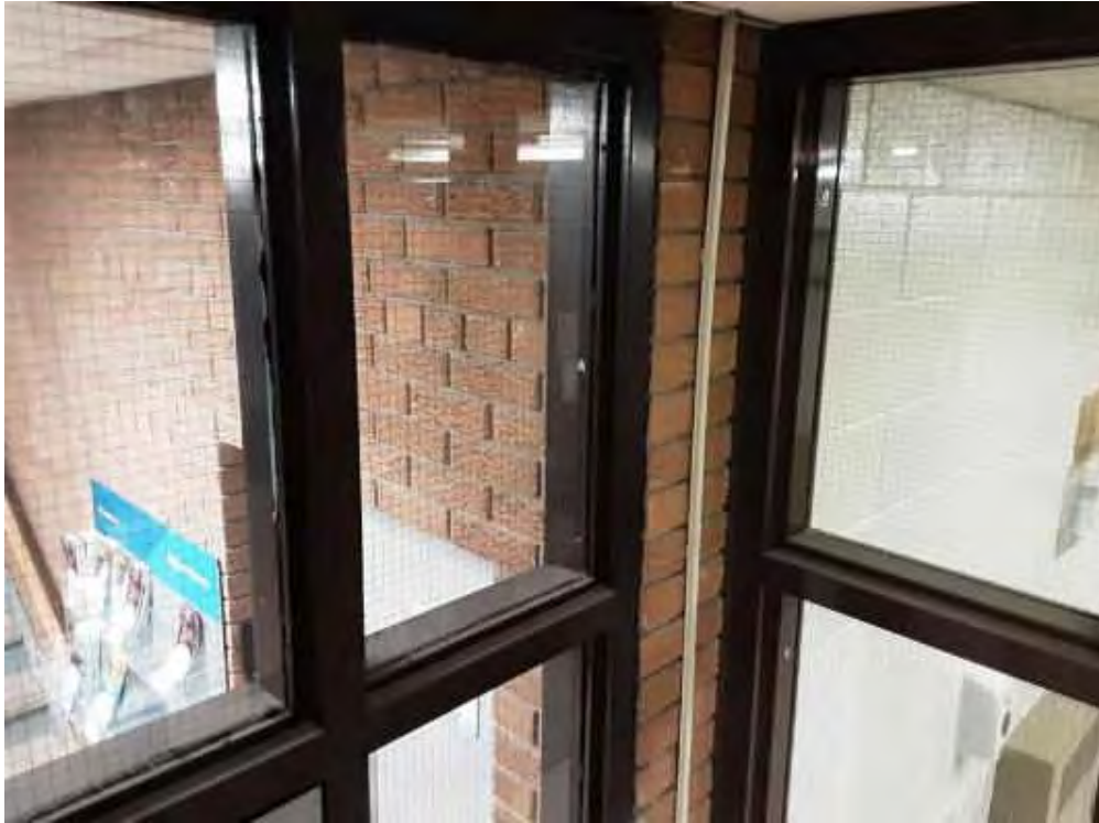
V0000 (None), Wall, All, Masonry, Entrance Vestibule (Location #: 6) Brick wall
