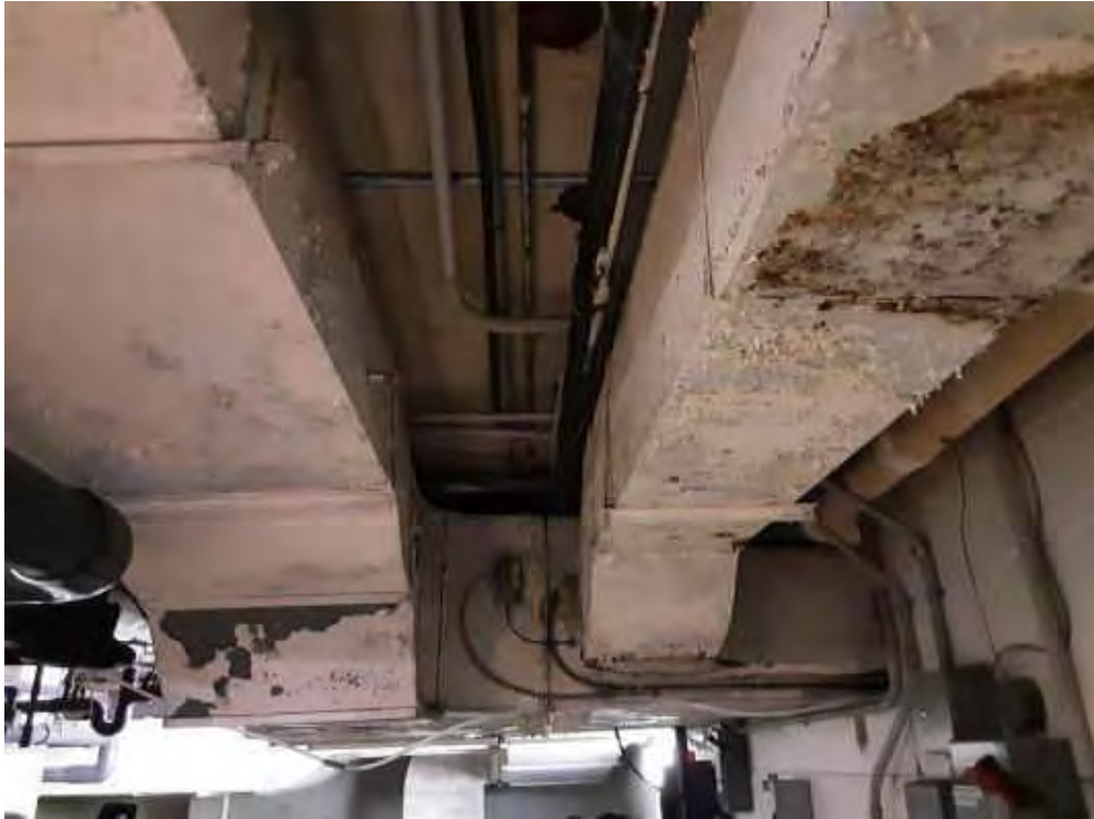
V0000 (None), Duct, All, Not Insulated, Filter Room (Location #: 2)
