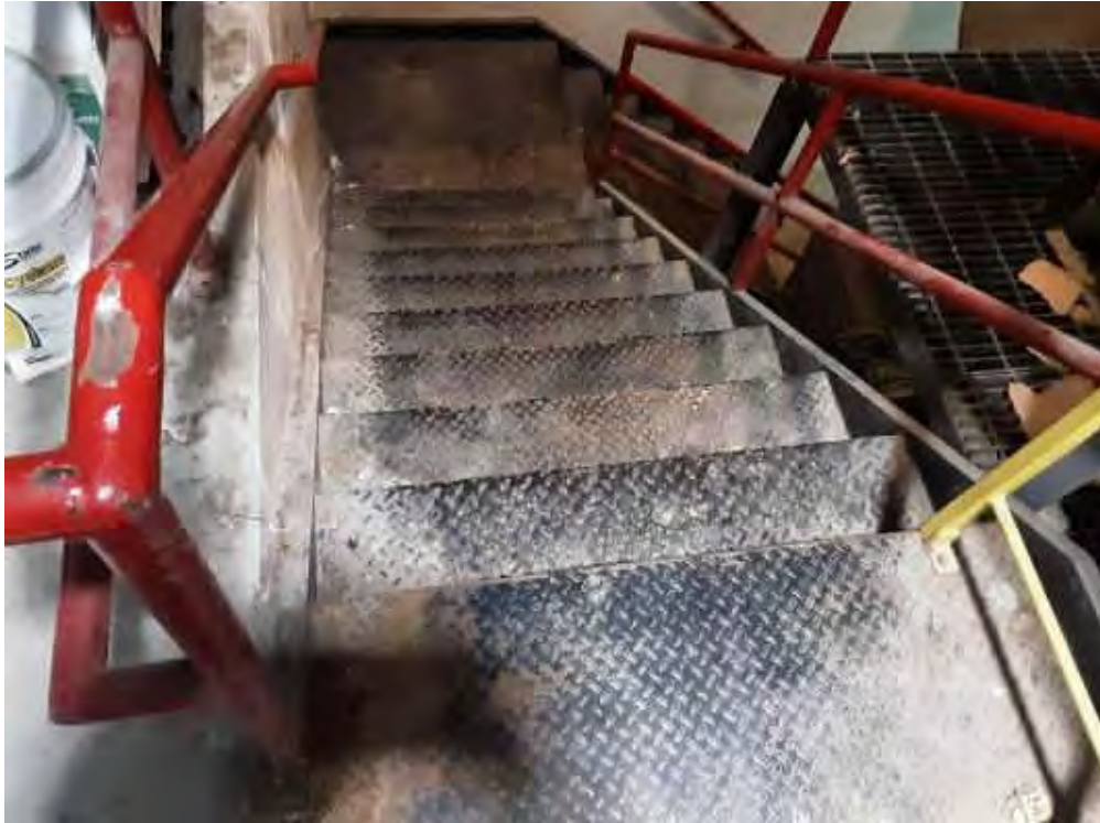
V0000 (None), Other, Stairs, Metal, Mechanical Room And Stairwell (Location #: 21)
