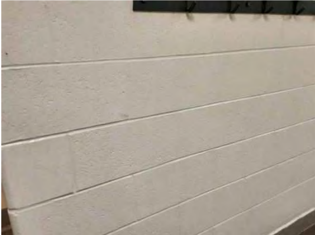
Masonry, White, V0012(Lead (High)), Women's Change Room (Location #: 12)
