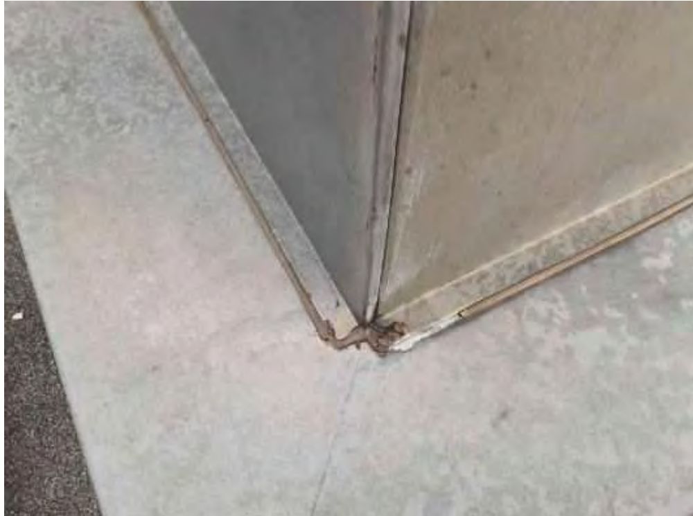
PCB, Lower Roof (Location #: 17)
