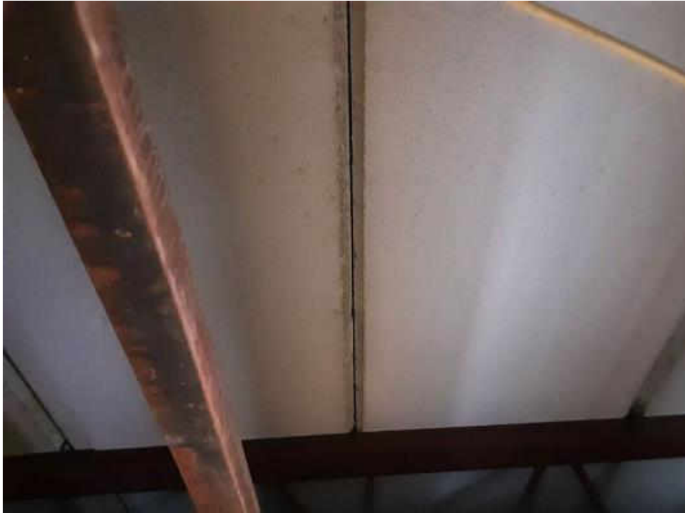
V0000 (None), Structure, All, Concrete (precast), Entrance Vestibule (Location #: 6)
