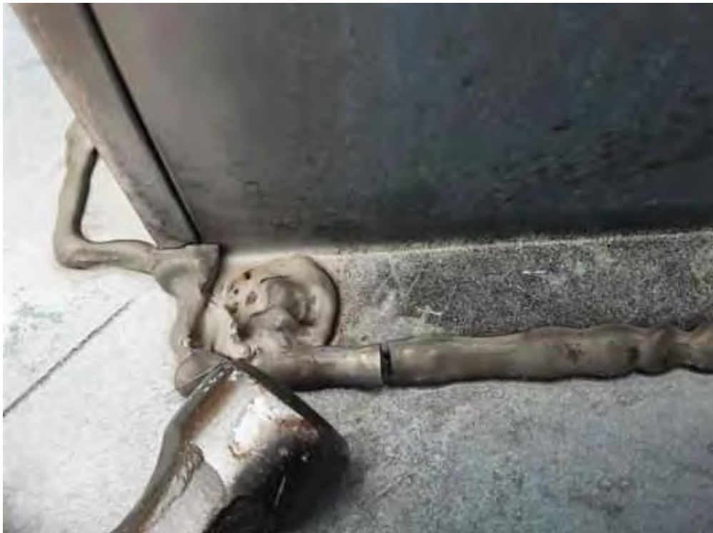
S0021A (None), Duct, Caulking, Lower Roof (Location #: 17) Grey
