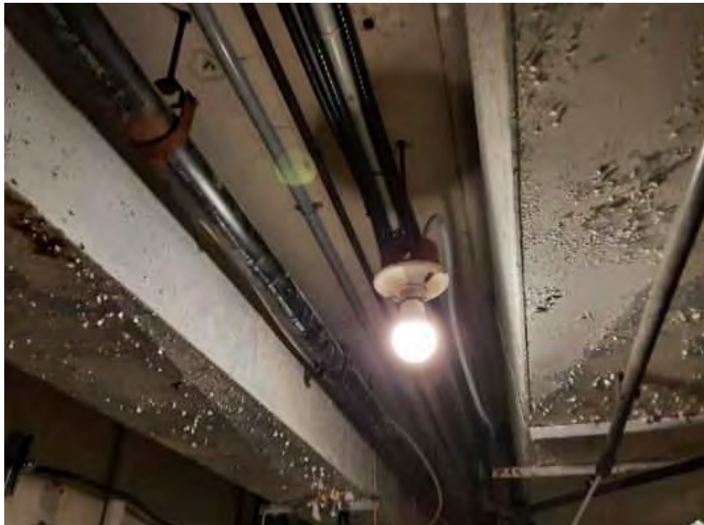
Mercury, Filter Room (Location #: 2)
