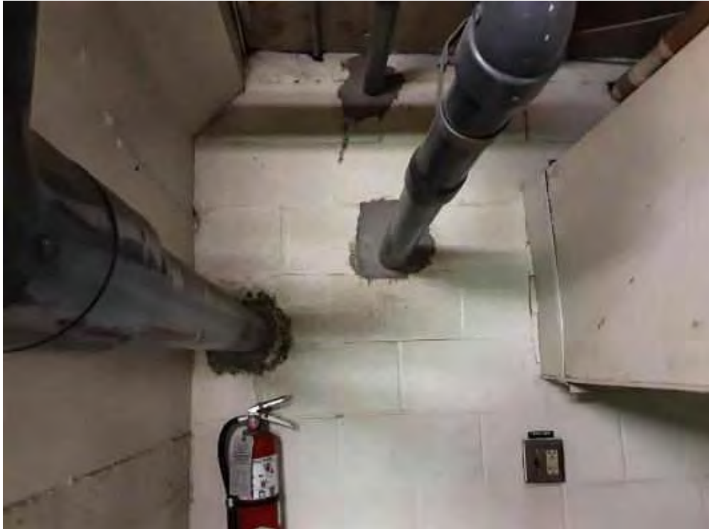
S0002A (None), Wall, Fire Stop, Cement Product, Filter Room (Location #: 2)
