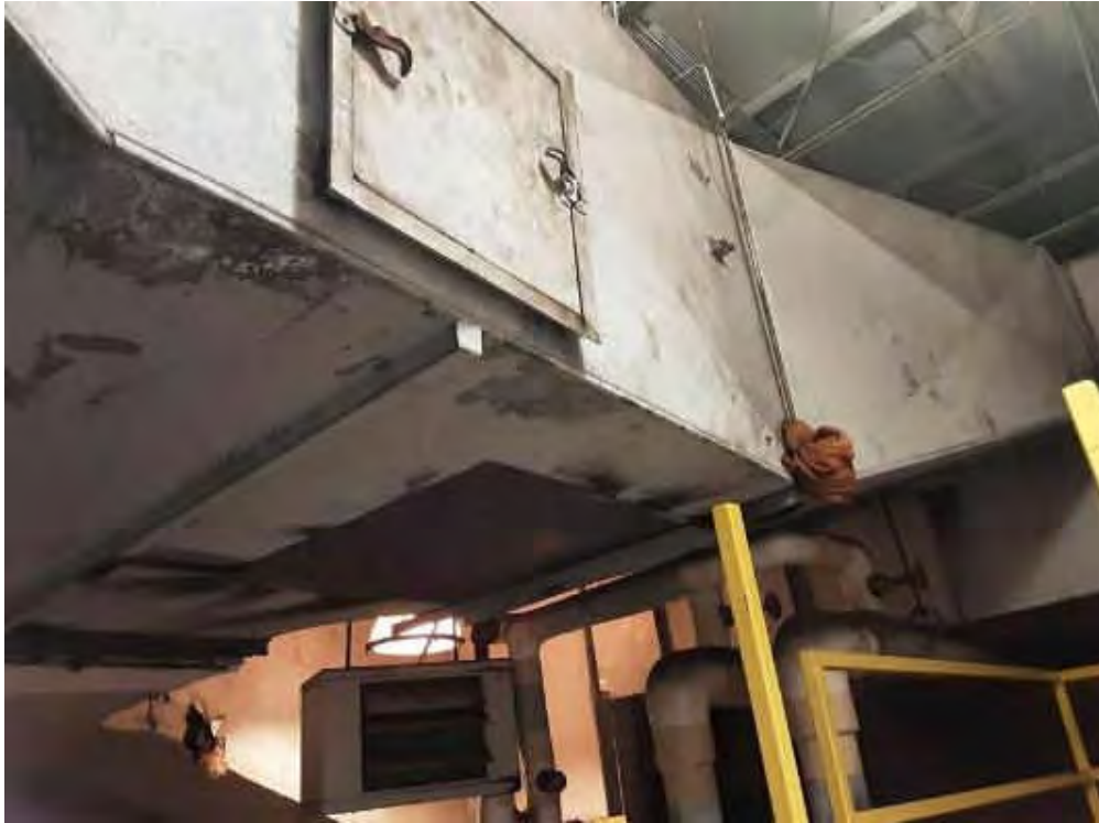
V0000 (None), Duct, Not Insulated, Mechanical Room And Stairwell (Location #: 21)
