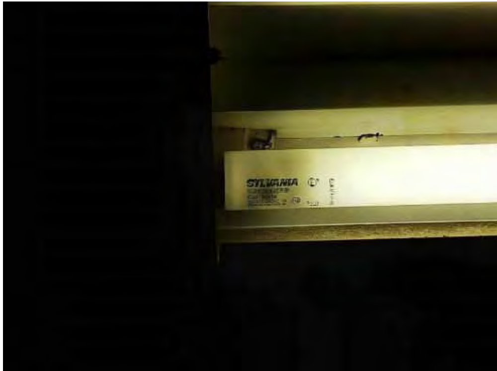
Mercury, Filter Room (Location #: 2)
