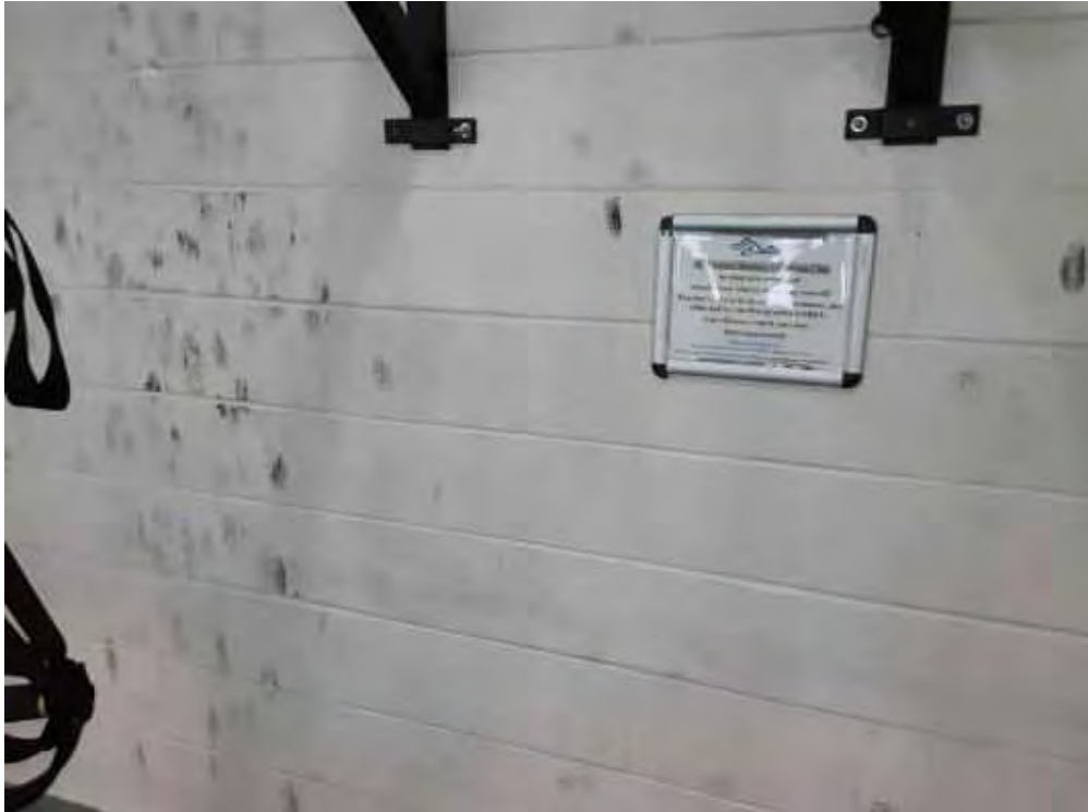
V0000 (None), Wall, All, Masonry, Balcony (Location #: 4) Block wall
