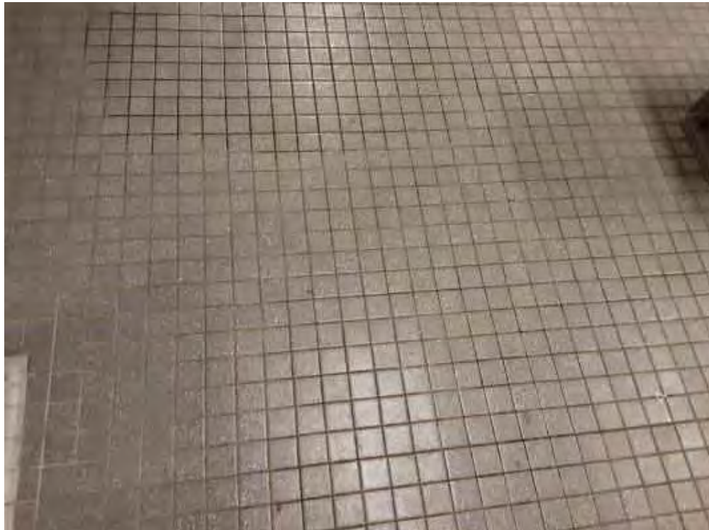
S0009C (None), Floor, All, Mortar, Men's Change Room (Location #: 9)
