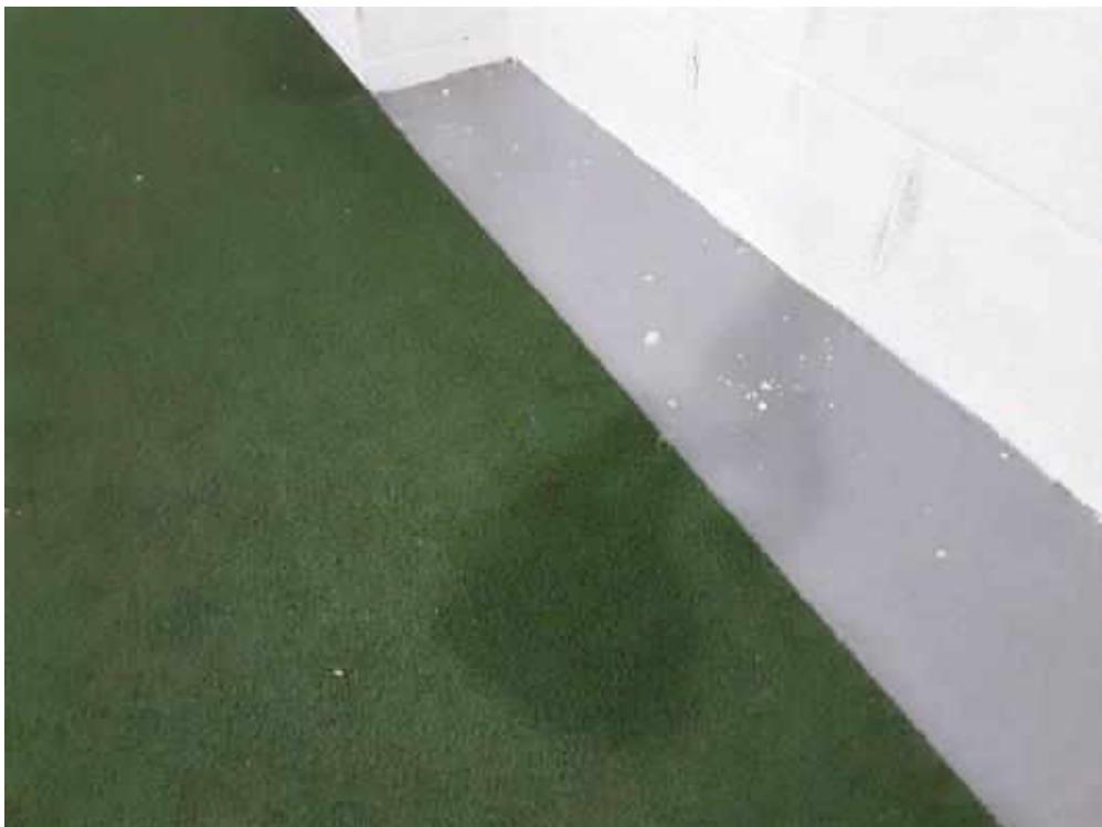
V0000 (None), Floor, All, Concrete (poured), Balcony (Location #: 4)
