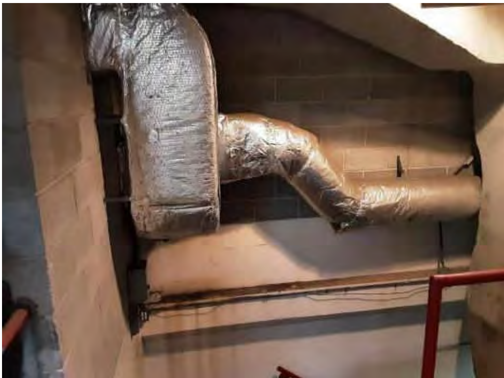
V0000 (None), Duct, All, Fibreglass, Mechanical Room And Stairwell (Location #: 21)
