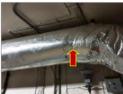
Photo 5: Non-asbestos fiberglass(foil-faced) insulated duct present in the Fan Room (Loc.1).
