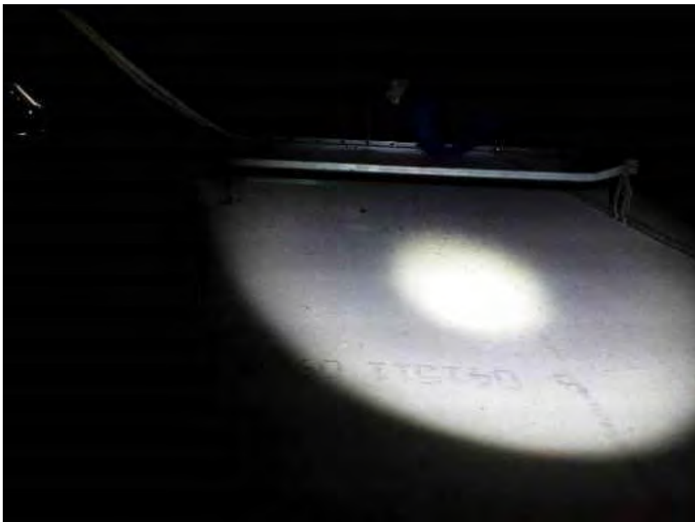
V0000 (None), Ceiling, All, Ceiling Tiles (lay-in), Supervisor Office (Location #: 15) Date stamp- 04/15/11
