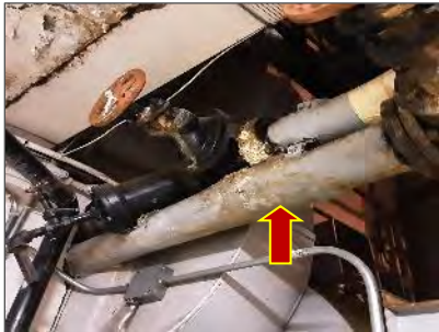
Photo 1: Non-asbestos fiberglass insulated pipe present in the Fan Room (Loc.1)
