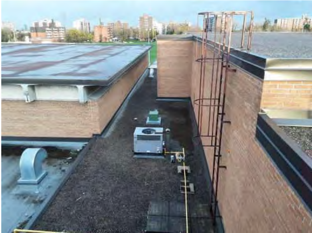
Pool roof (Location #: 18)
