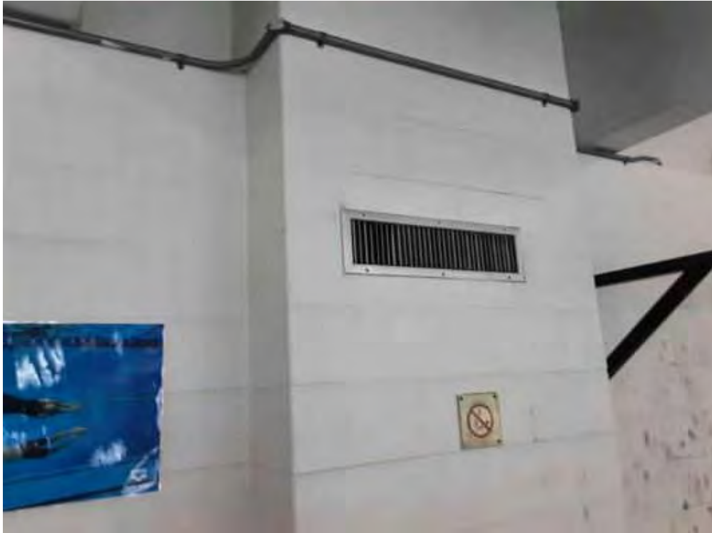
Duct, AI, None Found, Balcony (Location #: 4)
