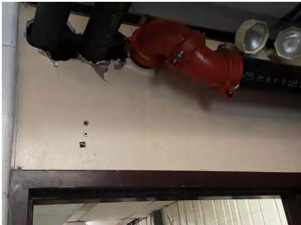
Drywall and joint compound, Light yellow, L0024, Custodian (Location #: 29)
