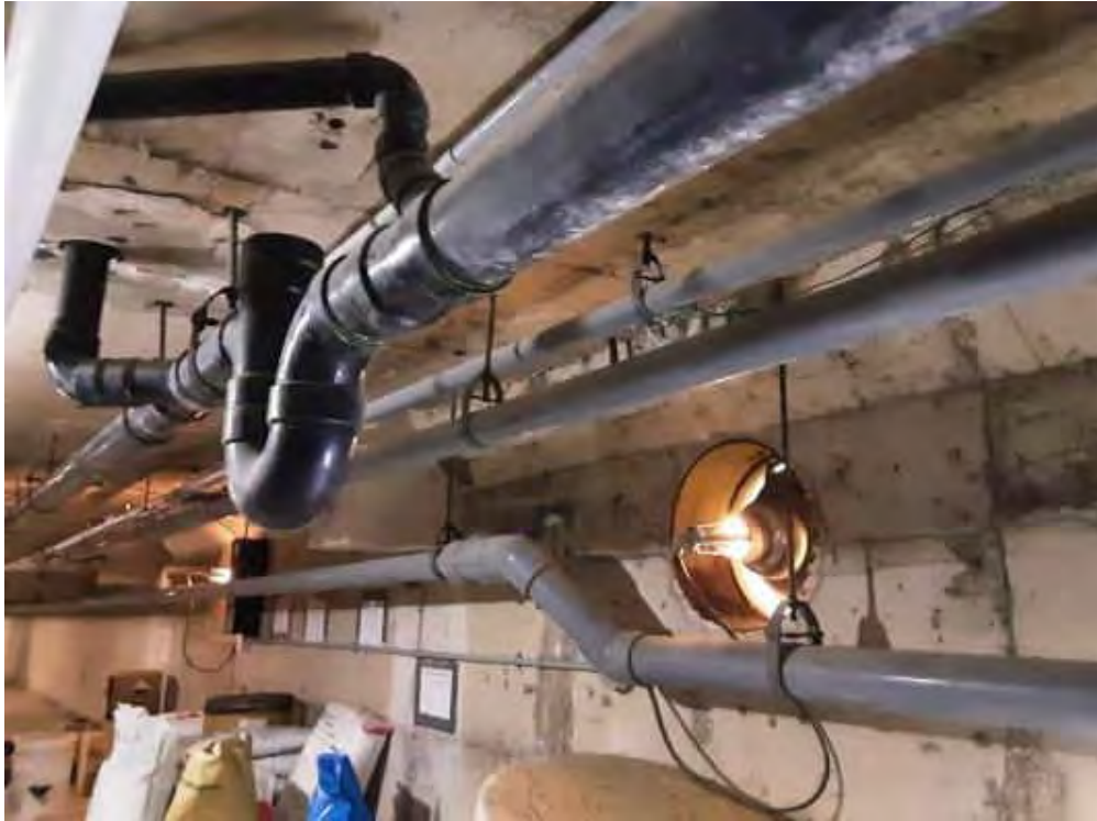
V0000 (None), Piping, Polyvinyl chloride (PVC), Tunnel Area (Location # 3)
