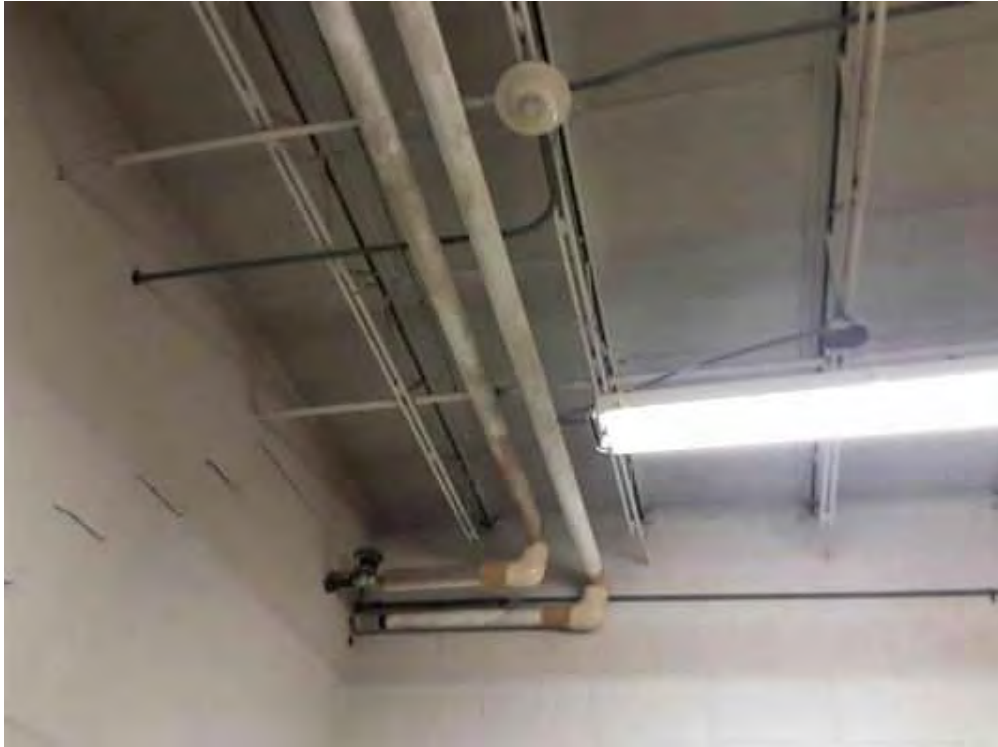
V0000 (None), Piping, All, Fibreglass, Equipment Room 2 (Location #: 20)
