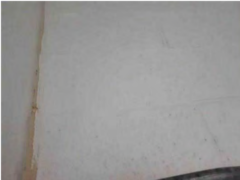
S0003A (None), Wall, Expansion Joint, Caulking, Balcony (Location #: 4) Beige
