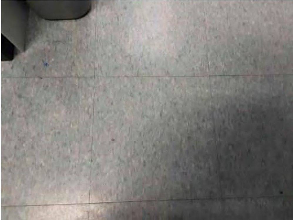
S0019A (None), Floor, Vinyl Floor Tile and Mastic, Supervisor Office (Location #: 15) Black mastic
