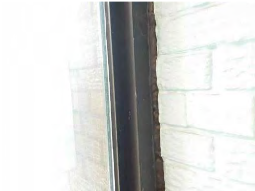
S0016B (Confirmed Asbestos), Other, Door, Caulking, Entrance Vestibule (Location #: 6) Black, between wall and door frame
