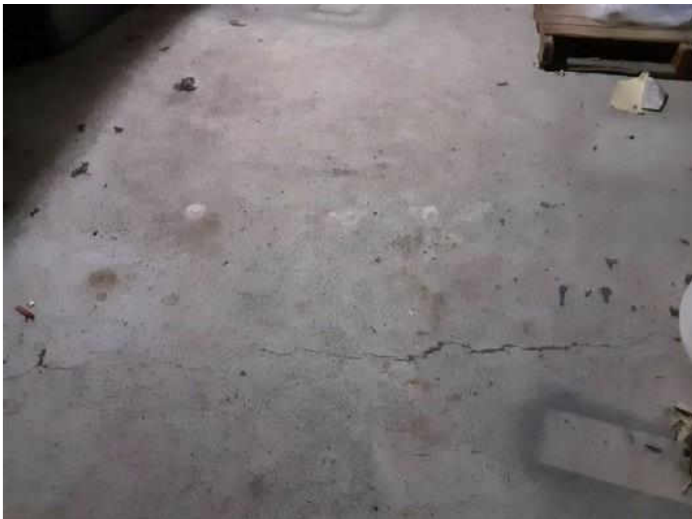
V0000 (None), Floor, All, Concrete (poured), Tunnel Area (Location #: 3)
