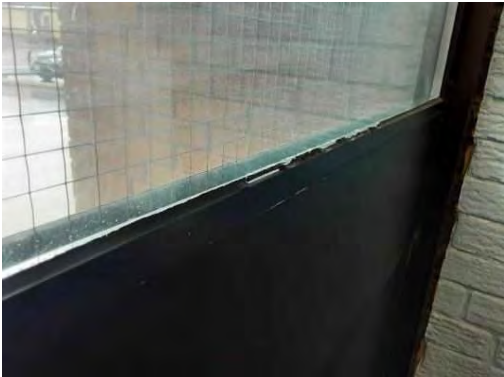
PCB, Entrance Vestibule (Location #: 6)
