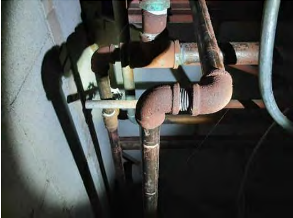
V0000 (None), Piping, Not Insulated, Men's Washroom (Location #: 10)
