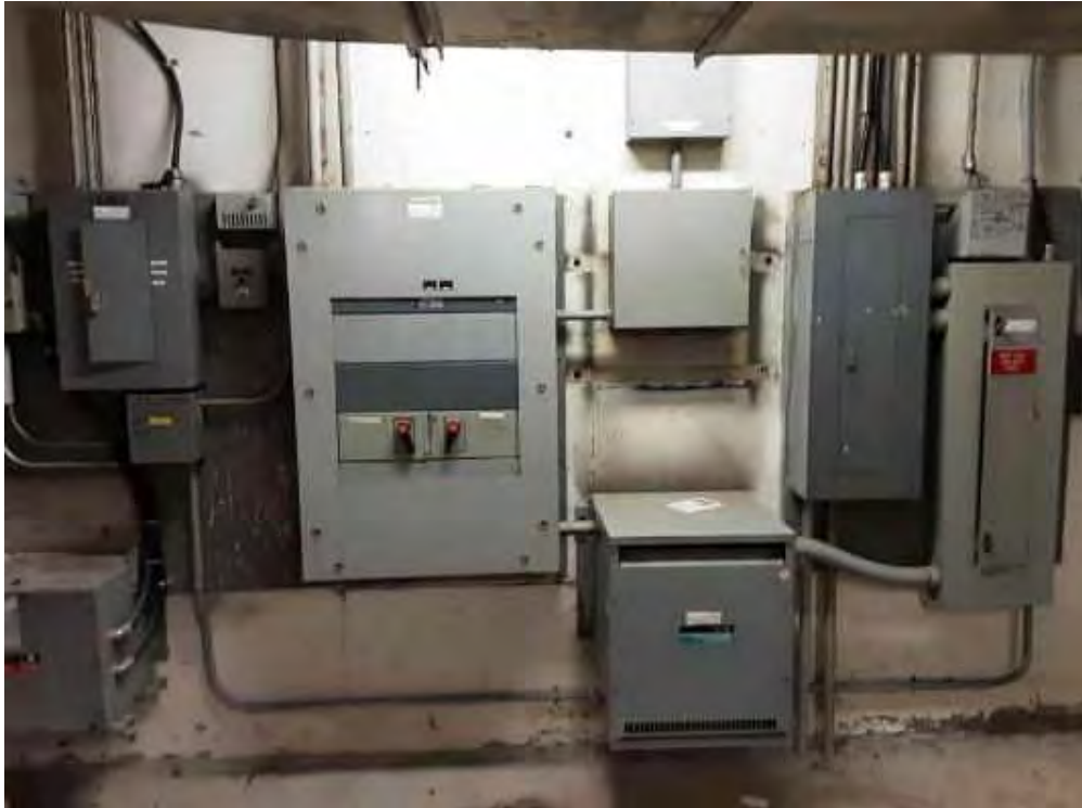
V0000 (None), Other, Electrical Panel, Not Insulated, Filter Room (Location #: 2)
