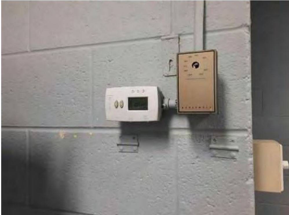
Mercury, Supervisor Office (Location #: 15)
