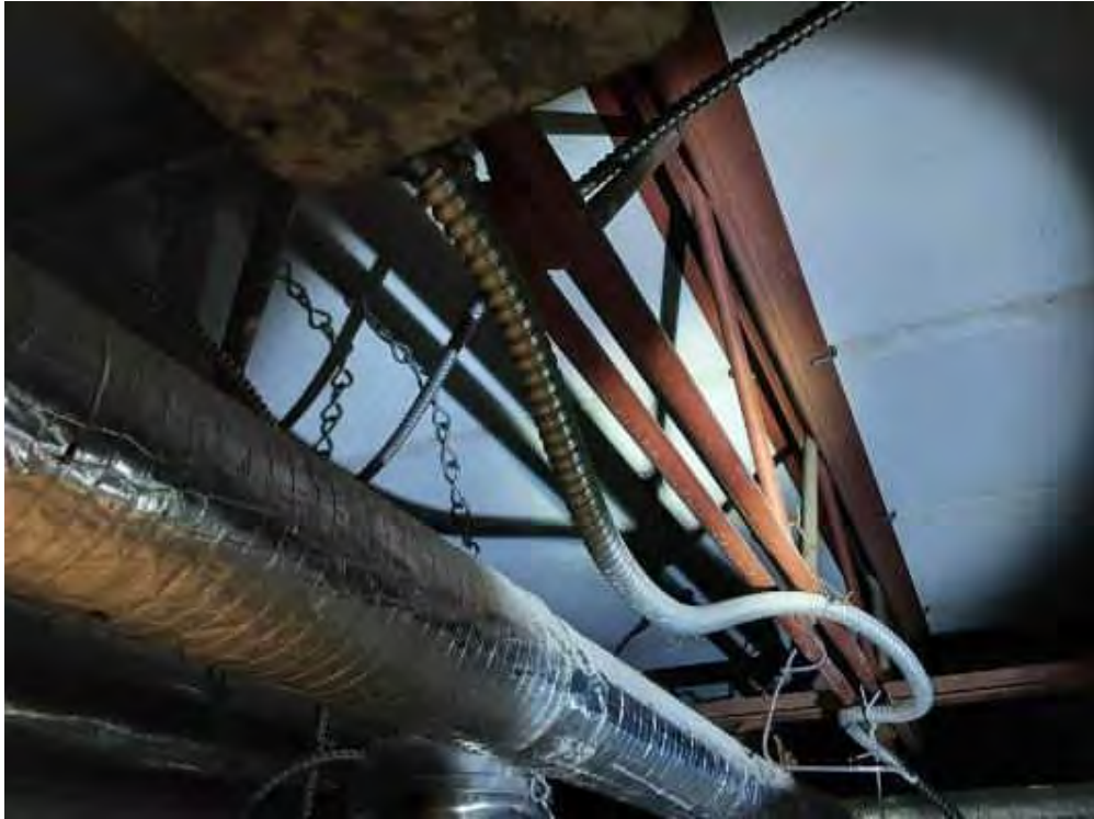
V0000 (None), Structure, Beam, Metal, Lobby (Location #: 7)
