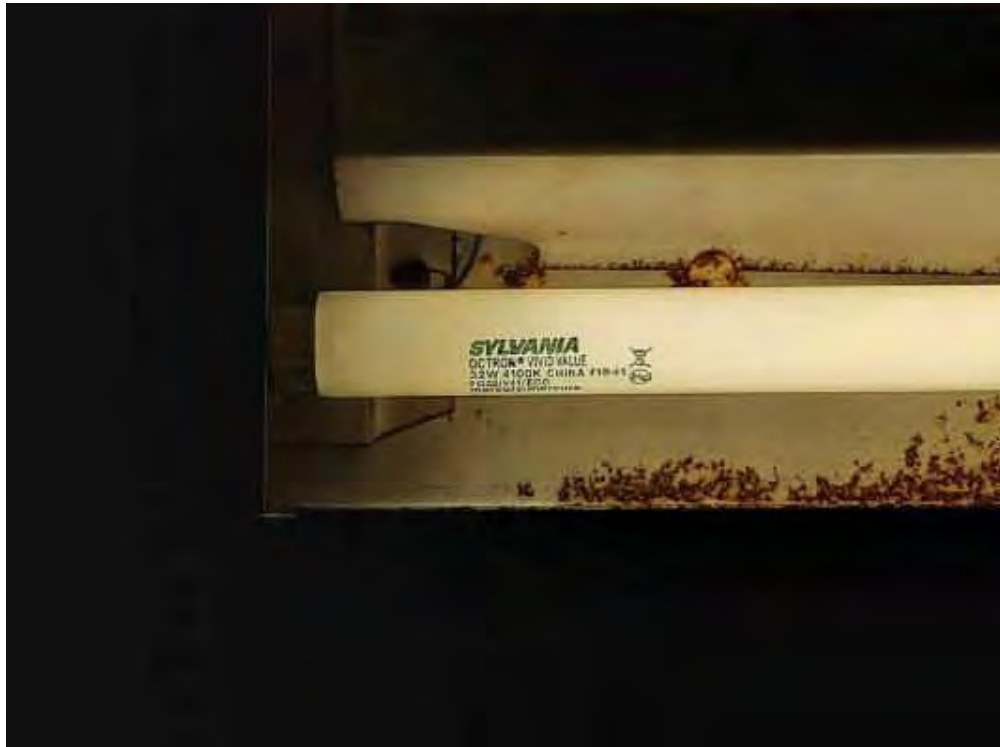
Mercury, Filter Room (Location #: 2)
