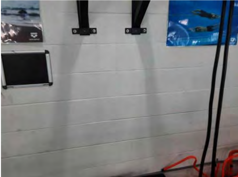
Masonry, Off white, L0008(Lead (Low)), Balcony (Location #: 4)
