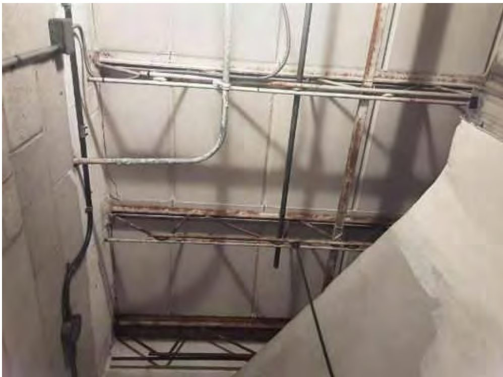
V0000 (None), Structure, All, Concrete (precast), Mechanical Room And Stairwell (Location #: 21)
