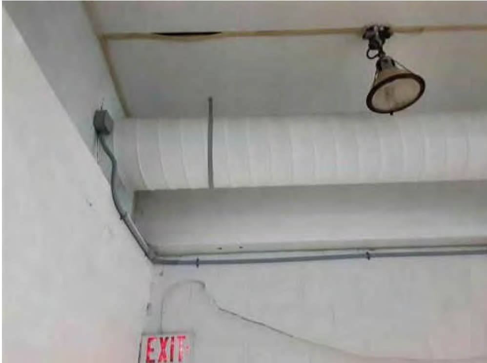
V0000 (None), Duct, All, Not Insulated, East Stairwell (Location #: 5)
