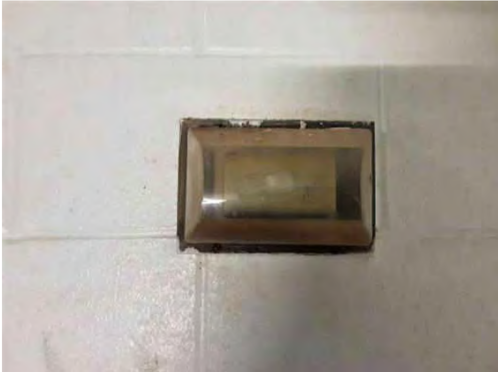
Mercury, East Stairwell (Location #: 5)
