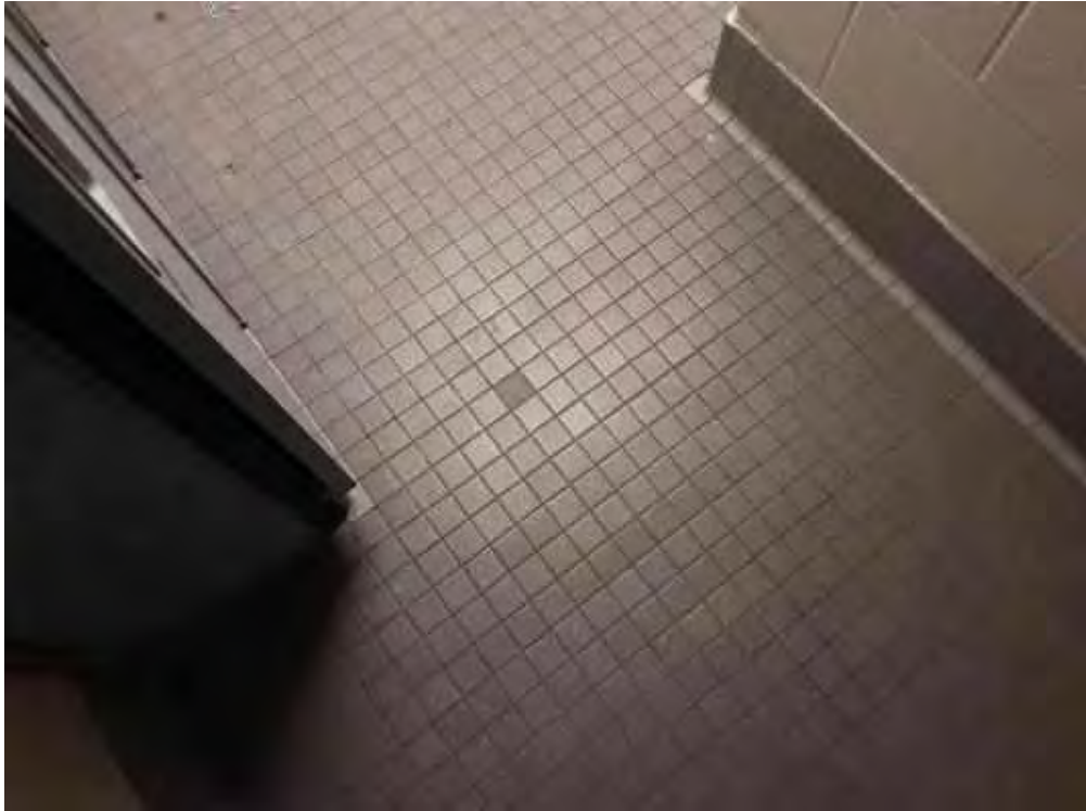
V0000 (None), Floor, All, Ceramic Tiles, Men's Washroom (Location #: 22)
