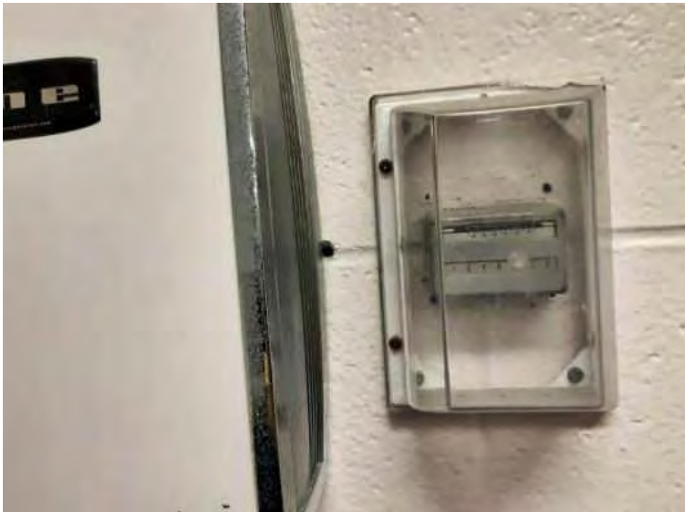
Mercury, Men's Change Room (Location #: 9)
