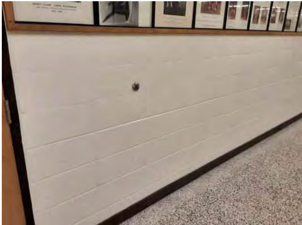
Concrete (poured), Light beige, V0017(Lead (Low)), Corridor (Location #: 27)
