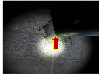
Photo 21: Non-asbestos firestopping (cementitious) present in Tunnel Area (Loc. 3).
