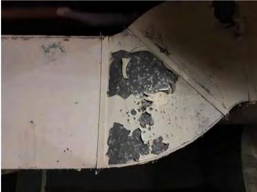
Metal, Off white, L0004(Lead (Low)), Filter Room (Location #. 2)
