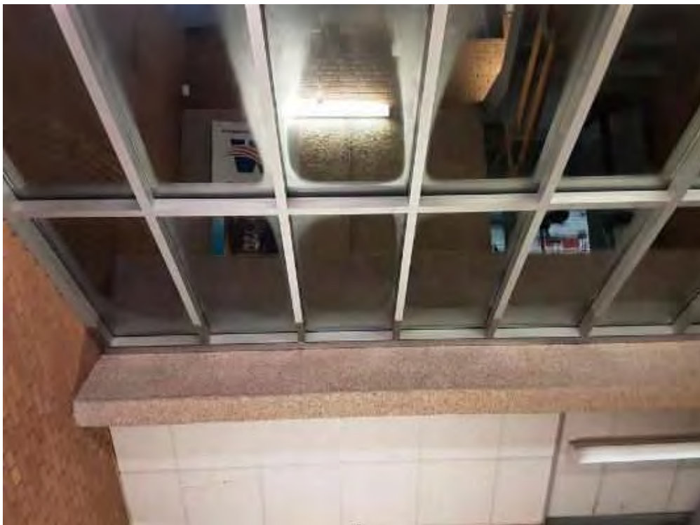
V0000 (None), Other, Skylight, Aluminum, Lobby (Location #: 7) Glass windows
