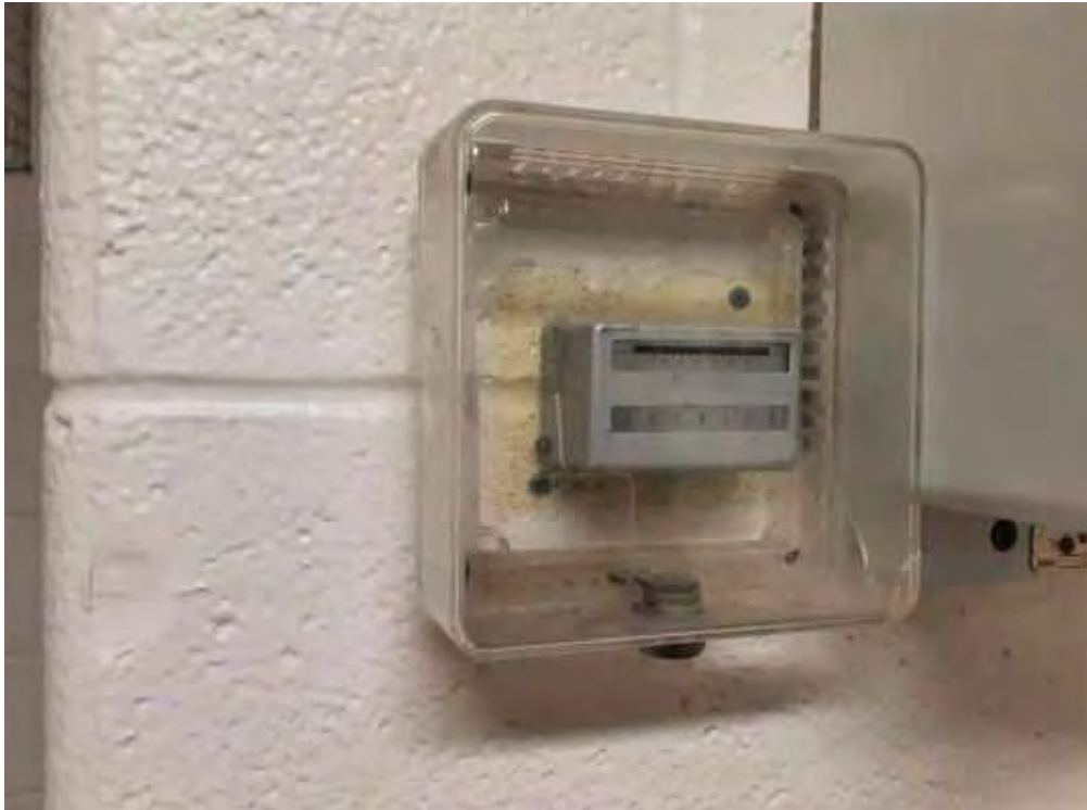
Mercury, Women's Change Room (Location #: 12)
