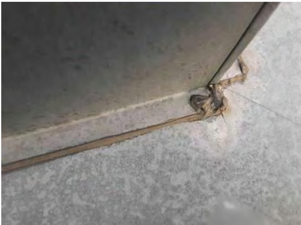
S0021C (None), Duct, Caulking, Lower Roof (Location #: 17) Grey
