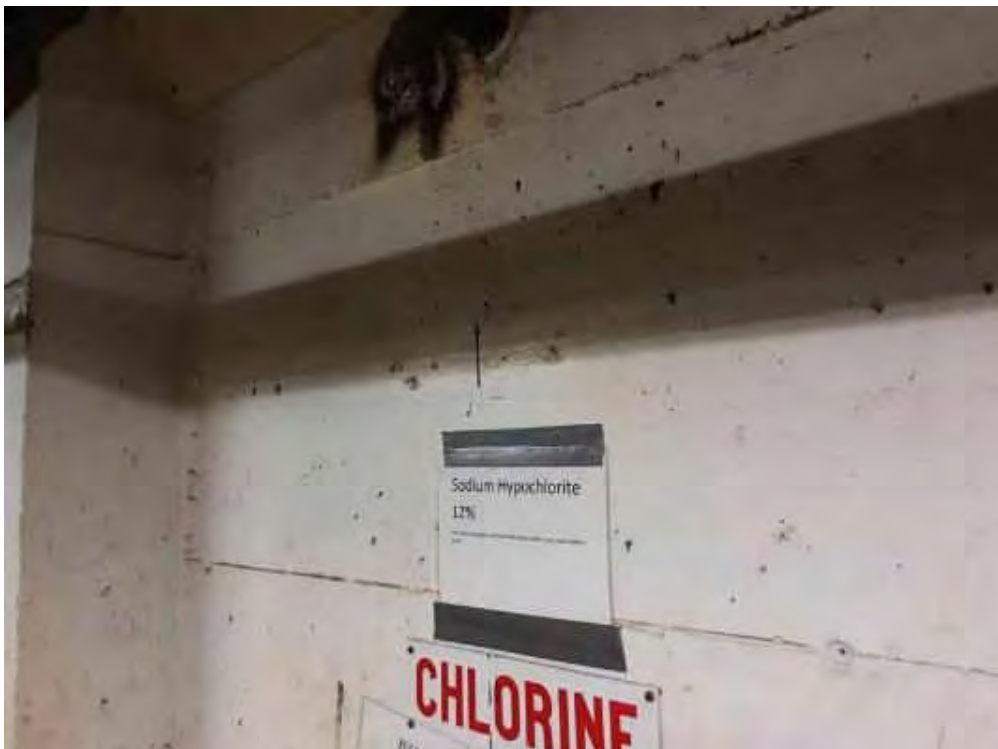
V0000 (None), Wall, All, Concrete (poured), Filter Room (Location #: 2)
