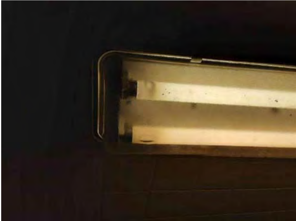
Mercury, Women's Change Room (Location #: 12)
