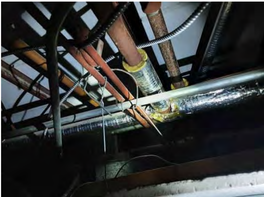
V0000 (None), Piping, All, Fibreglass, Men's Wash room (Location #: 10)
