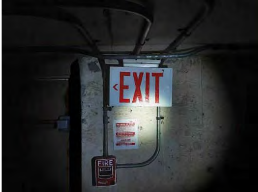
Pb Products, Tunnel Area (Location #: 3)
