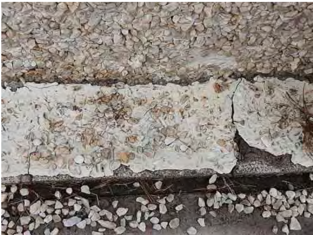
S0014C (None), Wall, Unidentified Material, Exterior (Location #: 14)
