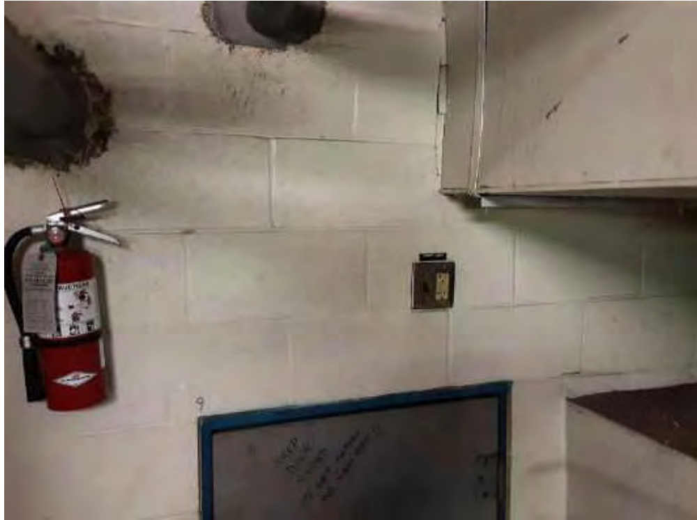
Masonry, Off white, L0005(Lead (Low)), Filter Room (Location #: 2)
