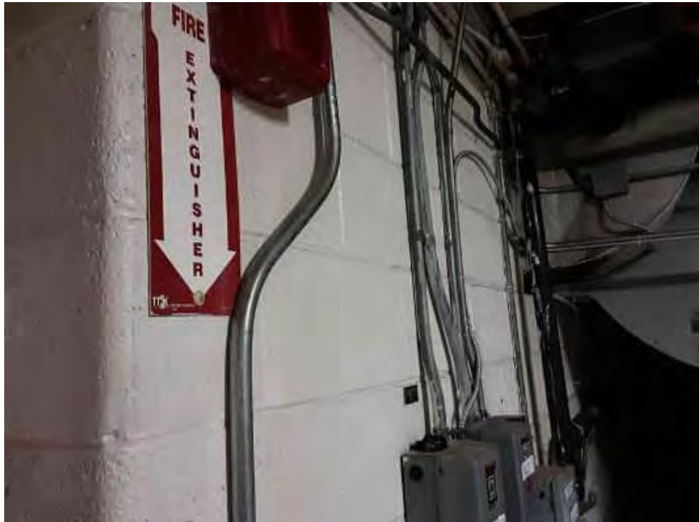
S0001A (None), Wall, Mortar, Fan Room (Location #: 1) Block wall
