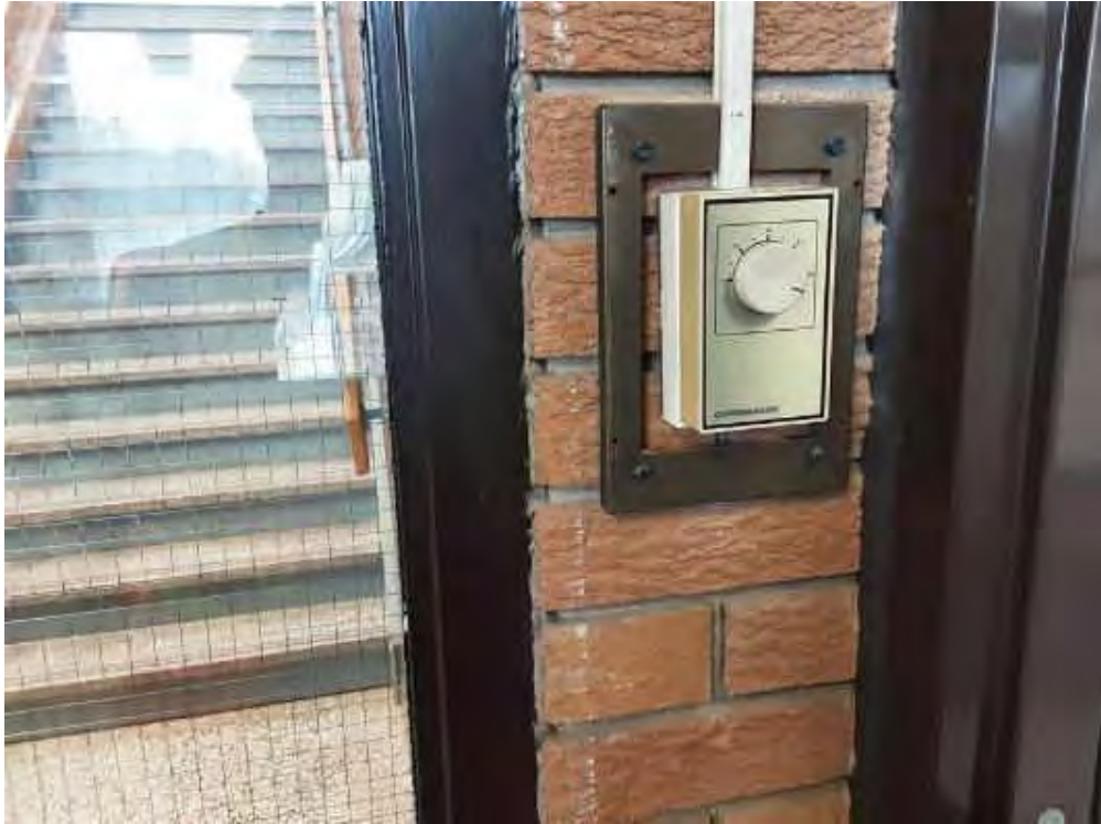
Mercury, Entrance Vestibule (Location #: 6)
