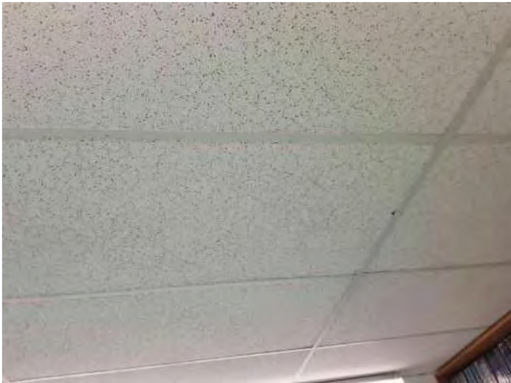
V0000 (None), Ceiling, All, Ceiling Tiles (lay-in), Phys. Ed. Room (Location #: 24)
