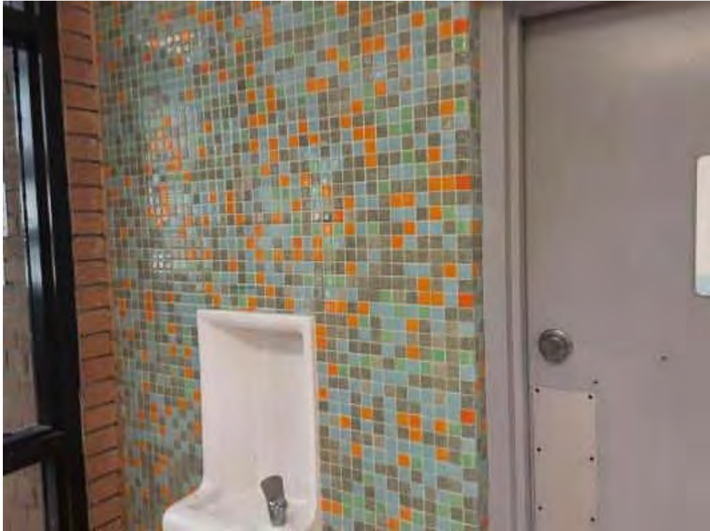
S0027A (None), Wall, Mortar, Lobby (Location #: 7)
