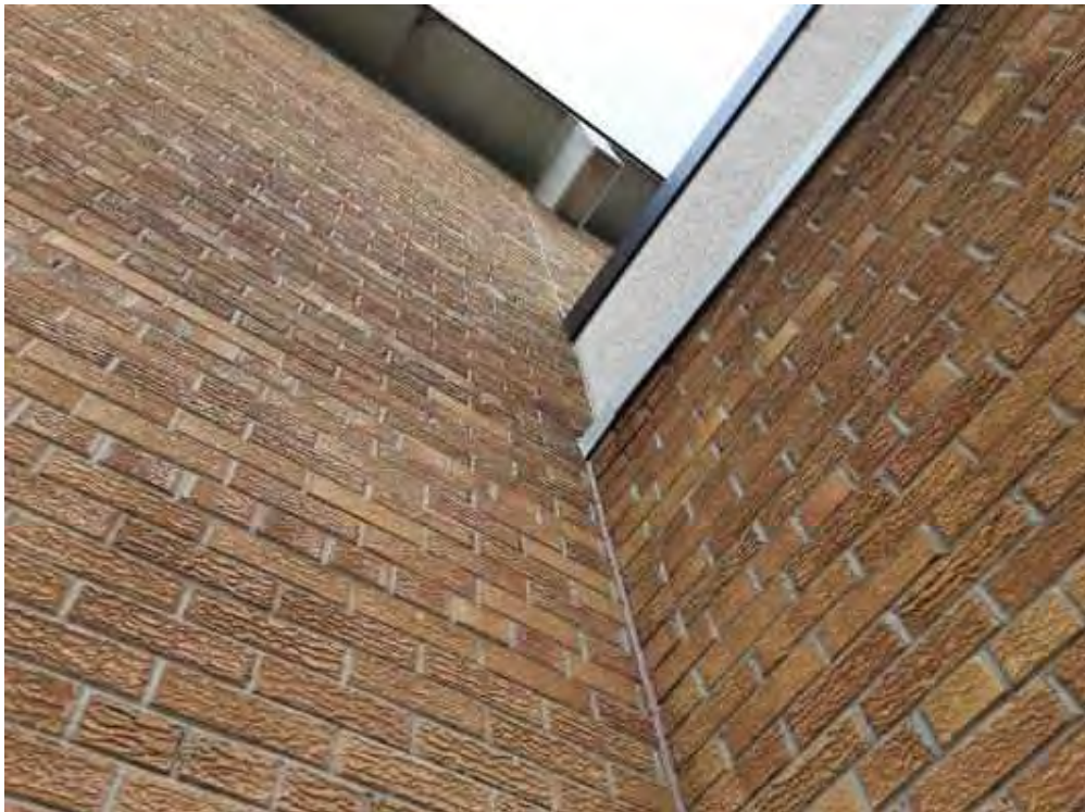
S0011A (None), Wall, Expansion Joint, Caulking, Exterior (Location #: 14) Light red
