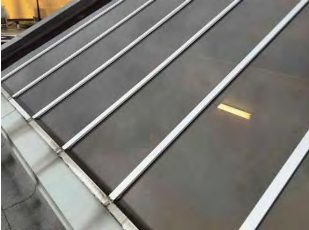
V0000 (None), Other, Skylight, Aluminum, Lower Roof (Location #: 17) Glass
