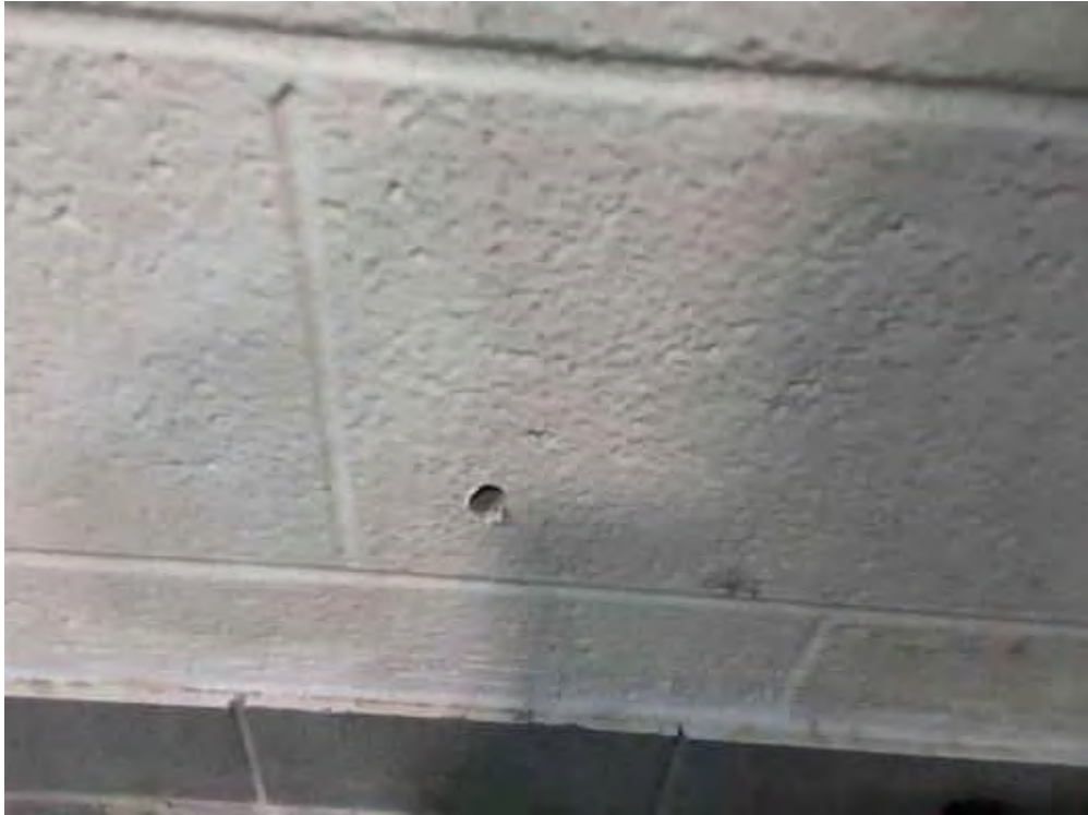
V0000 (None), Wall, Vermiculite/concrete block walls, In do or Pool (Location #: 13) 4 Drill holes, no vermiculite, N wall, E wall, W wall, S wall
