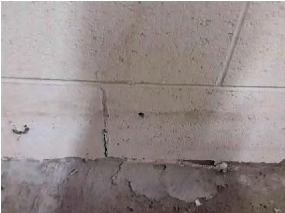
V0000 (None), Wall, Filter Room (Location #: 2) No vermiculite
