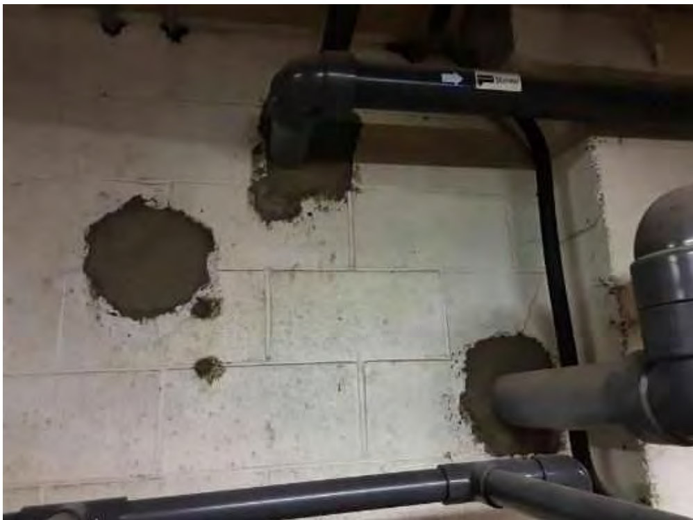
S0002B (None), Wall, Fire Stop, Cement Product, Filter Room (Location #: 2)
