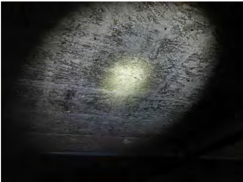
V0000 (None), Structure, All, Concrete (poured), Tunnel Area (Location #: 3)
