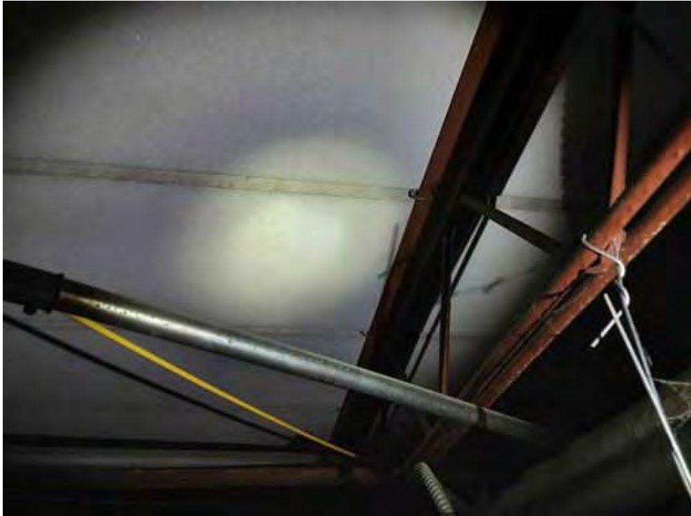
V0000 (None), Structure, All, Con crete (precast), Lobby (Location #: 7)
