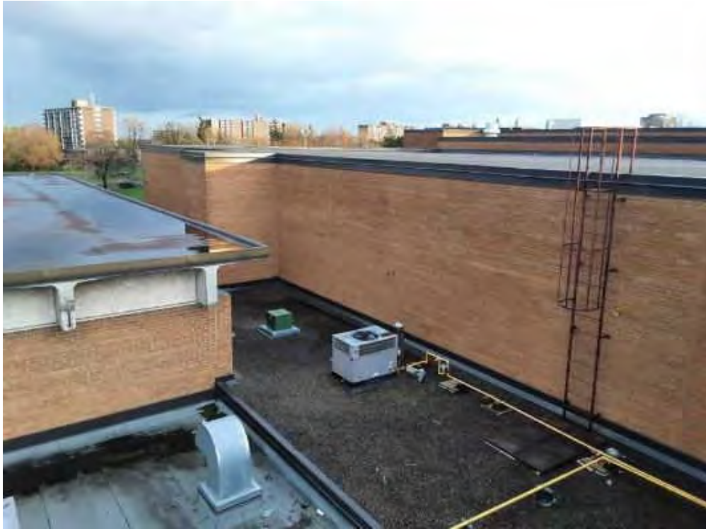
Lower Roof (Location #: 17)
