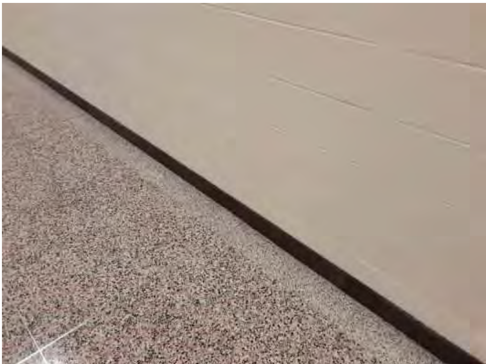
V0000 (None), Wall, All, Masonry, Corridor (Location #: 27) Block wall
