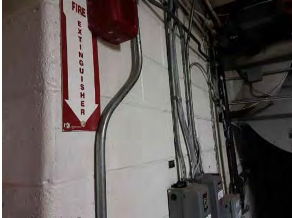
V0000 (None), Wall, Masonry, Fan Room (Location #: 1) Block wall
