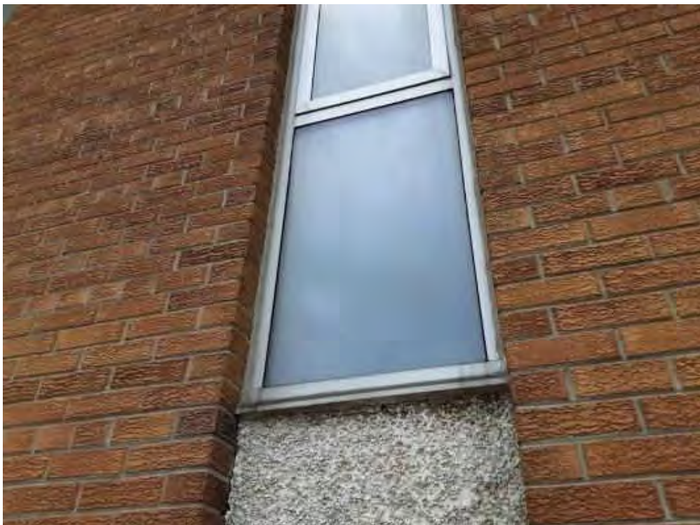
S0015A (None), Other, Window, Caulking, Exterior (Location #: 14) Light Grey, S wall
