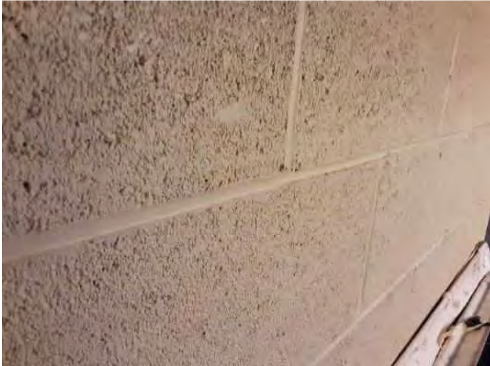
Masonry, Beige, L0019(Lead (Low)), Gym Storage (Location #: 25)
