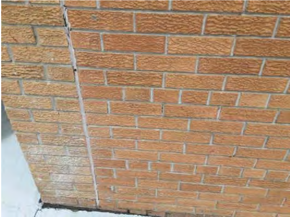
S0012C (Confirmed Asbestos), Wall, Mortar, Exterior (Location #: 14) Brick
