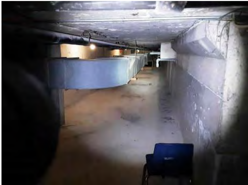
Tunnel Area (Location #: 3)
