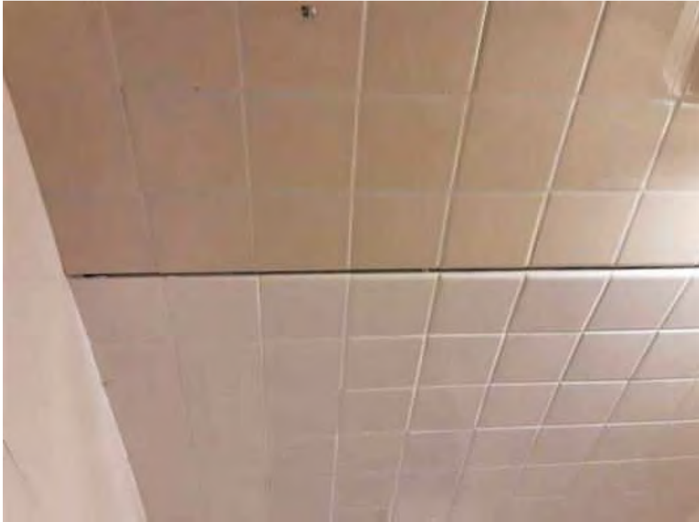
V0000 (None), Ceiling, Ceramic Tiles, Men's Change Room (Location #: 9)
