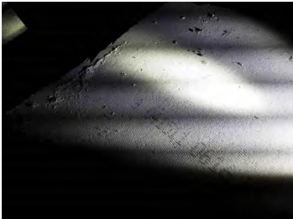
V0000 (None), Ceiling, All, Ceiling Tiles (lay-in), Women's Change Room (Location #: 12) Date stamp- 04/15/11
