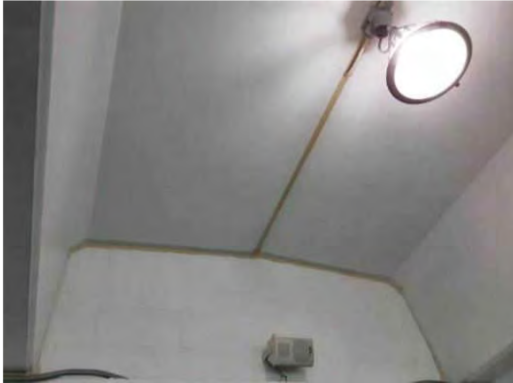
S0003C (None), Wall, Expansion Joint, Caulking, Balcony (Location #: 4) Beige
