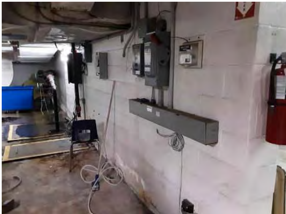
S0001B (None), Wall, Mortar, Filter Room (Location #: 2) Block wall
