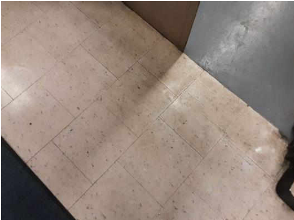
S0032A (None), Floor, All, Vinyl Floor Tile and Mastic, Hallway (Location #: 28)
