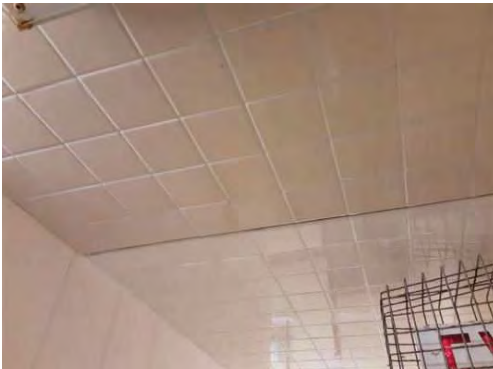
Ceiling, Ceramic Tiles, Women's Change Room (Location #: 12)
