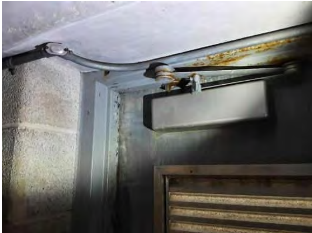
Metal, Grey, L0015(Lead (Low)), Mechanical Room And Stairwell (Location #: 21)
