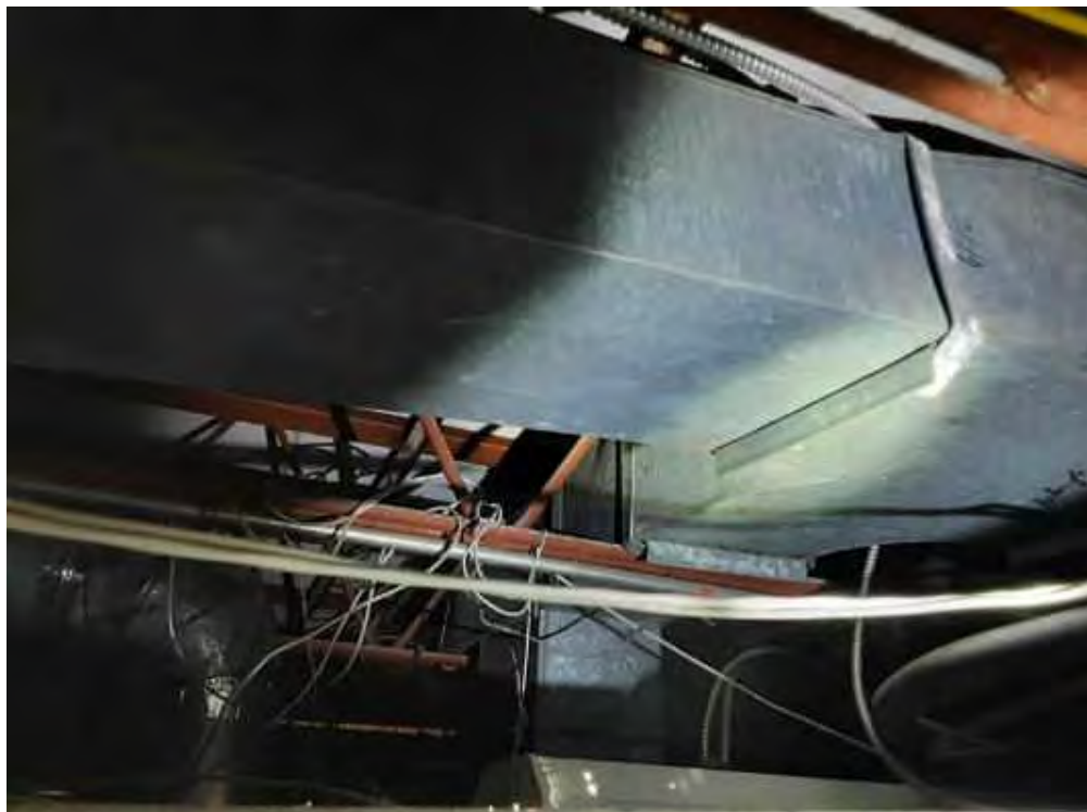
V0000 (None), Duct, All, Not Insulated, Supervisor Office (Location #: 15)
