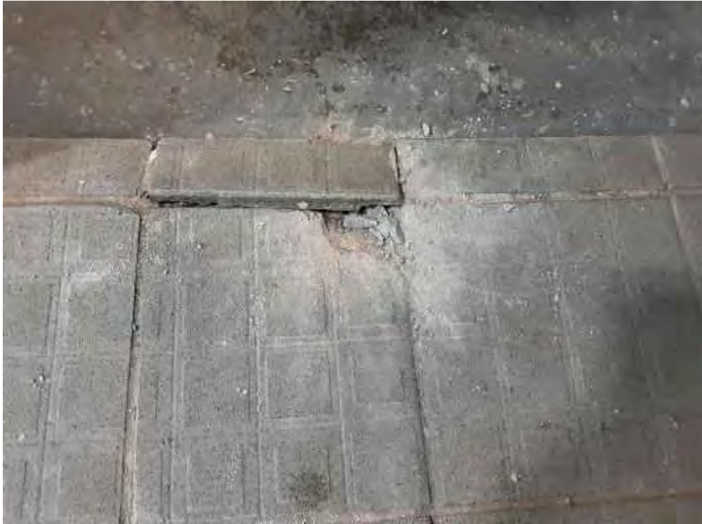
S0022A (None), Floor, All, Mortar, Indoor Pool (Location #: 13)
