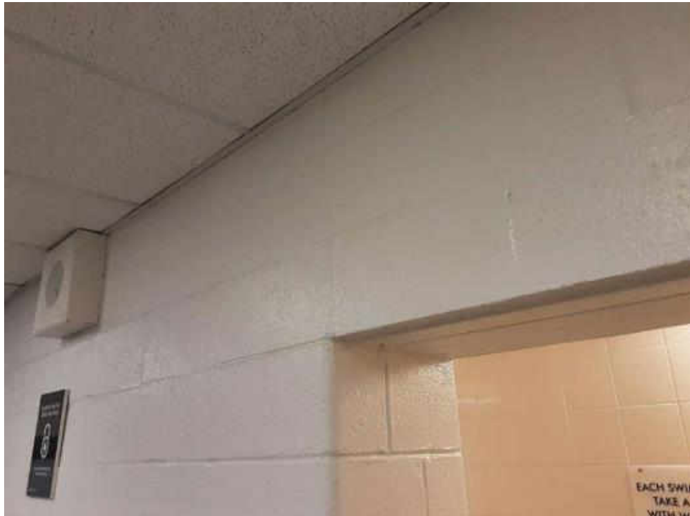
V0000 (None), Wall, All, Masonry, Men's Change Room (Location #: 9) Block wall
