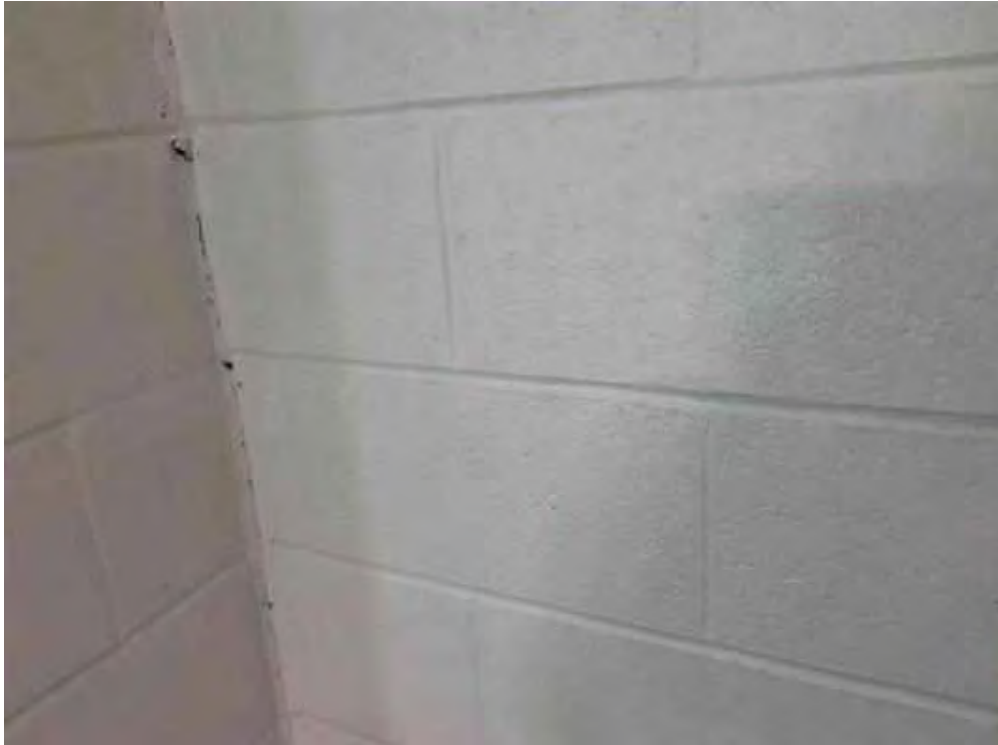
S0001D (None), Wall, All, Mortar, Balcony (Location #: 4) Block wall
