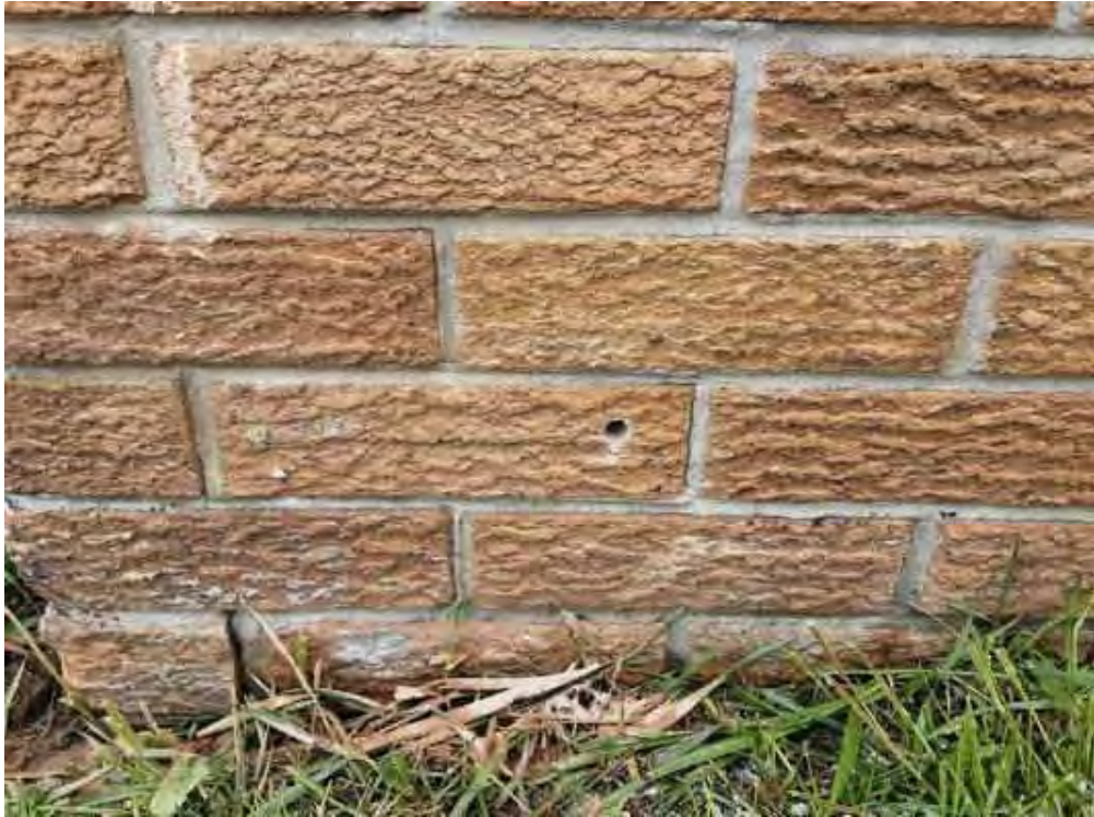
V0000 (None), Wall, Vermiculite, Exterior (Location #: 14) 5 Drill holes, no vermiculite, N wall, NE wall, S wall, SW wall, brick wall
