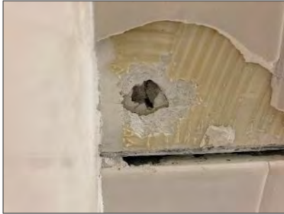
Photo 14: Non-asbestos plaster in the Men's Change Room (Loc. 9).
