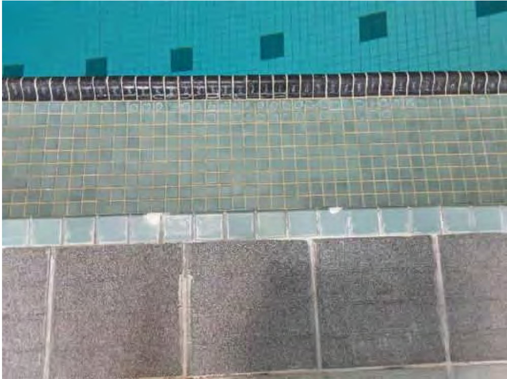
V0000 (None), Floor, Ceramic Tiles, Indoor Pool (Location # 13)
