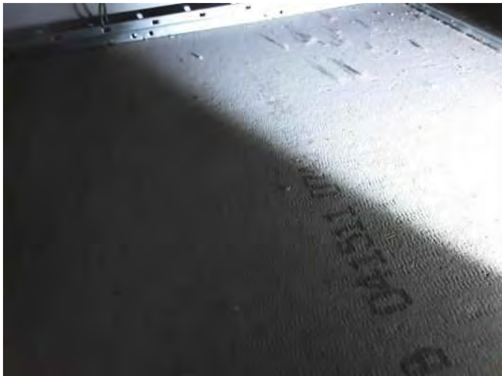
V0000 (None), Ceiling, All, Ceiling Tiles (lay-in), Lobby (Location #: 7) Date stamp- 04/15/11
