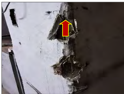
Photo 8: Fibreglass insulated air handling unit present in the Fan Room (Loc. 1).
