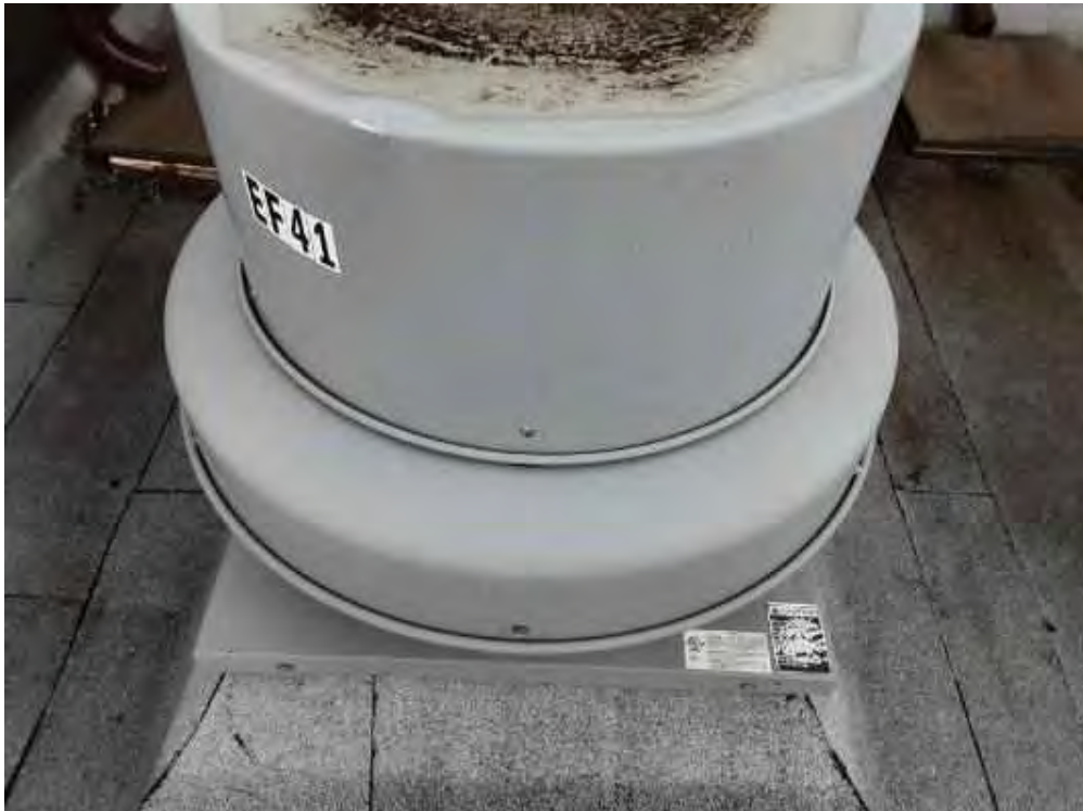
V0000 (None), Mechanical Equipment, Fan Unit, Not Insulated, Lower Roof (Location #: 17) Ventilator
