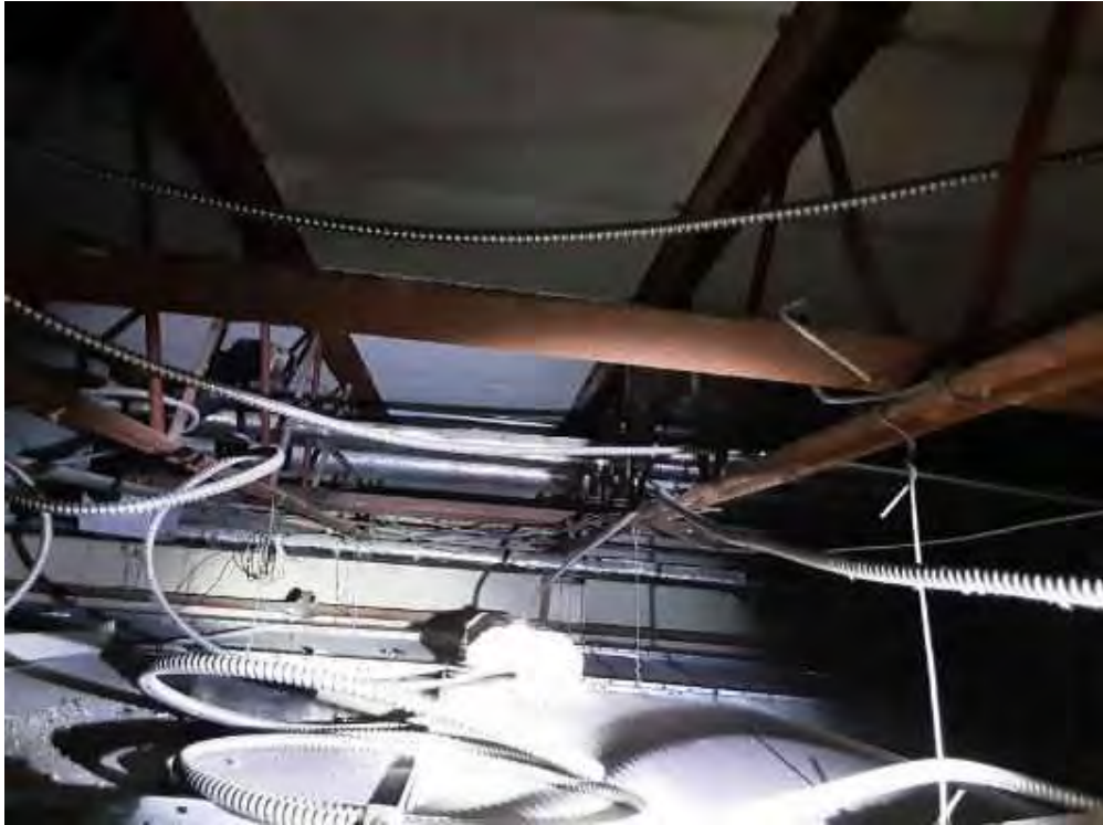
V0000 (None), Piping, All, Fibreglass, Women's Change Room (Location #: 12)
