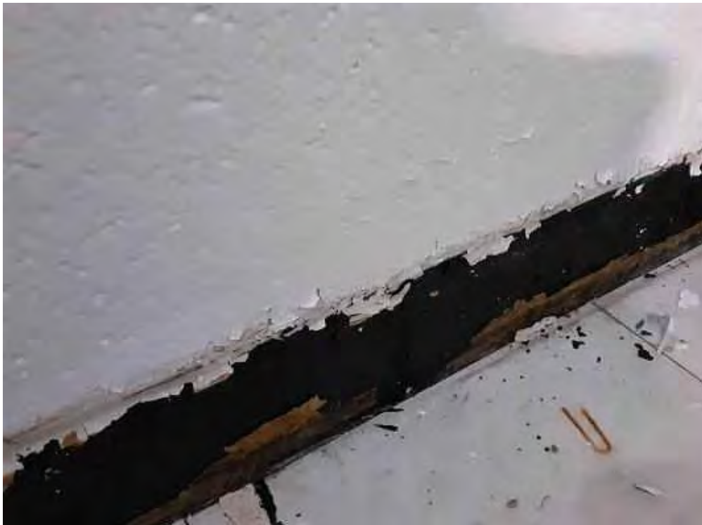
Concrete (poured), Black, L0011(Lead (High)), East Stairwell (Location #: 5)
