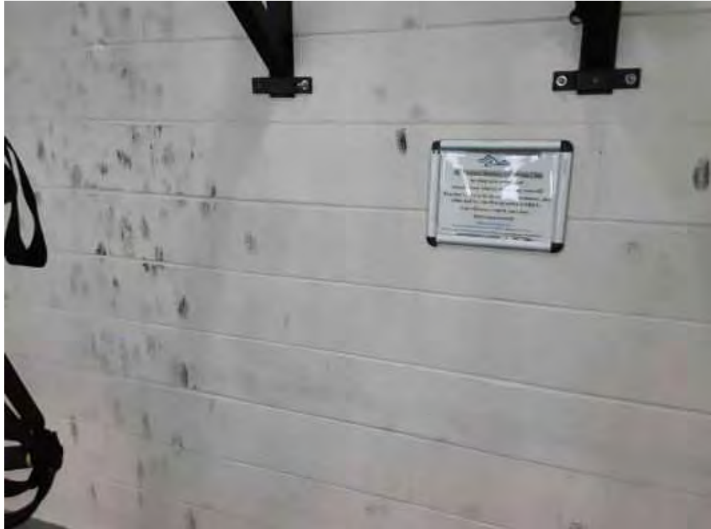
S0001C (None), Wall, All, Mortar, Balcony (Location #: 4) Block wall
