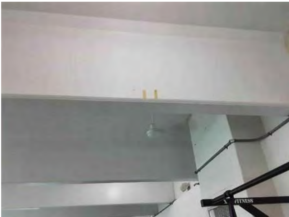
V0000 (None), Structure, All, Concrete (poured), Balcony (Location #: 4)
