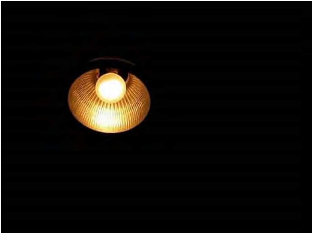
Mercury, Mechanical Room And Stairwell (Location #: 21)
