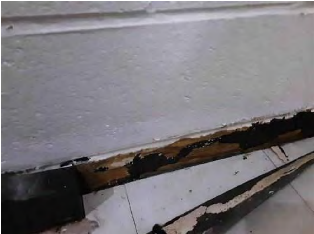
S0006A (None), Wall, Base, Mastic, Yellow, East Stairwell (Location #: 5)
