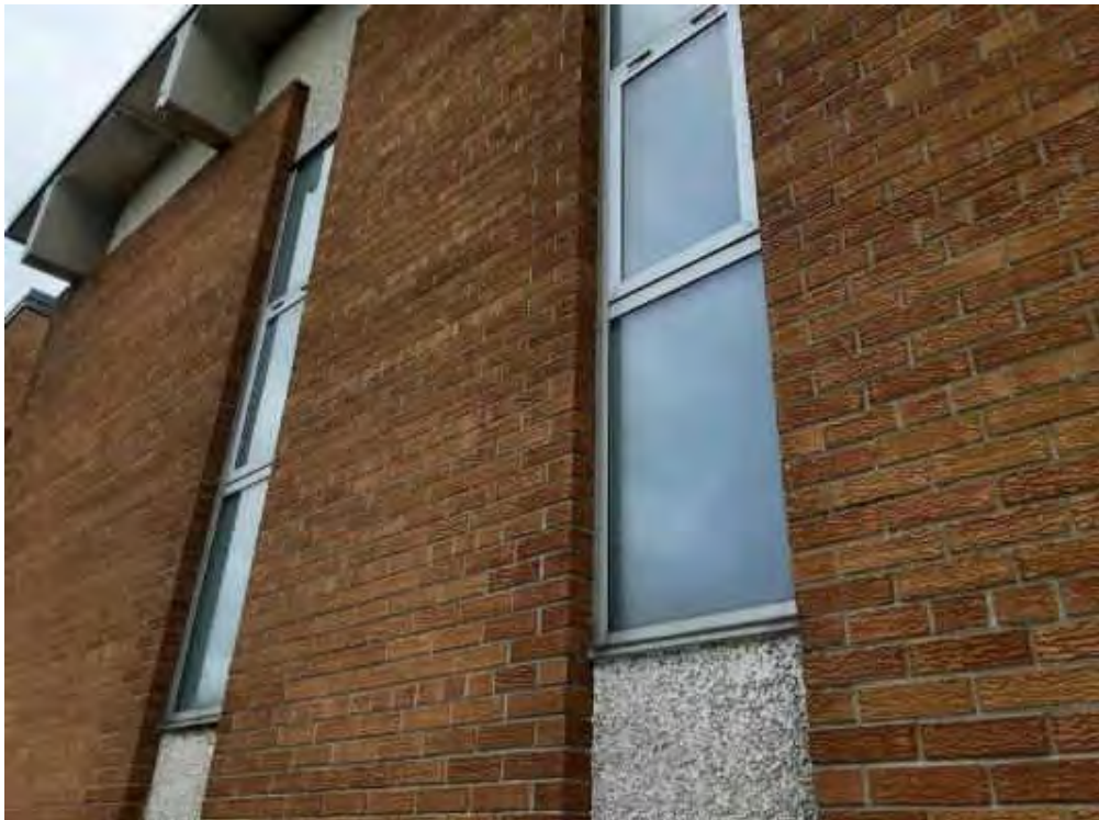
S0015C (None), Other, Window, Caulking, Exterior (Location #: 14) Light Grey, S wall
