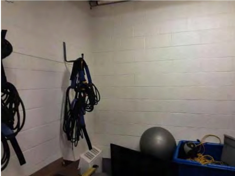
V0000 (None), Wall, All, Masonry, Equipment Room 2 (Location #: 20) Block wall
