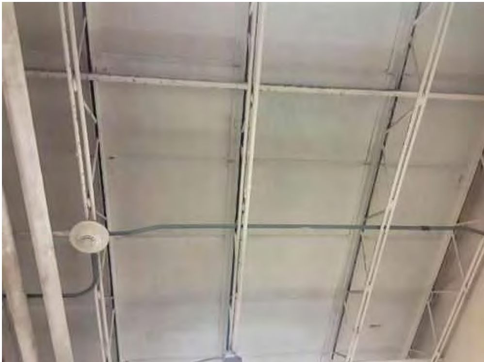
V0000 (None), Structure, All, Concrete (precast), Equipment Room 2 (Location #: 20)
