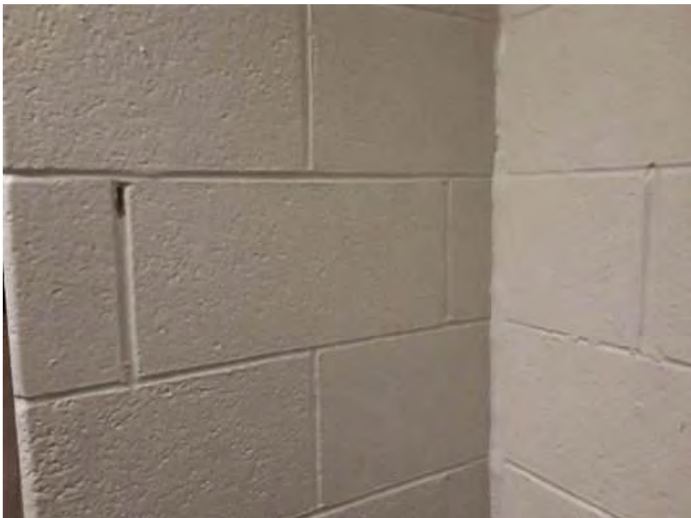
S0001E (None), Wall, All, Mortar, Men's Change Room (Location #: 9) Block wall
