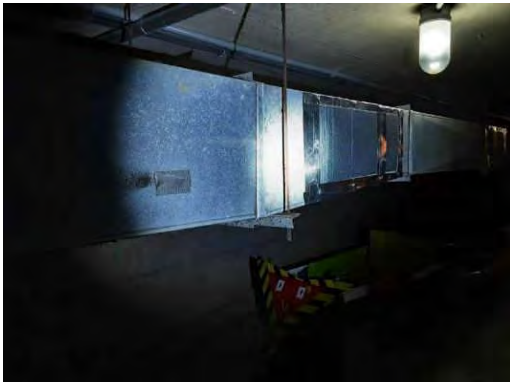
V0000 (None), Duct, All, Not Insulated, Tunnel Area (Location #: 3)
