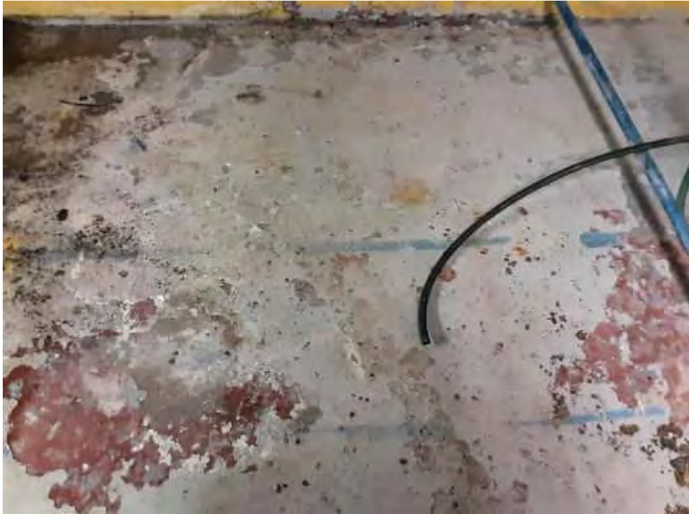
Concrete (poured), Grey, V0001(Lead (Low)), Filter Room (Location #: 2)
