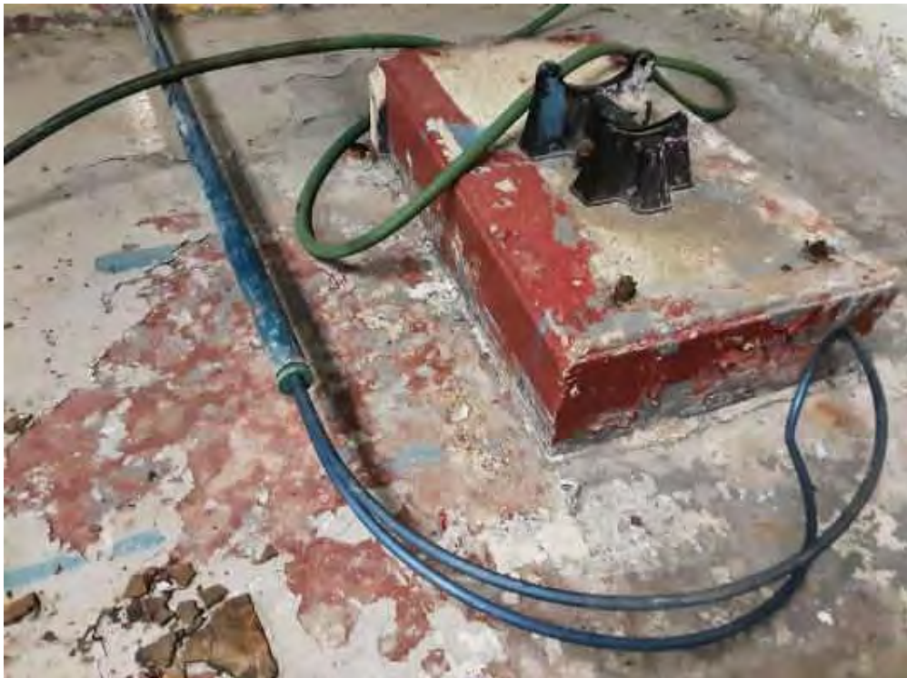
Concrete (poured), Red, L0003(Lead (High)), Filter Room (Location #: 2)
