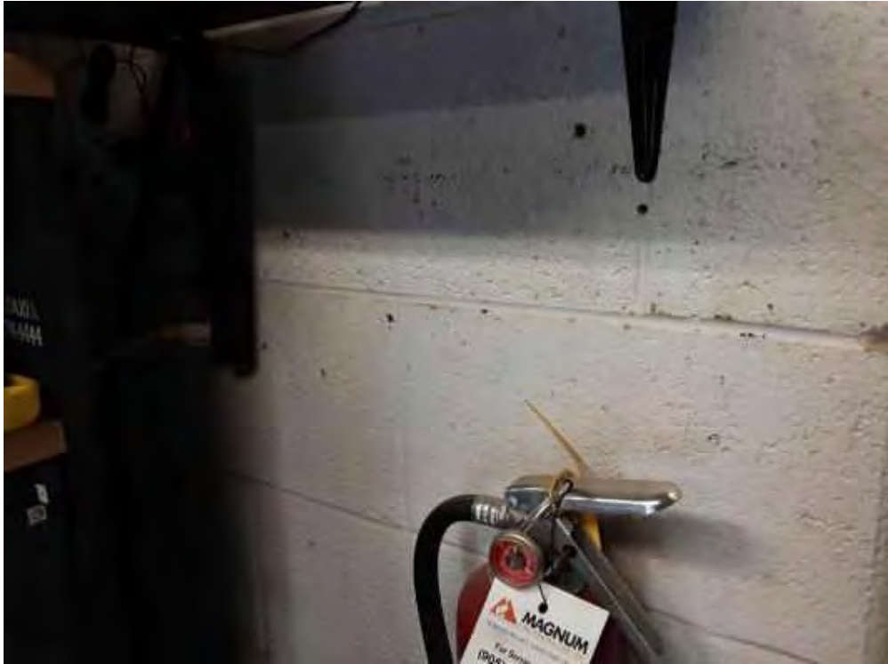
S0028C (Confirmed Asbestos), Wall, All, Mortar, Custodian (Location #: 29) Block wall
