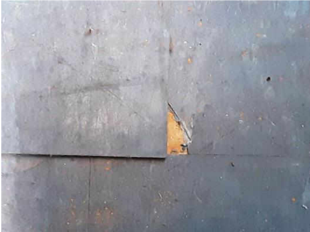
S0020C (None), Floor, Vinyl Floor Tile and Mastic, Equipment Storage (Location #: 16) Yellow mastic
