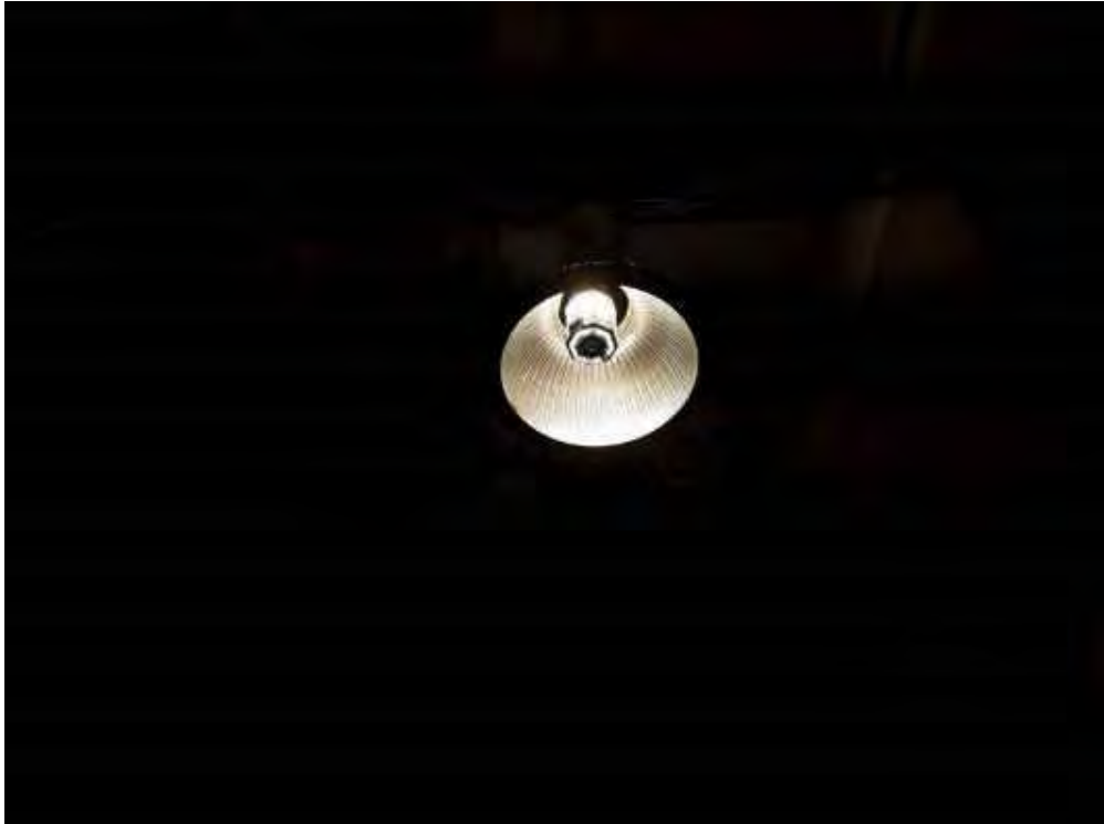
Mercury, Mechanical Room And Stairwell (Location #: 21)
