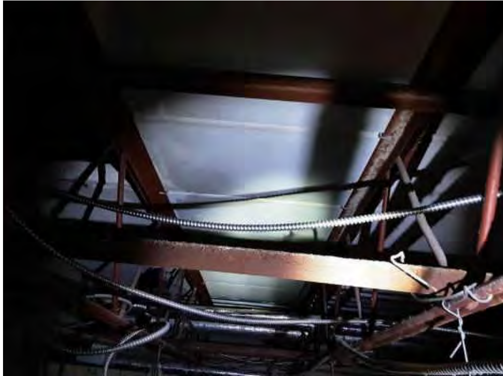
V0000 (None), Structure, All, Concrete (precast), Women's Change Room (Location #: 12)
