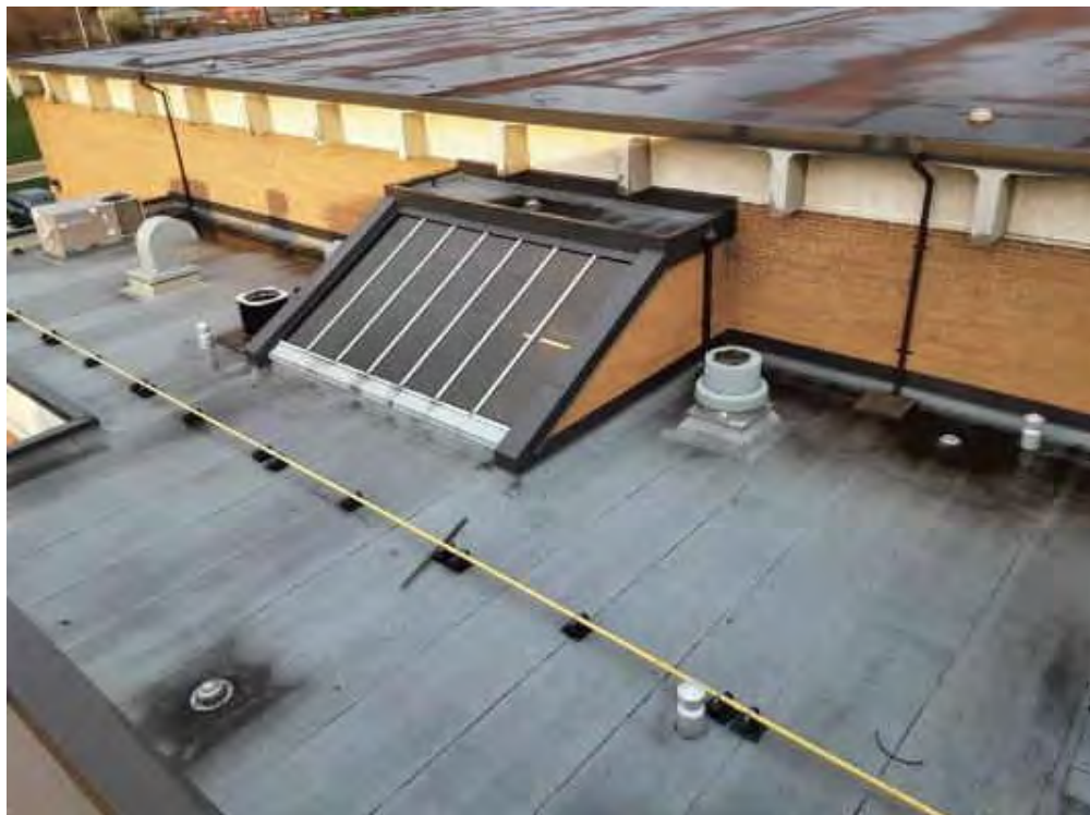
Lower Roof (Location #: 17)
