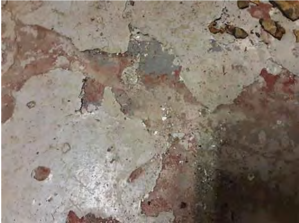
Concrete (poured), Light Grey, L0002(Lead (Low)), Filter Room (Location #: 2)
