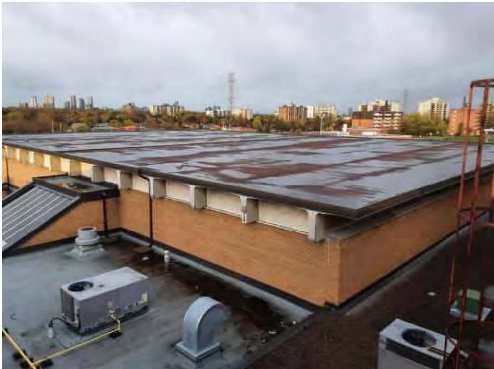
Pool roof (Location #: 18)
