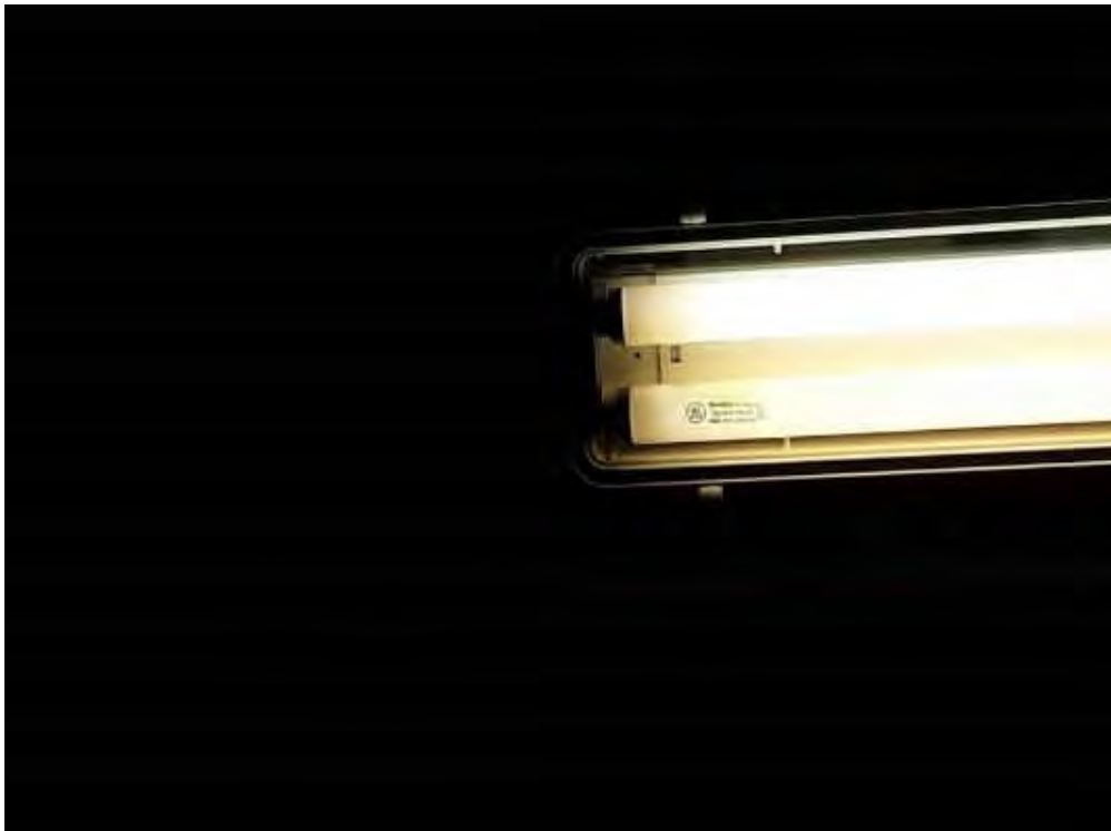
Mercury, Equipment Room 2 (Location #: 20)
