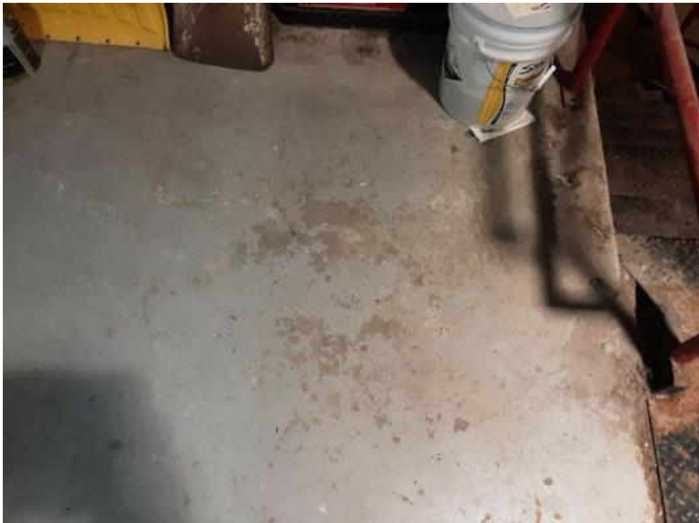
Concrete (poured), Grey, V0001(Lead (Low)), Mechanical Room And Stairwell (Location #: 21)
