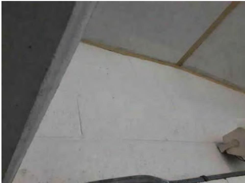
PCB, Balcony (Location #: 4)
