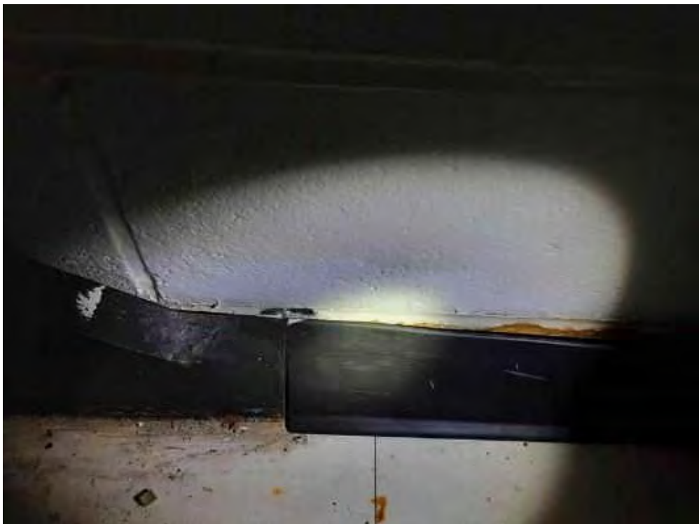
V0000 (None), Floor, Base, Rubber, East Stairwell (Location #: 5)
