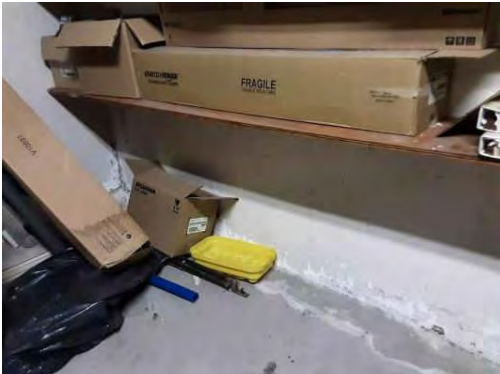
V0000 (None), Wall, All, Concrete (poured), Fan Room (Location #: 1)
