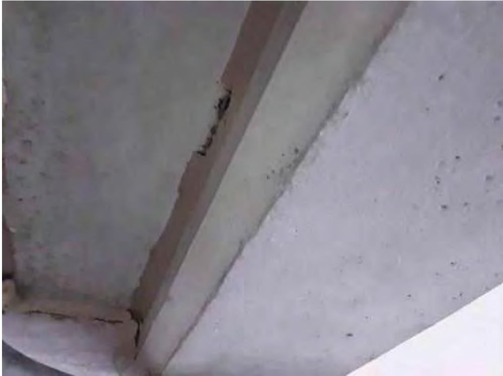
PCB, Balcony (Location #: 4)
