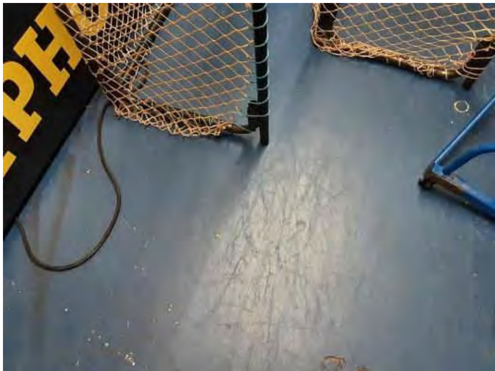
V0000 (None), Floor, All, Concrete (poured), Gym Storage (Location #: 25)
