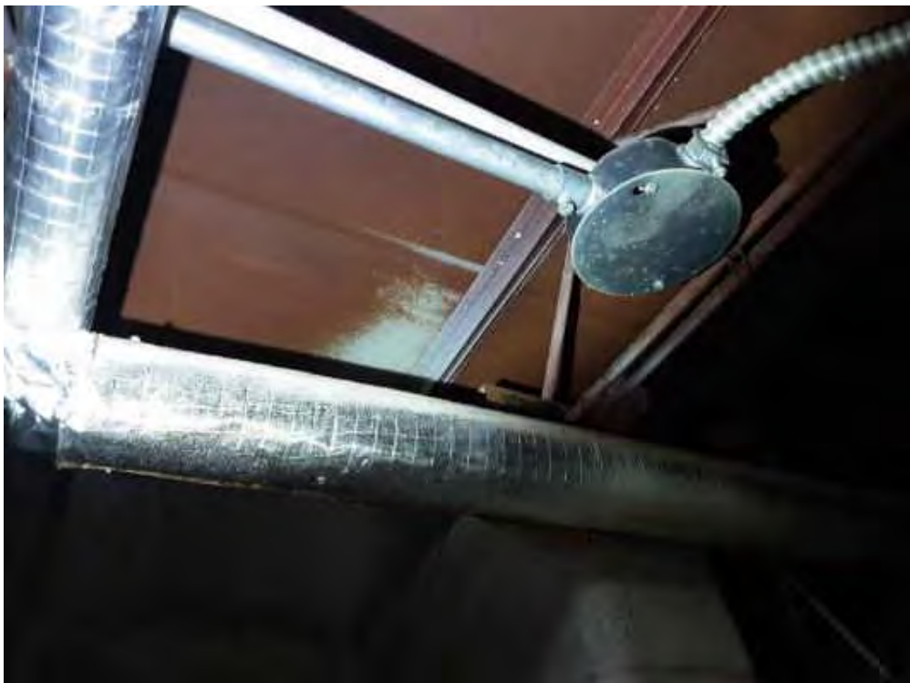
V0000 (Non e), Structure, Deck, Metal, Men's Washroom (Location # 22)
