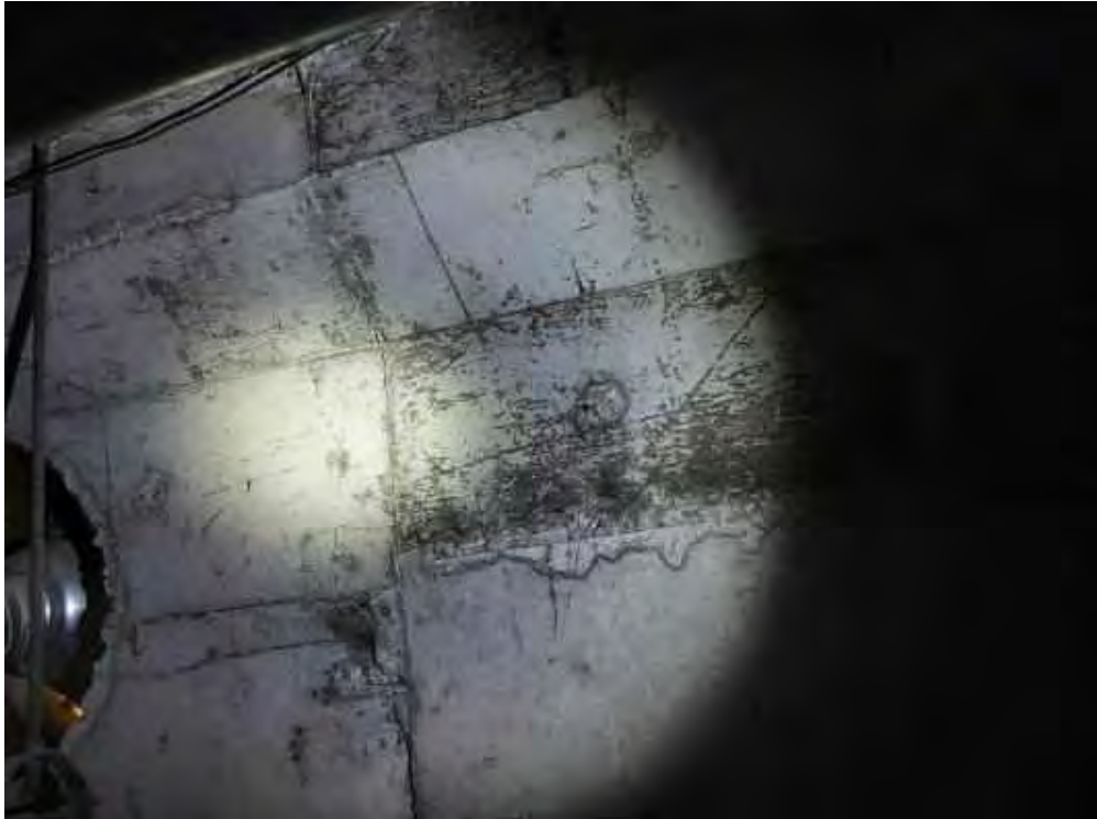
V0000 (None), Wall, All, Concrete (poured), Tunnel Area (Location #: 3)
