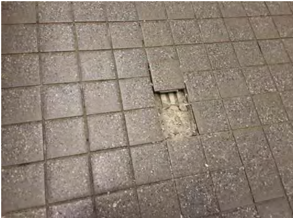
S0009B (None), Floor, All, Mortar, Pool Office (Location #: 8)
