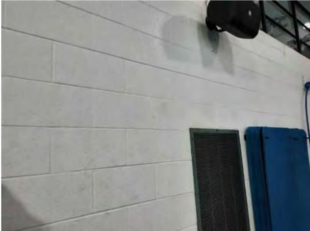
V0000 (None), Wall, All, Masonry, Indoor Pool (Location #: 13) Block wall
