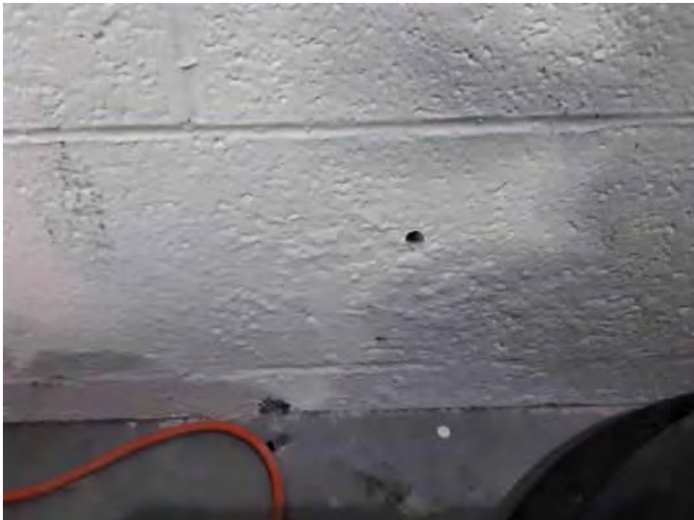
V0000 (Non e), Wall, Vermiculite/concrete block walls, Balcony (Location #: 4) 2 Drill holes, no vermiculite
