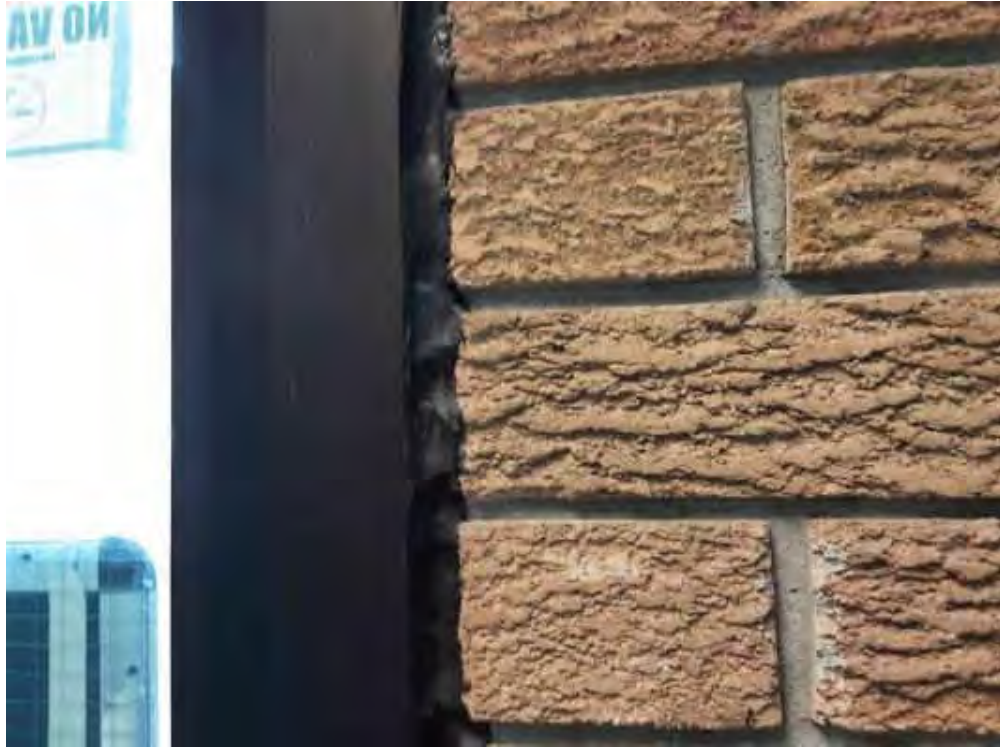
PCB, Entrance Vestibule (Location #: 6)
