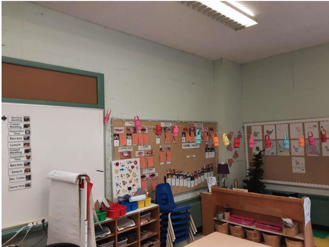
S0035C (None), Blue paint on block wall in Location #: 7
