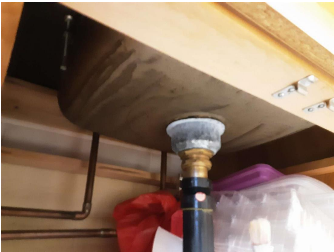
S0032C (Confirmed Asbestos), Sink mastic on sink bottom in Work Room (Location #: 38) Located on the underside of the sink
