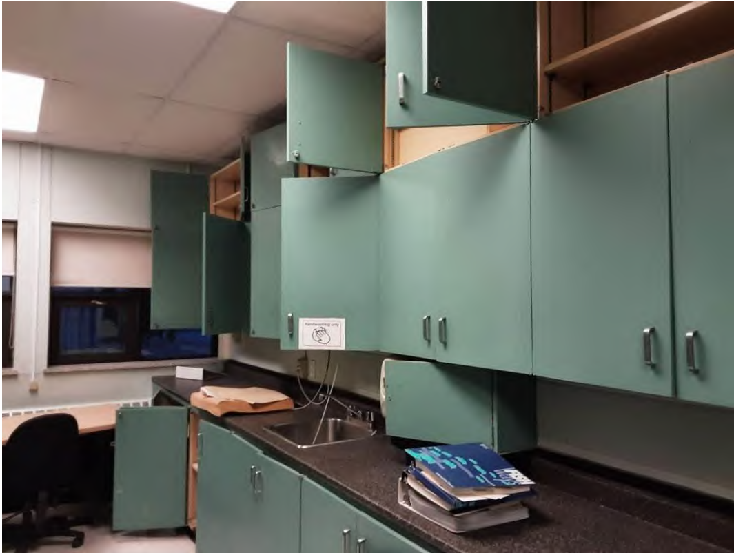
L0016(Lead, High), Green paint on cupboards in the Prep Room (Location #: 21)
