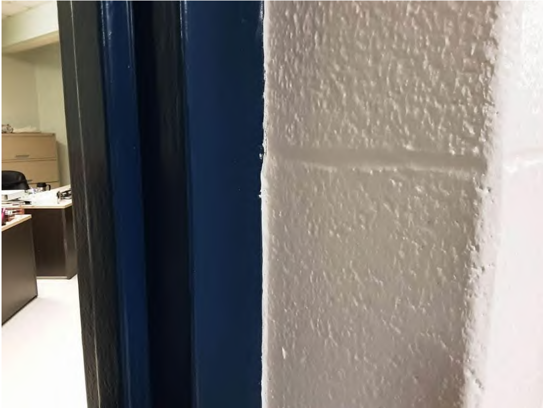
S0057C (None), Grey caulking around door frame in the Corridor (Location #: 125)
