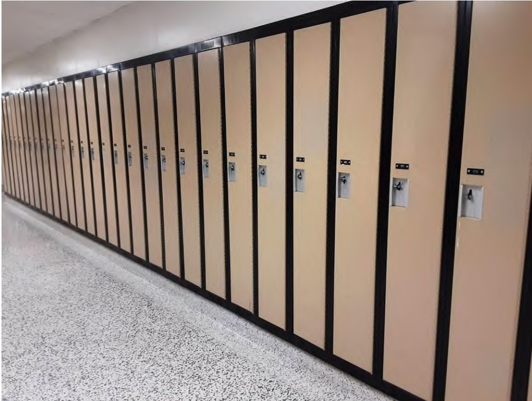
V9500(Presumed Lead), Beige paint on lockers in the Corridor (Location #: 89)
