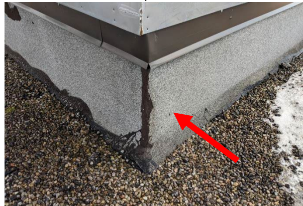
Samples 17A-C: non-asbestos asphalt sheeting, HVAC footings, East Roof
