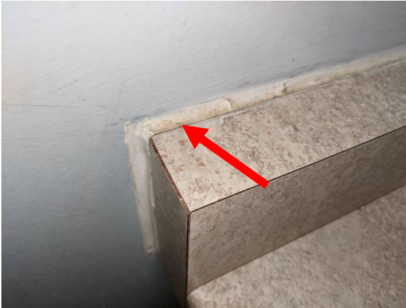
Samples 12A-C: non-asbestos white interior caulking, Second Floor Washrooms, Ground Floor Washrooms, and Ground Floor Kitchen
