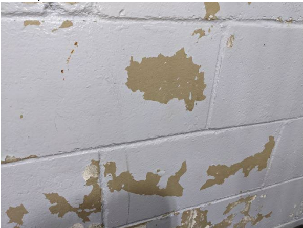
Sample LP6: lead-containing multilayered light blue-grey paint, Arena
