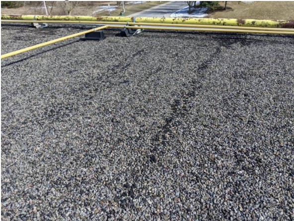
Samples 20A-C: non-asbestos built up roof matrix, East Roof
