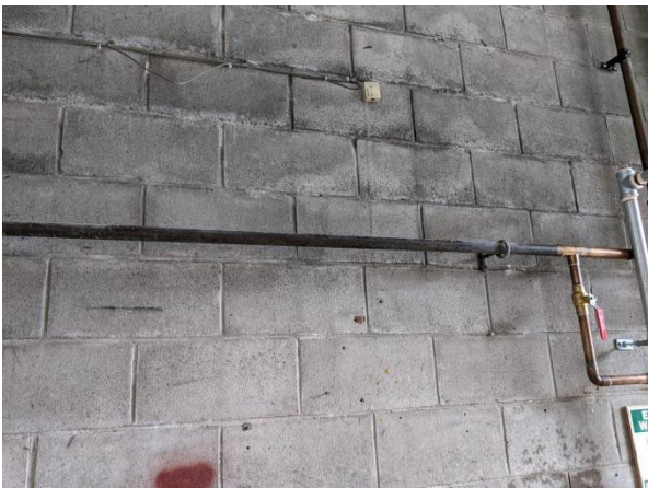
Samples 10A-C: non-asbestos concrete block mortar, 1977 build
