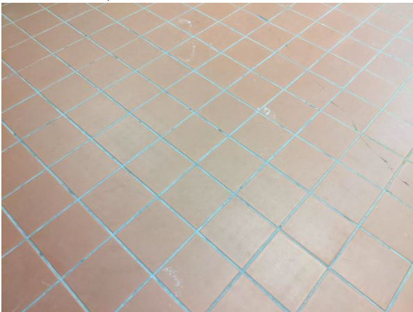
Samples 4A-C: non-asbestos terracotta tile grout, Stairwell/ Arena Vestibule
