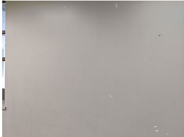
Sample LP1: non-lead dark blue-grey wall paint, throughout Second Floor
