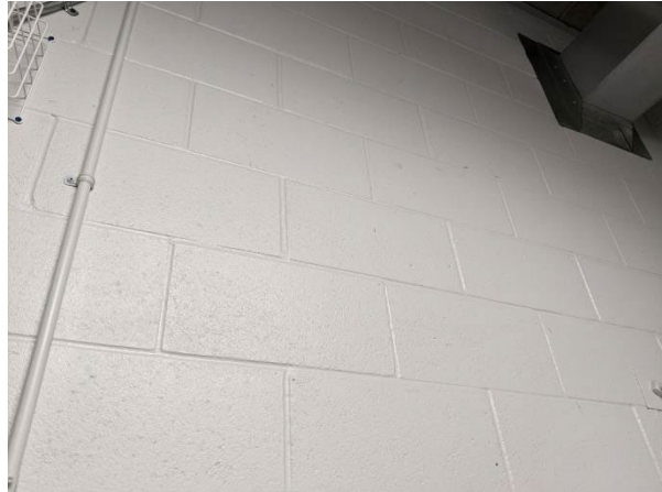
Sample LP5: non-lead light grey paint, Mechanical Room
