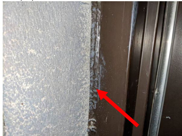
Samples 15A-C: asbestos-containing grey caulking (some sections painted brown), Ground Floor interior door and window frames, 1977 build
