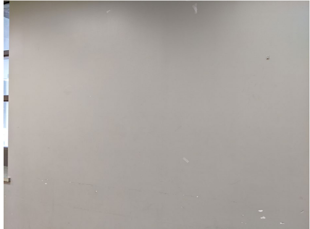
Samples 1A-G: non-asbestos drywall joint compound, throughout 1977 build
