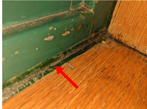
Samples 13A-C: non-asbestos green interior caulking, around wood window frames, Second Floor Multipurpose Room
