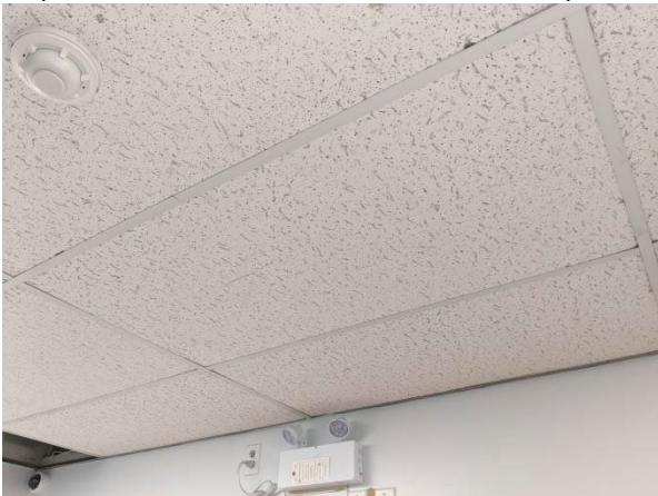
Samples 8A-C: non-asbestos acoustic ceiling tile, Second Floor Stairwell
