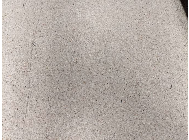
Samples 7A-C: non-asbestos brown pebbled vinyl sheet flooring, Ground Floor Kitchen
