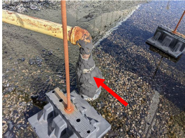
Samples 19A-C: non-asbestos tar sealant, roof penetrations, East and West Roofs
