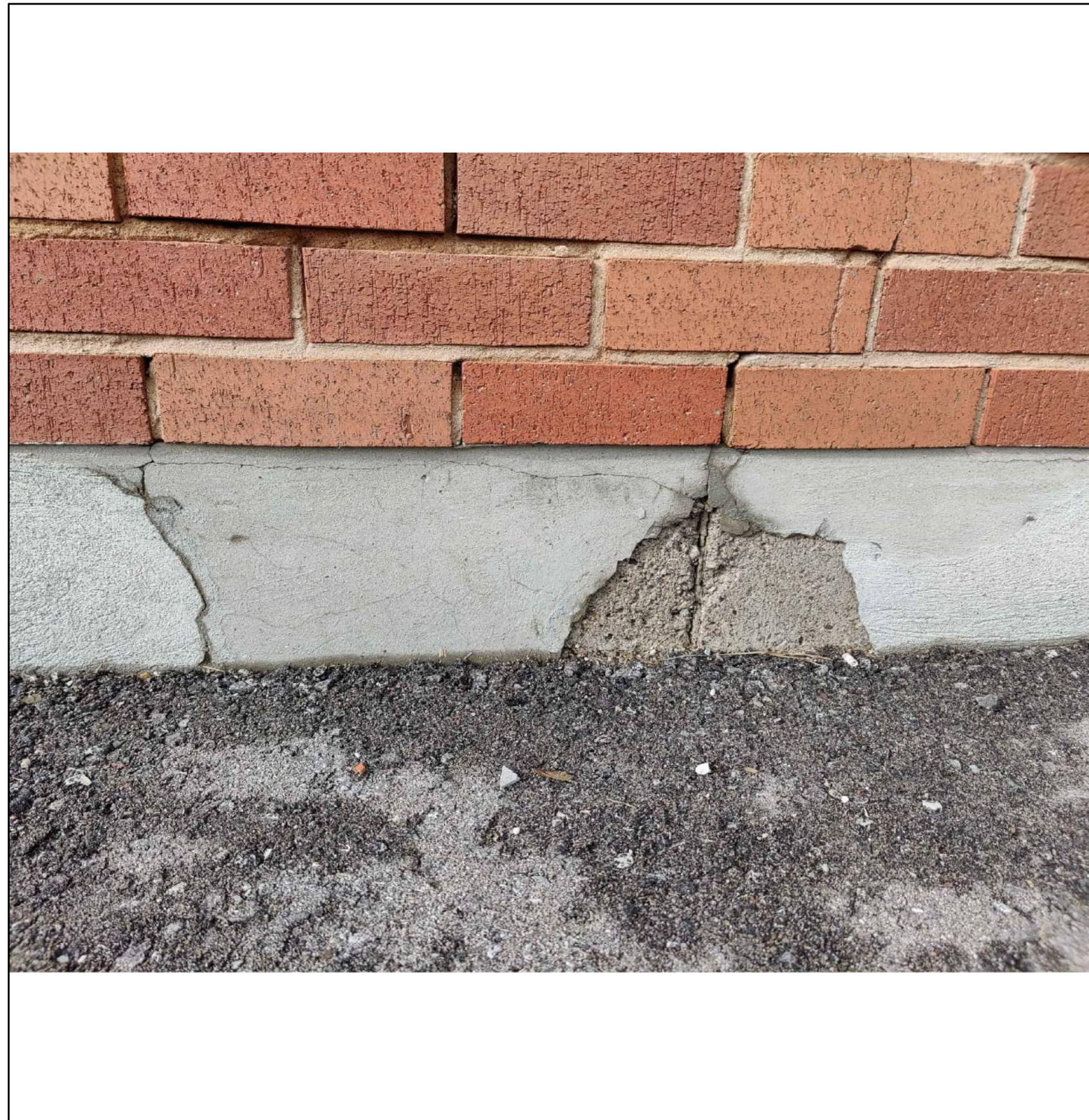
4 TYPICAL PARGING REPAIR R600
