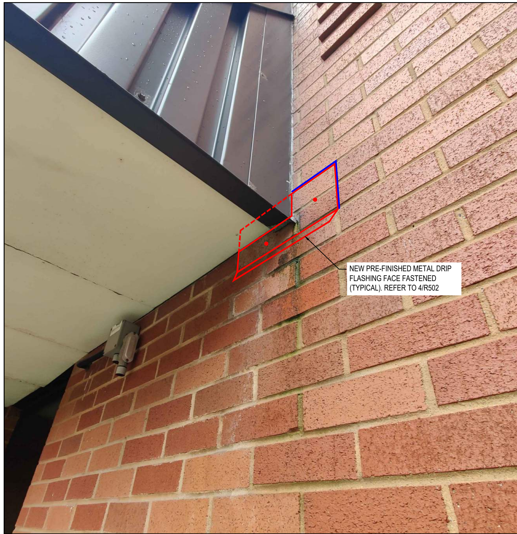
1 COURTYARD CORNER FLASHING R501
