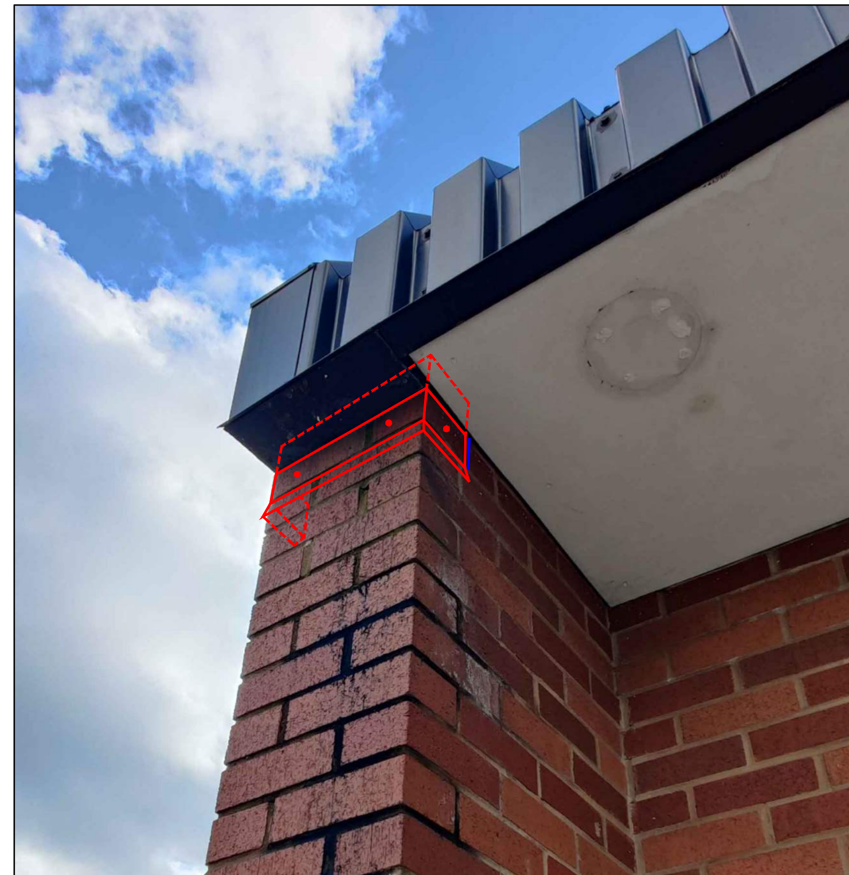
5 SOUTH-EAST CORNER FLASHING R501
