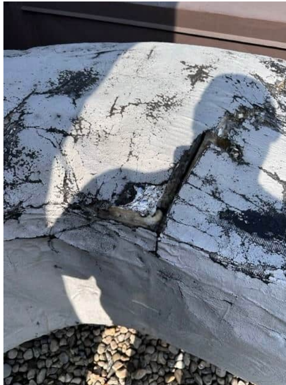
Photograph No. 22 – 115 Delhi Street – Roof - September 23, 2023. Exterior duct cladding confirmed as non-asbestos-containing (S04A, B, C).
