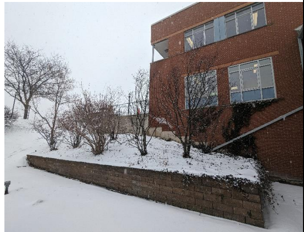
East patio retaining wall.
