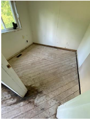
Post abatement (abated VFT) view, Location 10.
