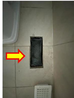
Post abatement (abated fiberboard insulation) view, Location 8.
