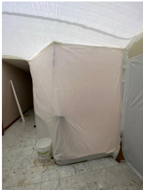
General view within enclosure, Location 8.
