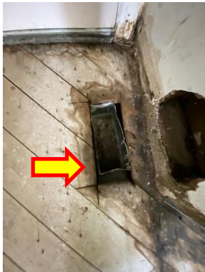
Post abatement (abated fiberboard insulation) view, Location 9.
