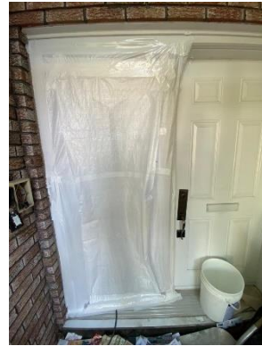
Enclosure entrance, Location 8
