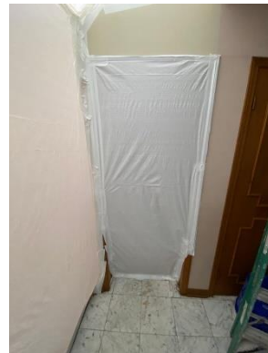
General view within enclosure, Location 8.
