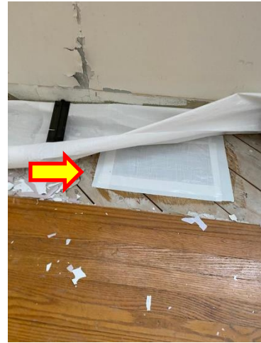
View of floor registers covered with poly.
