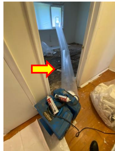
View of negative air unit venting outside of the building.
