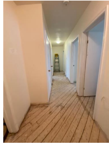
Abated asbestos-containing paper insulation and original hardwood flooring, Corridor, Location 17.
