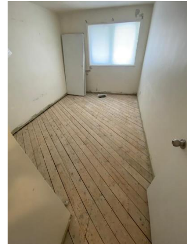
Abated asbestos-containing paper insulation and original hardwood flooring, Bedroom, Location 14.
