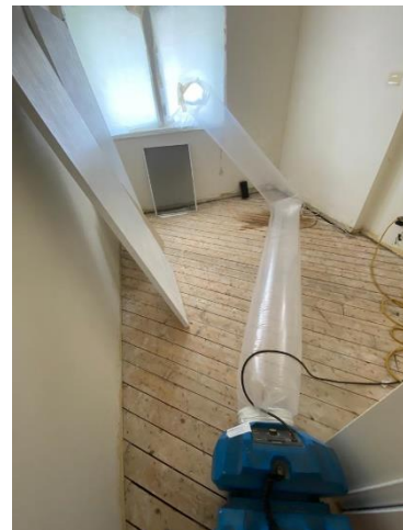
Abated asbestos-containing paper insulation and original hardwood flooring, Bedroom, Location 16.
