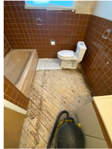
Abated asbestos-containing paper insulation and original hardwood flooring, Bathroom, Location 11.
