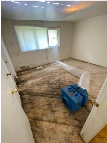
Abated asbestos-containing paper insulation and original hardwood flooring, Bedroom, Location 13.
