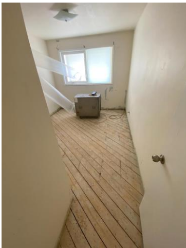
Abated asbestos-containing paper insulation and original hardwood flooring, Bedroom, Location 15.
