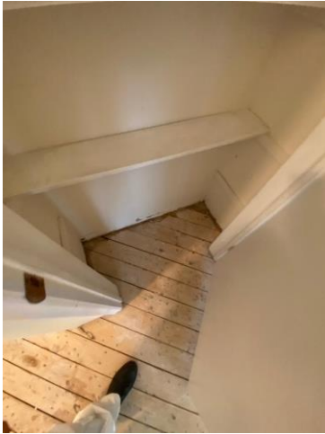
Abated asbestos-containing paper insulation and original hardwood flooring, Corridor's Closet, Location 17.
