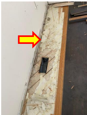
White paper insulation found under original hardwood flooring, Location 14.
