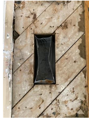
Post abatement (abated fiberboard insulation) view, Floor Register.
