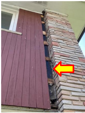
Post abatement (abated caulking) view, Wood Siding, Exterior.
