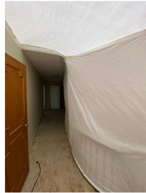
General view within enclosure, Location 8.
