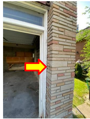
Post abatement (abated caulking) view, Garage Door, Exterior.
