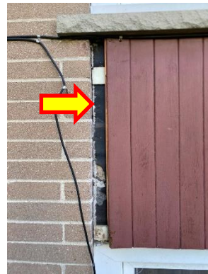
Black paper insulation behind wood siding, Exterior.
