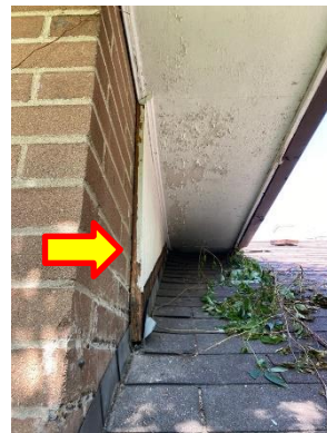
Post abatement (abated caulking) view, Roof Flashing, Exterior.
