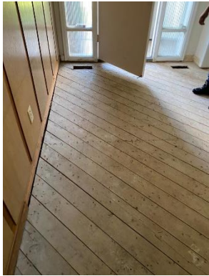
Post abatement (abated VFT) view, Location 4.
