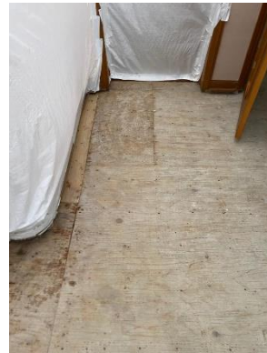
Post abatement view, Location 8
