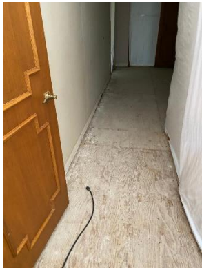
Post abatement view, Location 8
