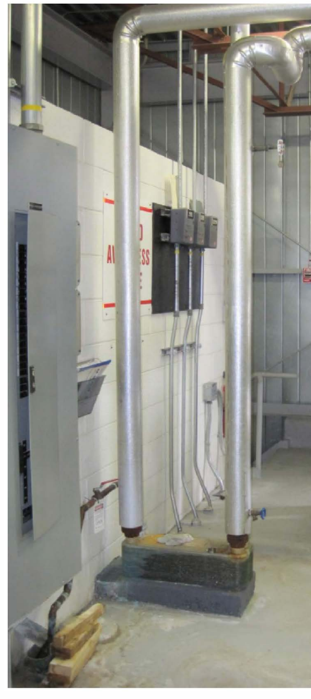
PHOTO 1: EXISTING HX-1 ON CONCRETE PAD (REFER TO DRAWING 404 FOR SYSTEM LOCATION)
