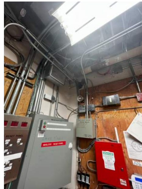
EXISTING CONDITION PHOTO - ECP13
