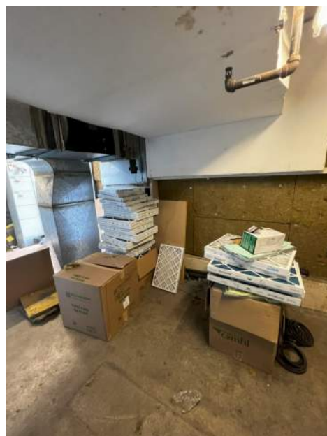
EXISTING CONDITION PHOTO - ECP6
