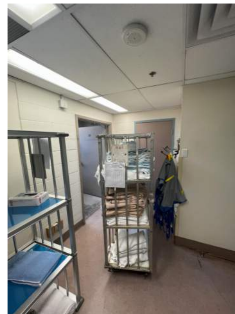
EXISTING CONDITION PHOTO - ECP14
