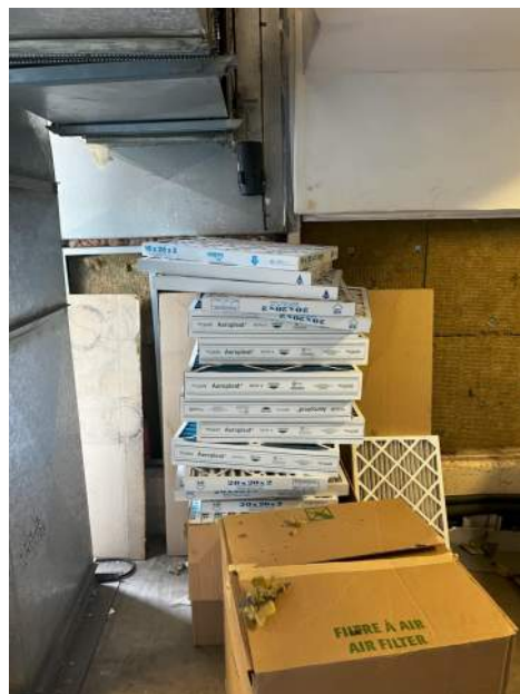
EXISTING CONDITION PHOTO - ECP3
