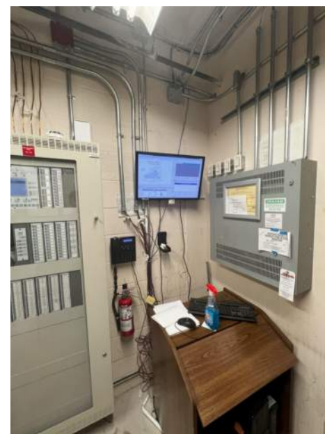
EXISTING CONDITION PHOTO - ECP15
