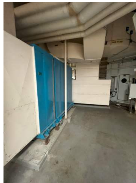
EXISTING CONDITION PHOTO - ECP11
