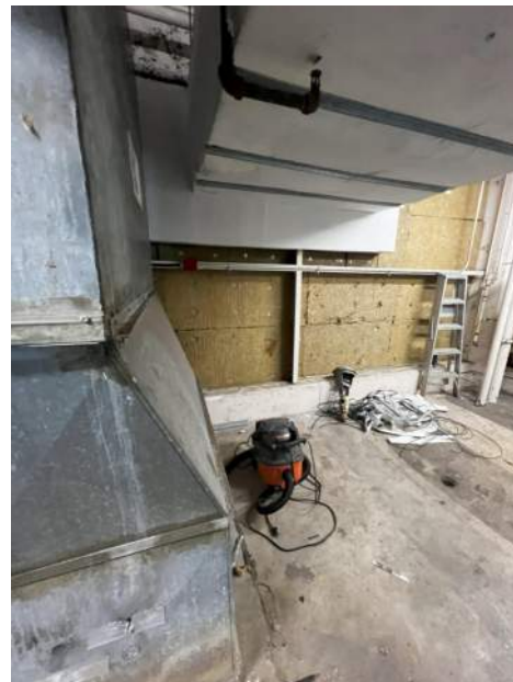
EXISTING CONDITION PHOTO - ECP7
