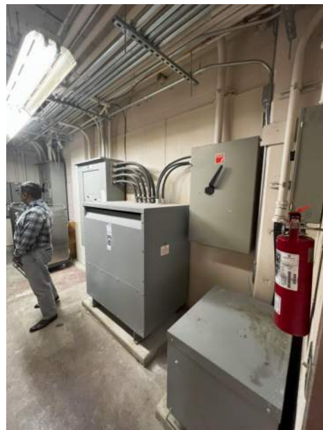
EXISTING CONDITION PHOTO - ECP4
