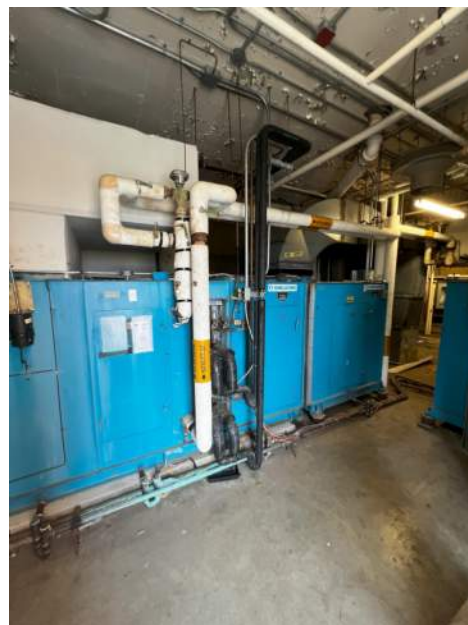
EXISTING CONDITION PHOTO - ECP8
