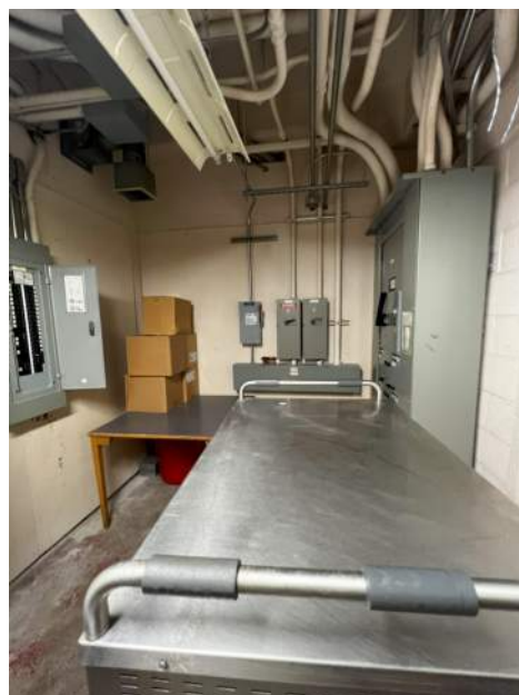
EXISTING CONDITION PHOTO - ECP2
