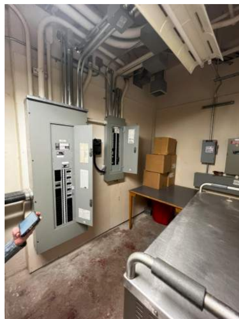
EXISTING CONDITION PHOTO - ECP5
