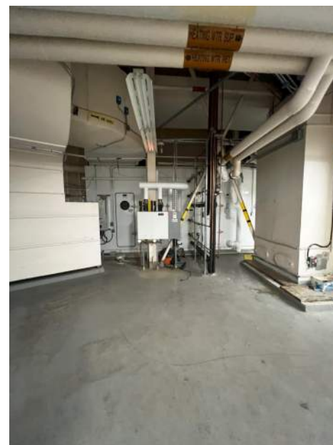
EXISTING CONDITION PHOTO - ECP12
