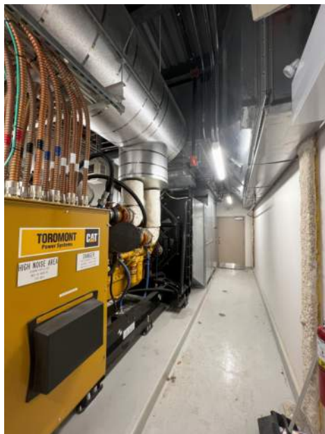
EXISTING CONDITION PHOTO - ECP1
