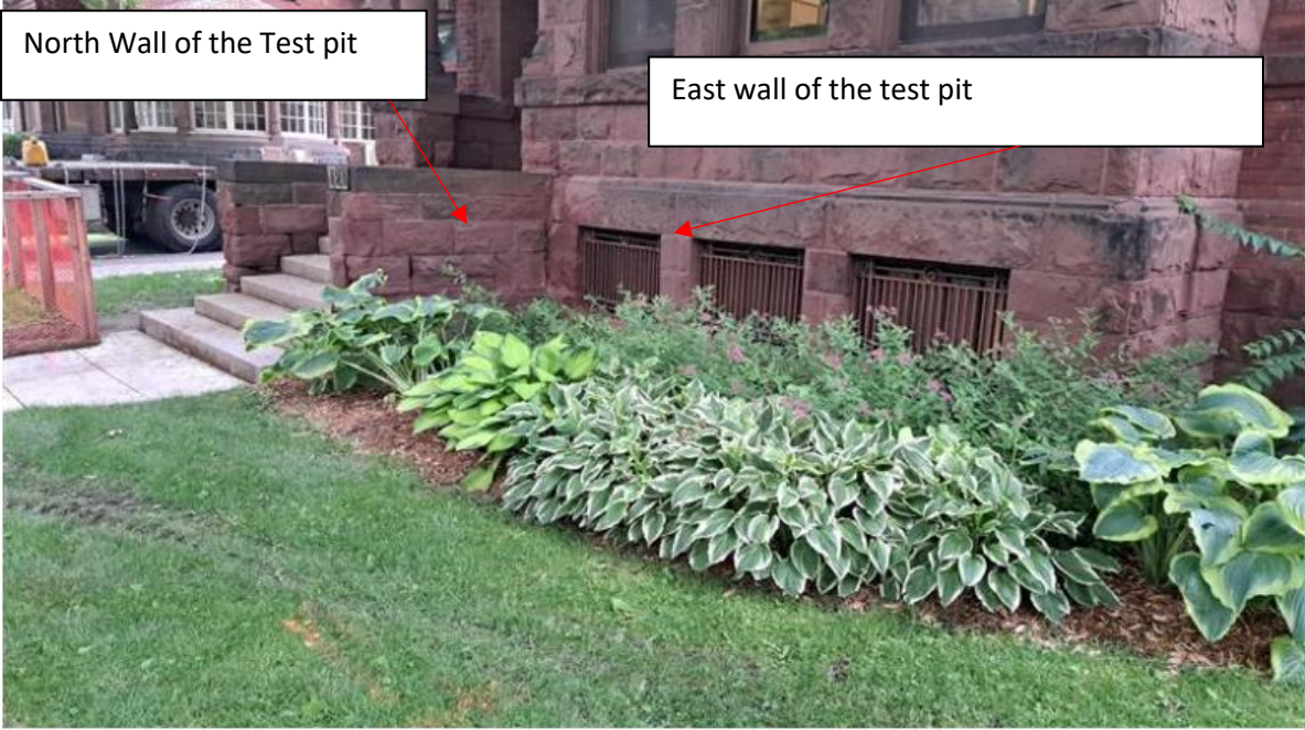
Photo 1 – Test Pit Location
