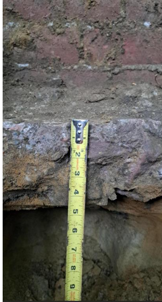
Photo 3: Thickness of the stone footing (115 mm)
