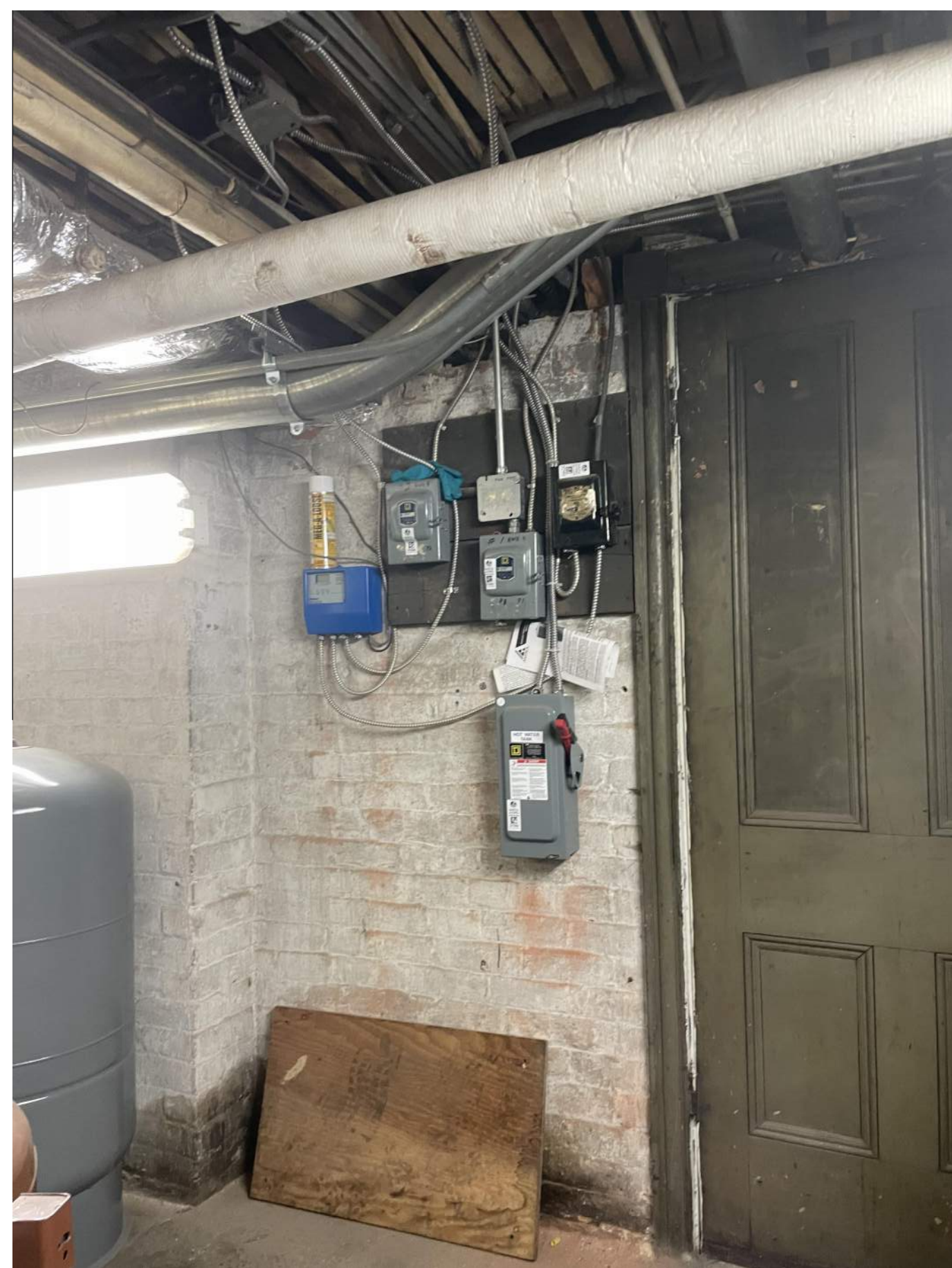
6 WALL MOUNTED DISCONNECT SWITCHES SCALE:N.T.S.
