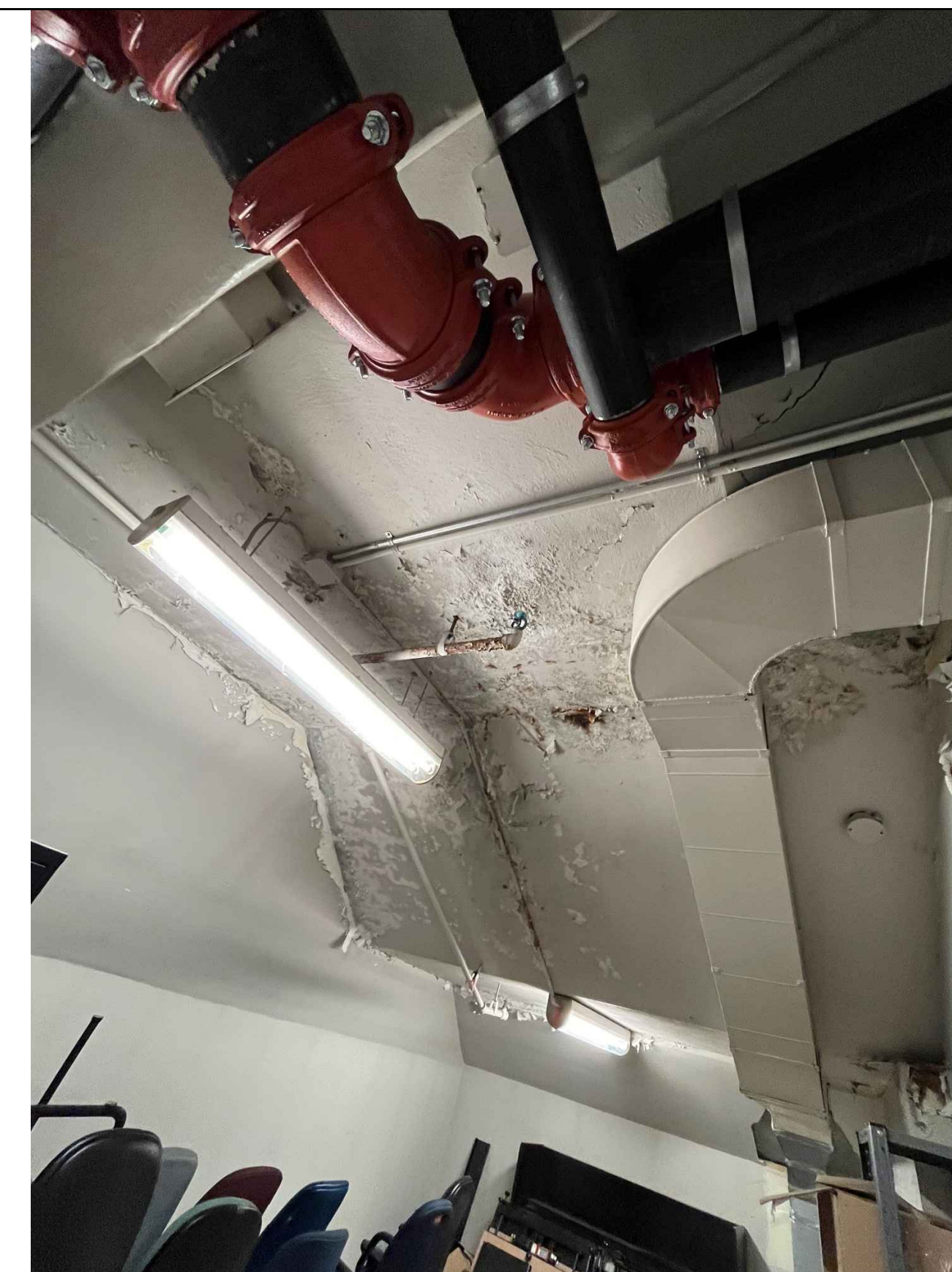
3 VIEW OF CONCRETE SOFFIT IN MECHANICAL ROOM R600
