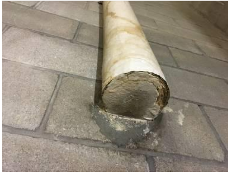
Hose Room - Piping Elbows and Piping T & End Joints Canvas Wrapped Applied White, Cementitious Insulations Not Asbestos Containing
