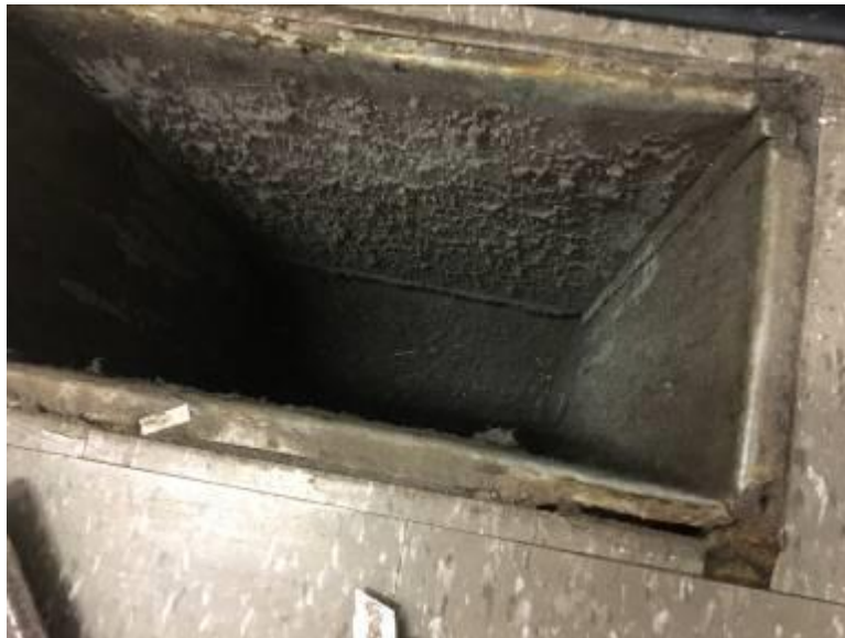
Main Floor Kitchen/Lounge/Sleeping Areas – 12” x 12” Vinyl Floor Tiles Beige White Flecked and Black Mastic Material Not Asbestos Containing
