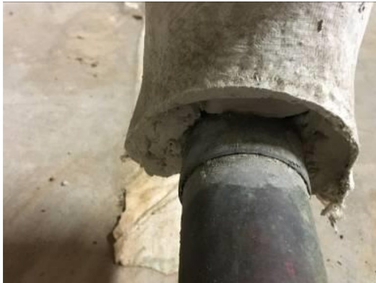
Hose Room - Piping Elbows and Piping T & End Joints Canvas Wrapped Applied White, Cementitious Insulations Not Asbestos Containing
