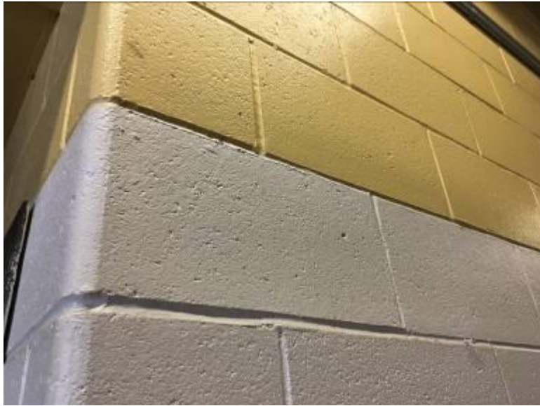
Main Floor – Painted Block Wall – White and Yellow
