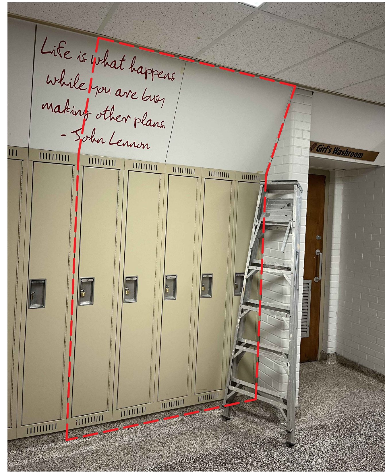
2 HALLWAY INTO EX. GIRLS BATHROOM A006 BROCK HS
