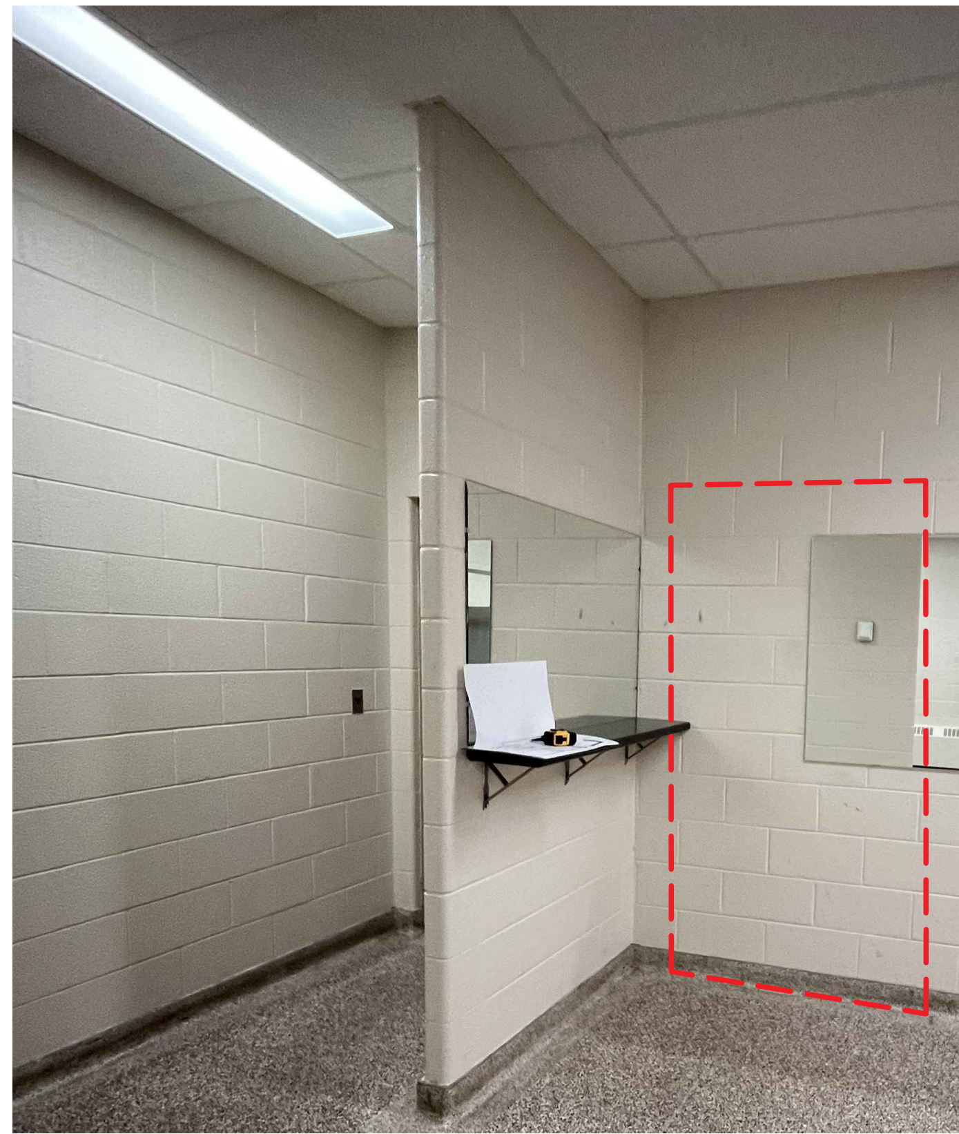
4 EXISTING GIRLS BATHROOM A006 BROCK HS
