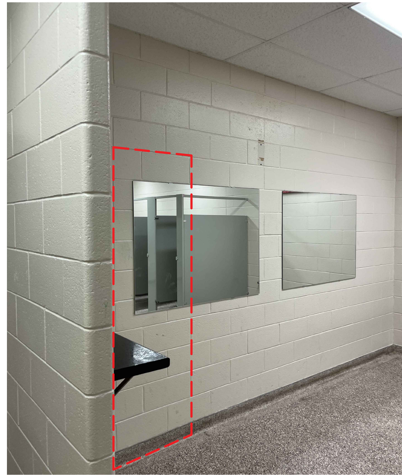
3 EXISTING GIRLS BATHROOM A006 BROCK HS
