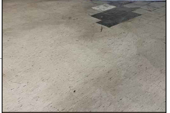
INSTALL NEW FLOOR AS SPECIFIED. INCLUDING EAST/WEST STAIRCASE (2 LOCATIONS). REFER TO ITEM 4 IN SCHEDULE.
