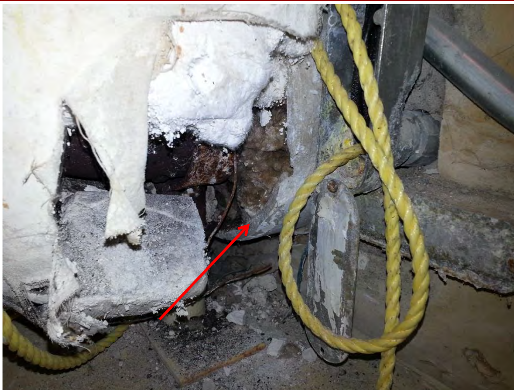
1 – View of asbestos containing Transite Pipe exiting the building
