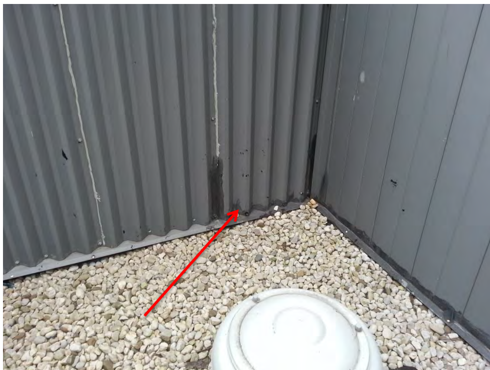
2 – View of asbestos black sealant on roof.
