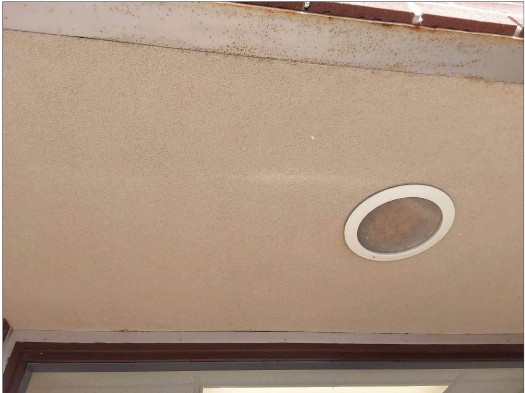
S0070C (None), Ceiling, Texture Coat, Exterior Wall For Renovation (Location #: 81) On soffit above door
