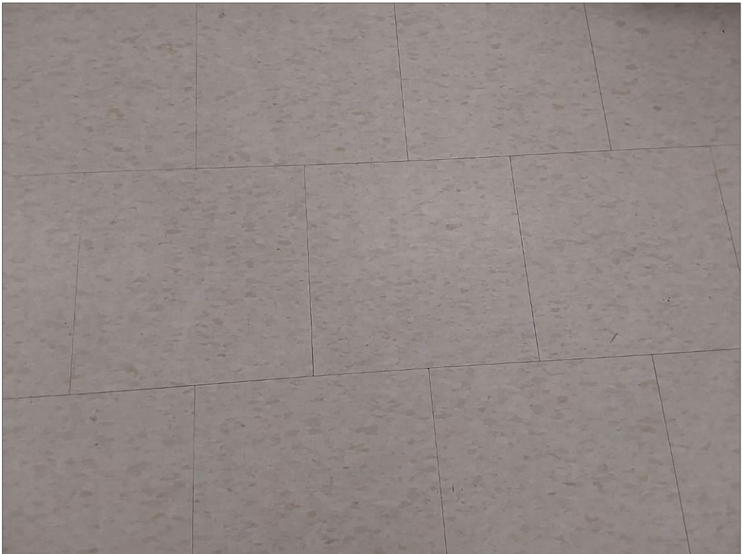
S0081C (None), 12" x 12" white with grey splotch, Floor, Vinyl Floor Tile and Mastic, Classroom (Location #: 40)
