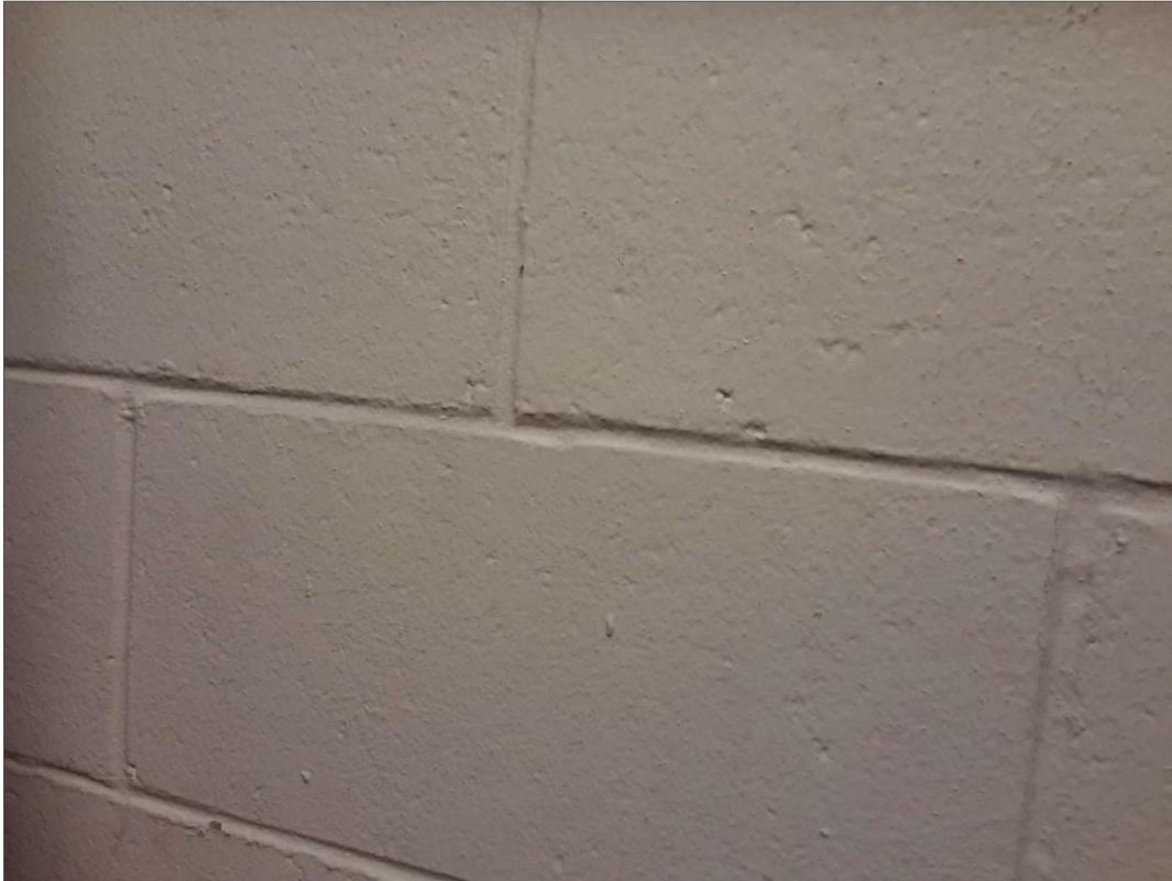
L0015(Lead, Low), White, Wall, Storage (Location #: 19)
