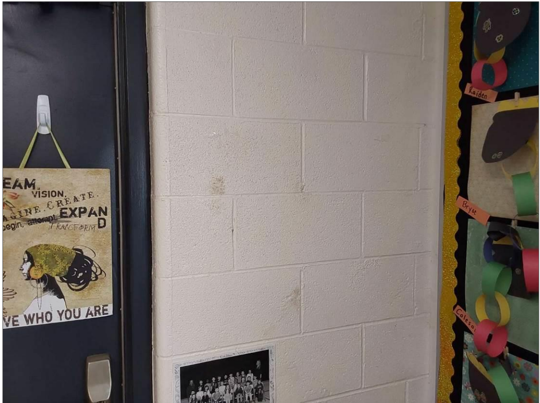
L0011(Lead, Low), White paint on concrete block wall, Wall, Kindergarten (Location #: 52)
