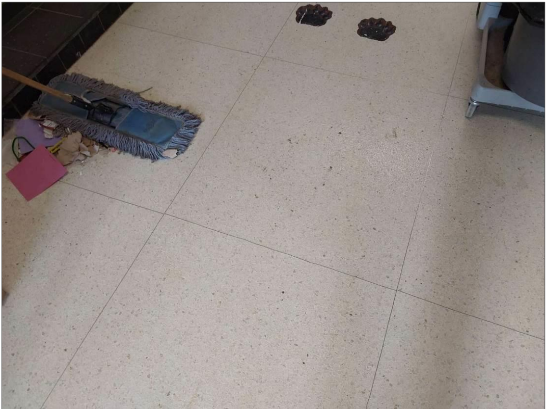
S0041A (None), Floor, Terrazzo, Corridor (Location #: 48)
