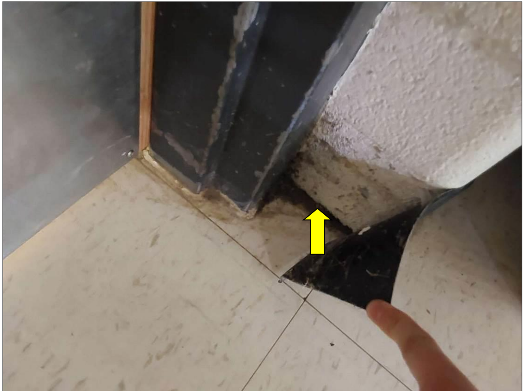
S0028 (None), Beige baseboard mastic, Other, Base, Adhesive/mastic, Kindergarten (Location #: 53)
