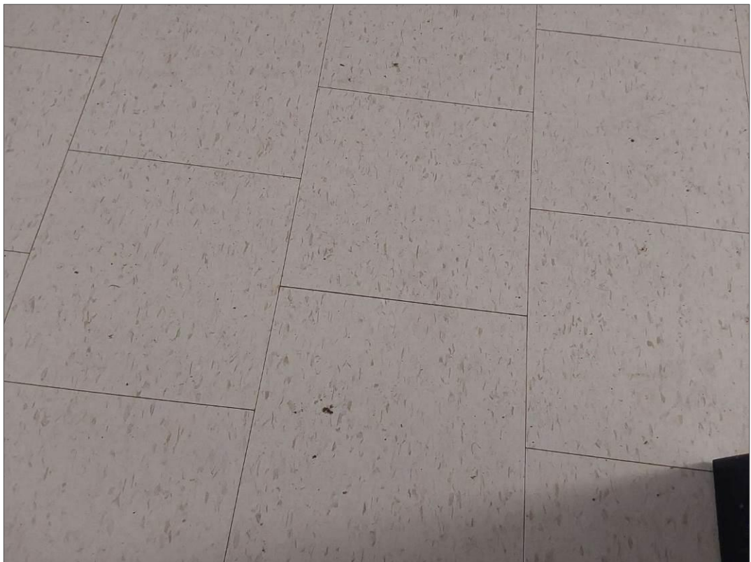
S0079C (None), 12" x 12" Off-white with brown specks, Floor, Vinyl Floor Tile and Mastic, Kindergarten (Location #: 52)
