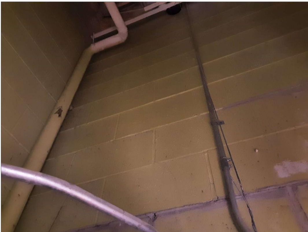
L0014(Lead, High), Light green, Wall, Storage (Location #: 19) Above ceiling
