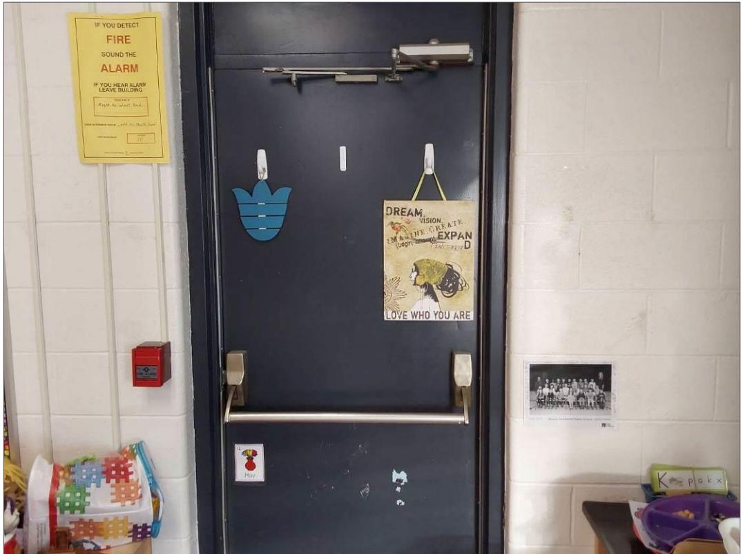
V0003(Lead, None), Dark blue on door, Other, Kindergarten (Location #: 52)
