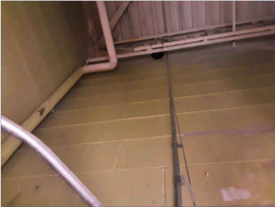
S0086C (Confirmed Asbestos), Light green, Wall, Paint, Storage (Location #: 19) Above ceiling
