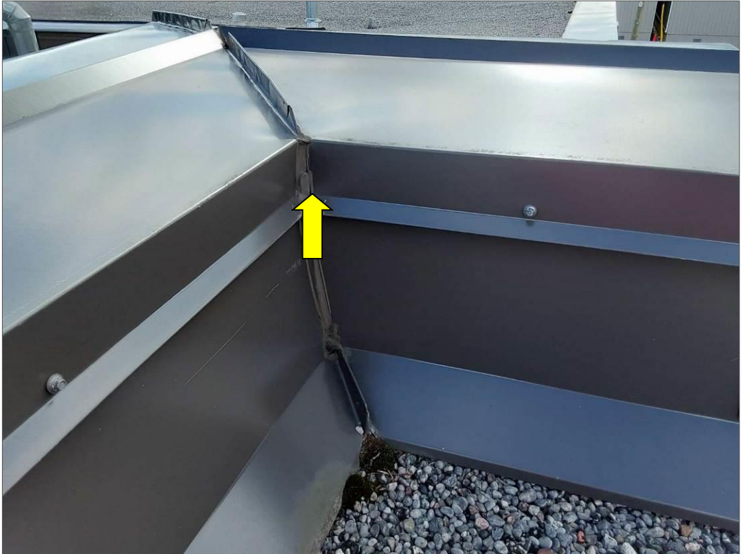
S0076A (None), Grey caulking on flashing, Other, Caulking, Roof G (Location #: 87)
